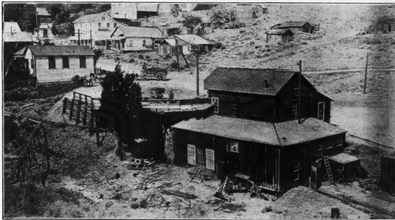
AN OLD CUSTOM MILL AT SILVER CITY, NEVADA
