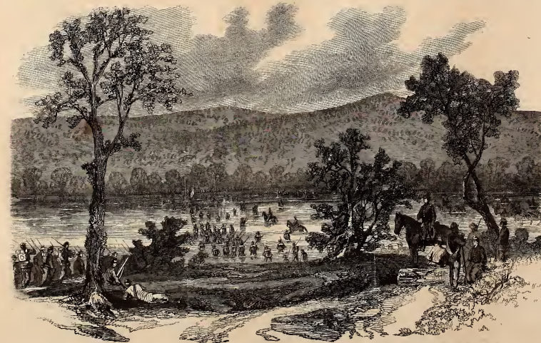
THE WAR IN GEORGIA—THE 16TH ARMY CORPS FORDING THE CHATTAHOOCHEE AT BOWWELL'S FERRY, JULY 10.—FROM A SKETCH BY GEN. D. B. PATLICK, 2ND IOWA INFANTRY.
