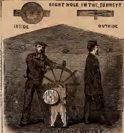
PORT HOLE AND MUZZLE OF 15 IN GUN
