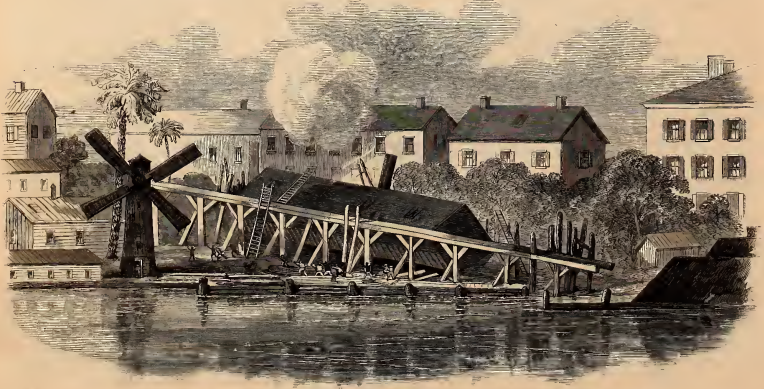
THE IRON BUILDING IN CHARLESTON HARBOR, THE REBELS' LAST WORKMEN ENGAGED IN BUILDING THE REBEL RAM.—FROM A SKETCH BY OUR SPECIAL ARTIST, W. T. CRANE.
