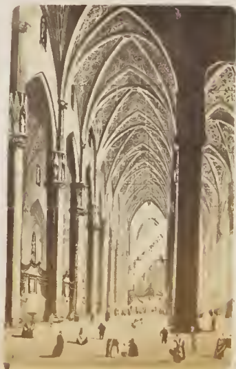
Interior of Duomo
