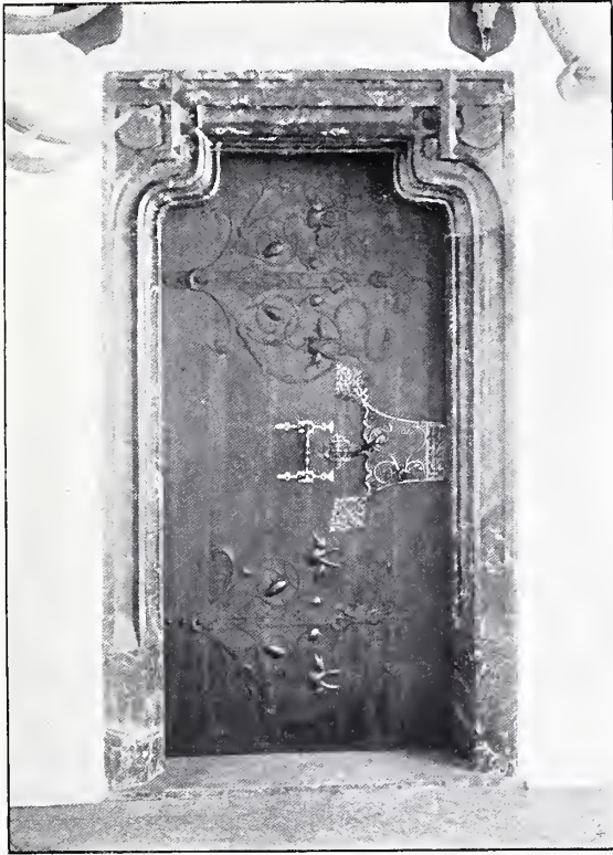
FIG. 4.—MARBLE DOORWAY AND GOTHIC IRONWORK IN SCHLOSS MATZEN, TYROL.
