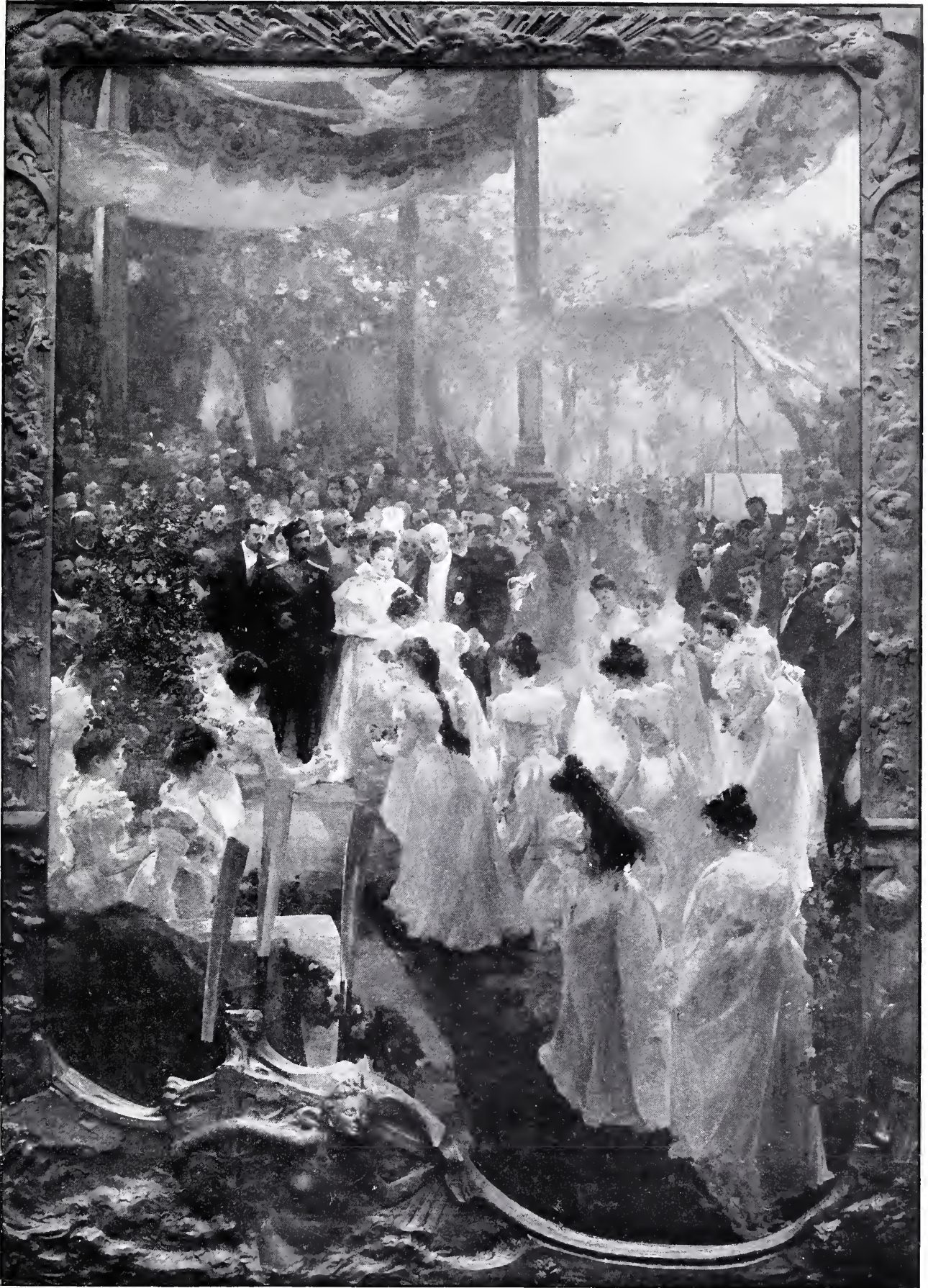
REMINISCENCE OF THE LAYING OF THE FIRST STONE OF THE ALEXANDER III BRIDGE.
