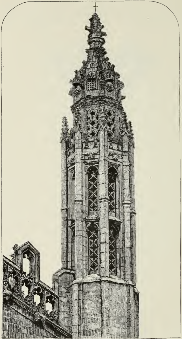
Fig. 49. Tower at the south-east angle of King's College Chapel.
