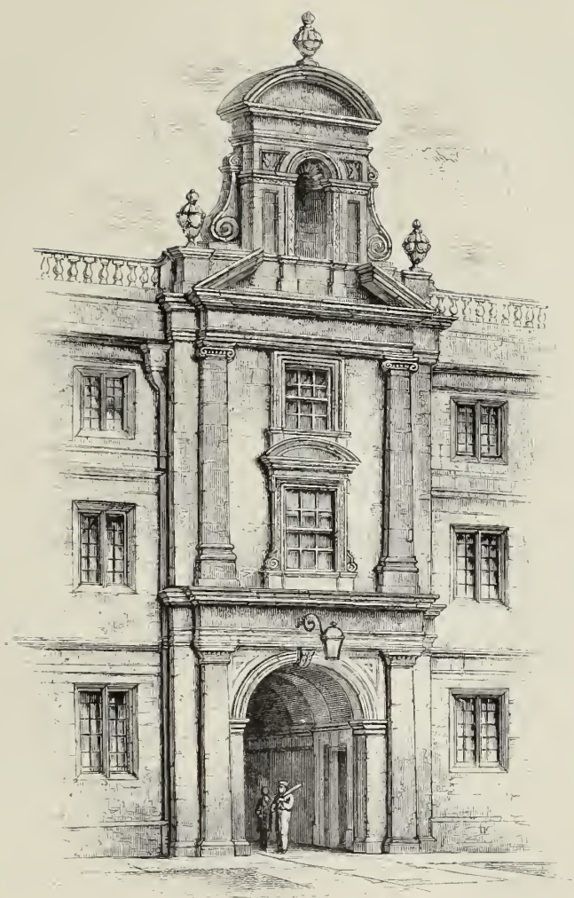
Fig. 12. East front of the gate-way in the west range of Clare Hall, designed and built by Robert Grumbold, 1765-7.
