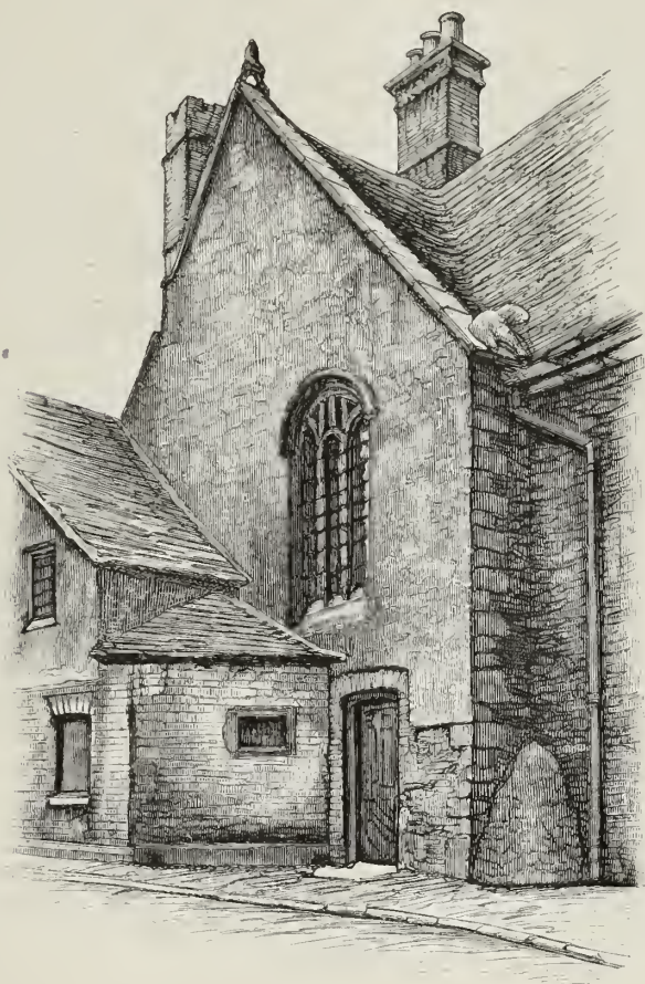
Fig. 8. East gable of the old Lodge from Free School Lane, now the entrance to the Kitchen.
