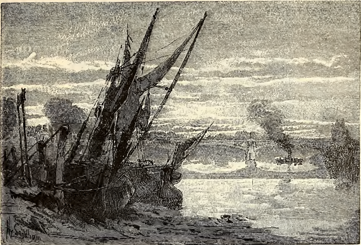
BARNES RAILROAD BRIDGE.
