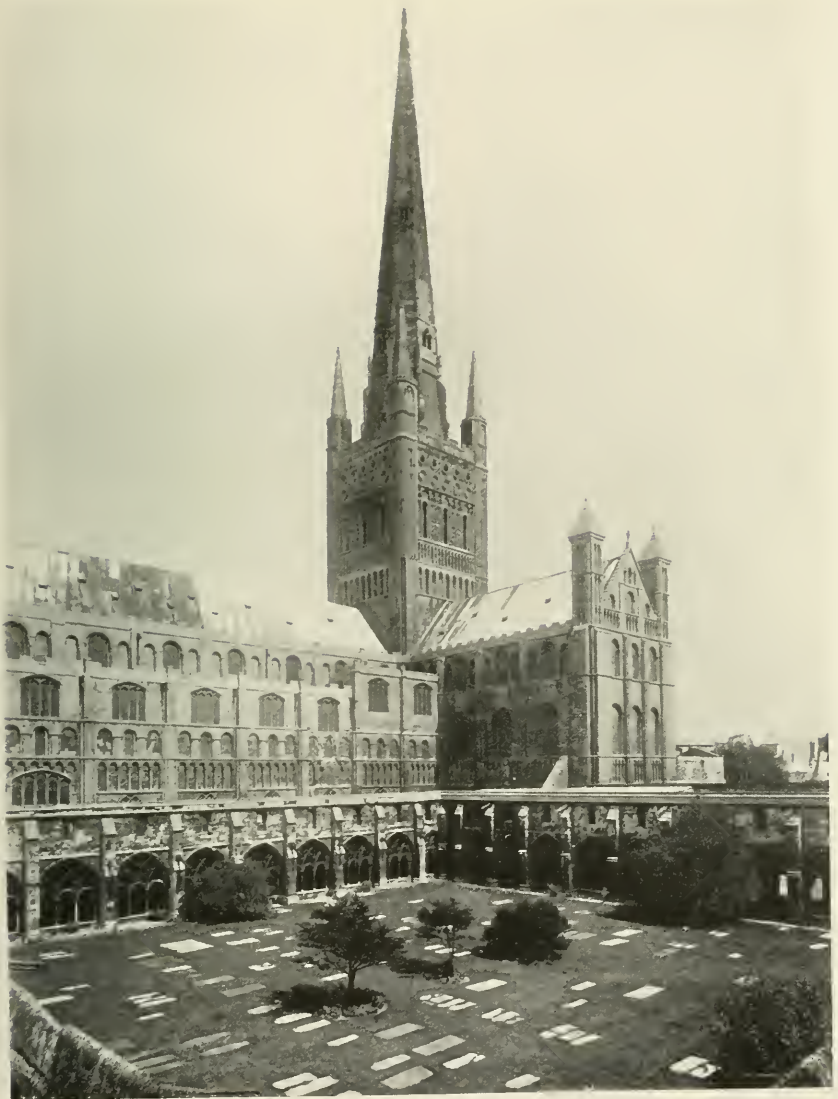
NORWICH CATHEDRAL, FROM THE SOUTH-WEST.
