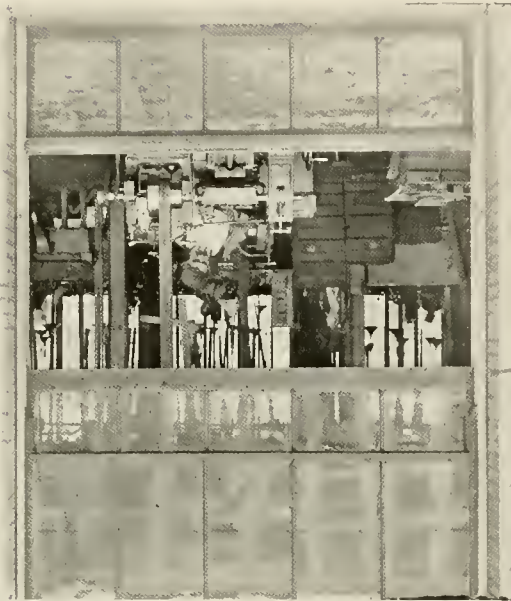
One of the factory windows. Four-fifths of the wall space is glass.
