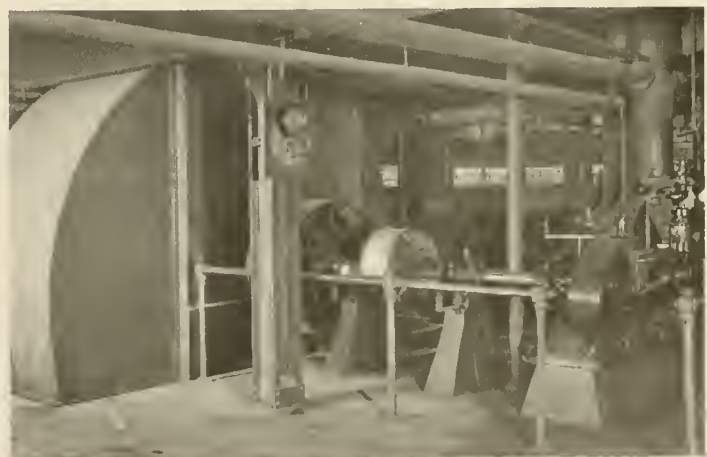
Ventilating apparatus which changes air in buildings every fifteen minutes.
