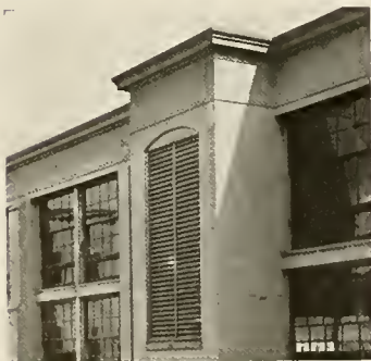
Air is drawn in through ventilators at the top of the building where the air is purest
