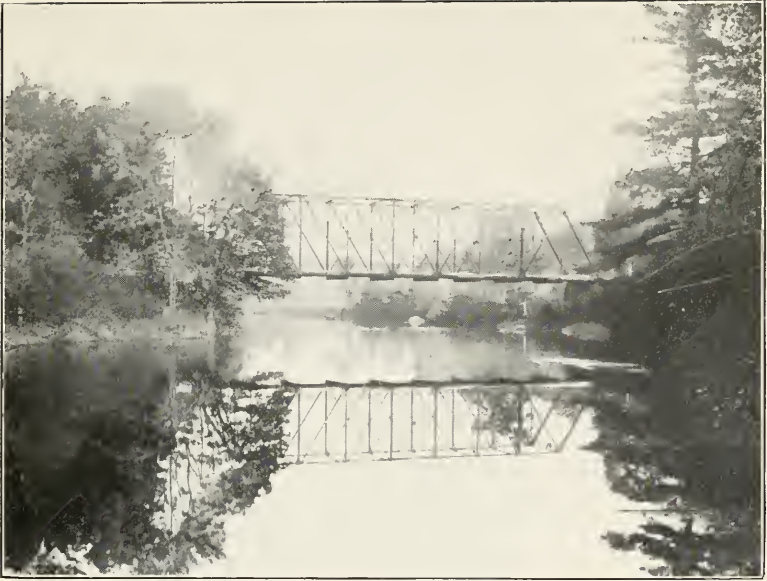
STEEL BRIDGE, HENNIKER ROAD.
