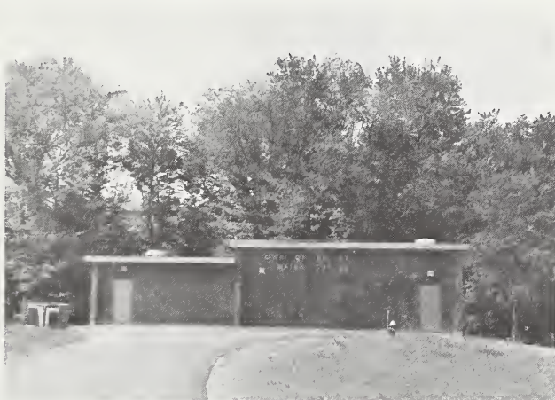
Callahan Well - A newly developed municipal ground water supply in Hadley.
