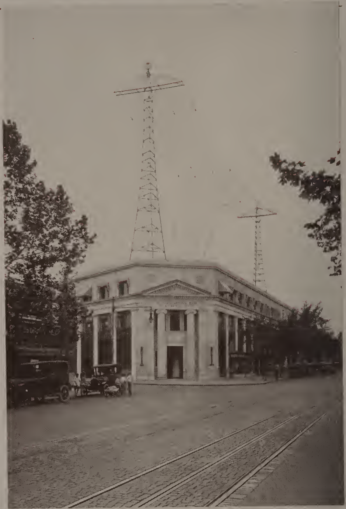
BROADCASTING ANTENNA OF RCA STATION "WRC" Atop the Riggs National Bank Building at Washington, D. C.
