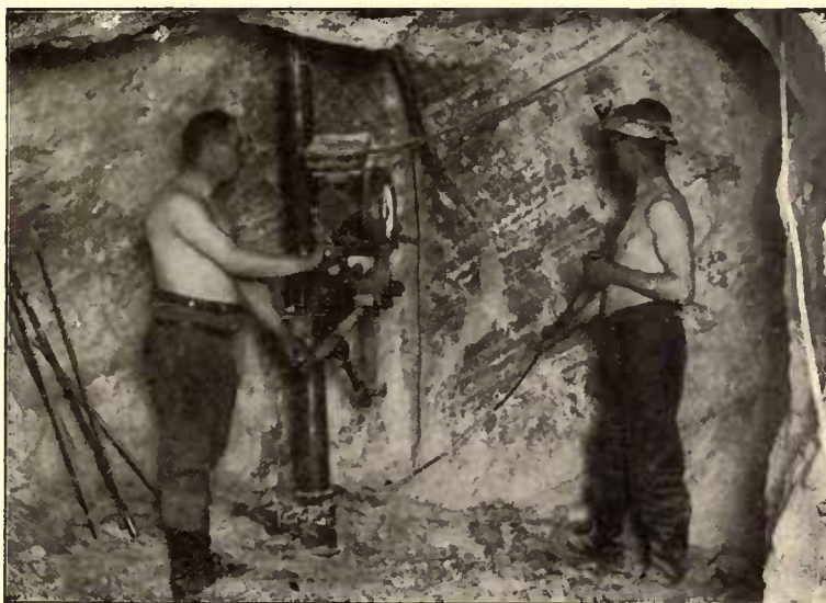
Fig. 155 Percussion Drill working as Cutter. Making a vertical cut.
