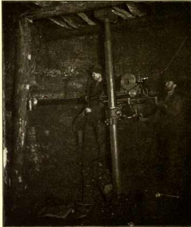
Fig. 156 Percussion Drill working as Cutter. Making a horizontal cut.
