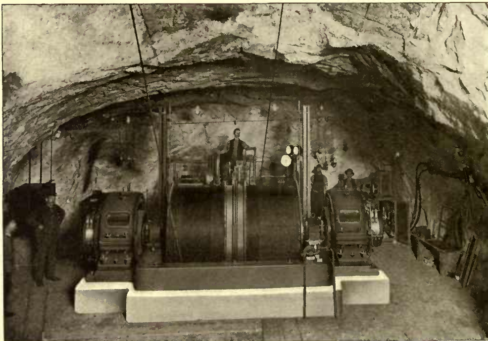
Fig. 61. Electric Winder at Thiede, near Brunswick, Germany.
