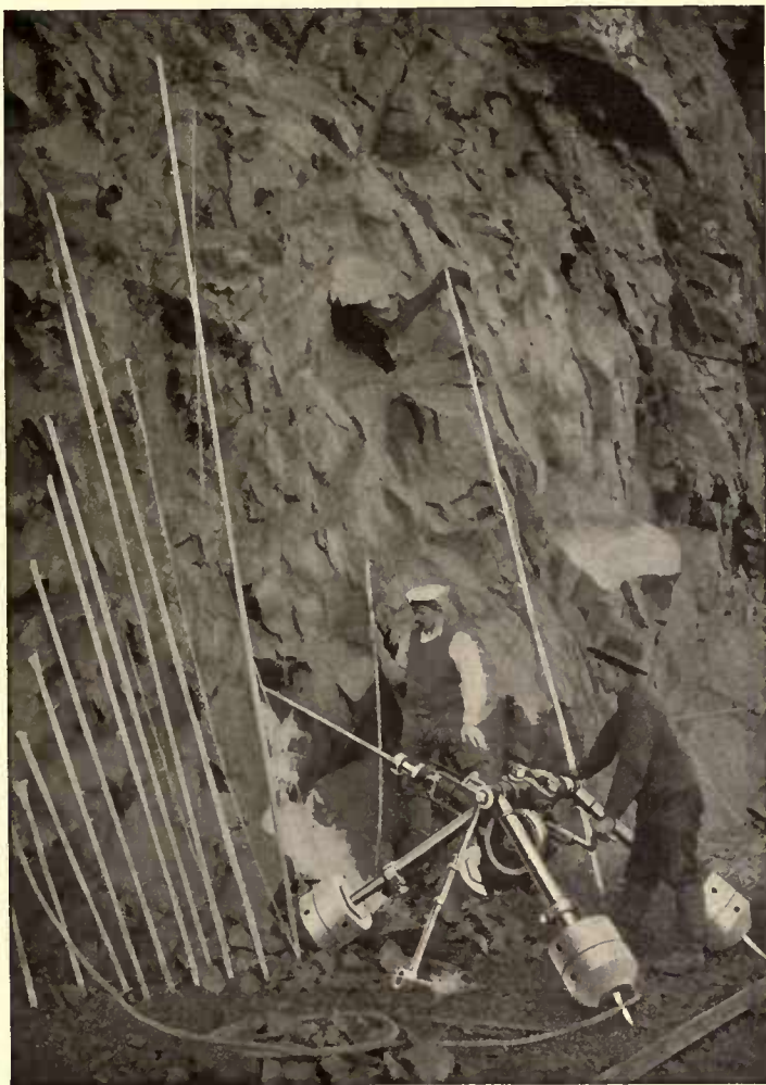
Fig. 154 Percussion Drill Mounted on tripod.
