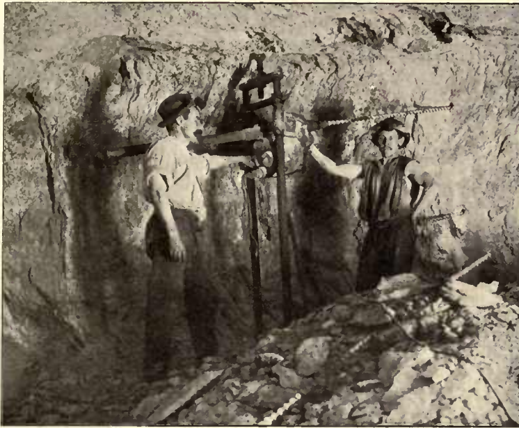
Fig. 159 Rotary Drill in a Potash Mine.
