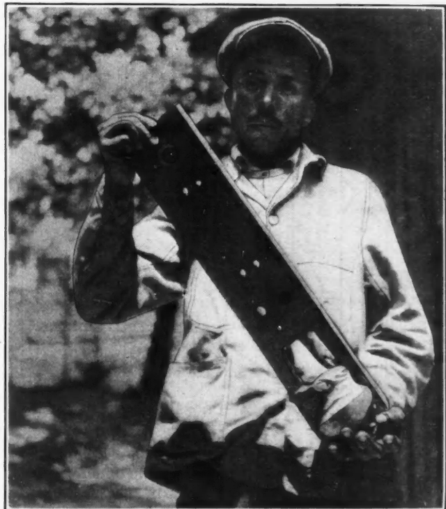
ROPE DRILL BIT RECOVERED BY SPECIAL RIG
