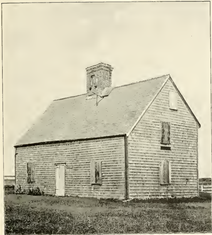
OLD HOUSE, BUILT 1686.
