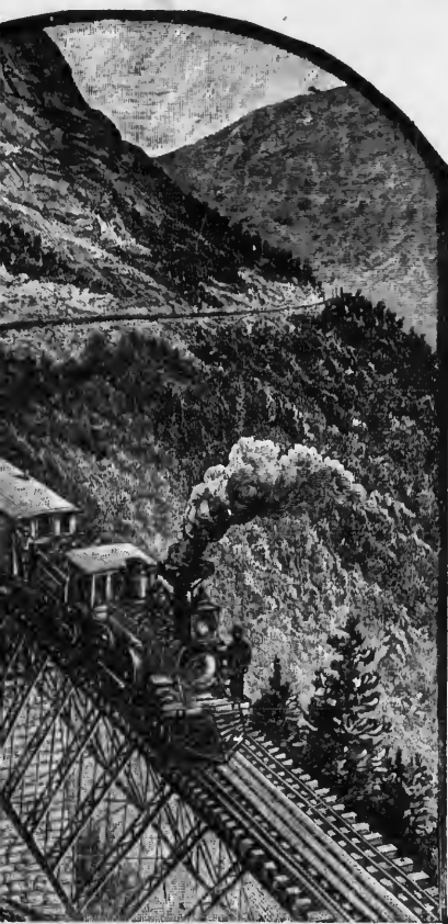
BRIDGE CROSSING MOUNT WASHINGTON.
