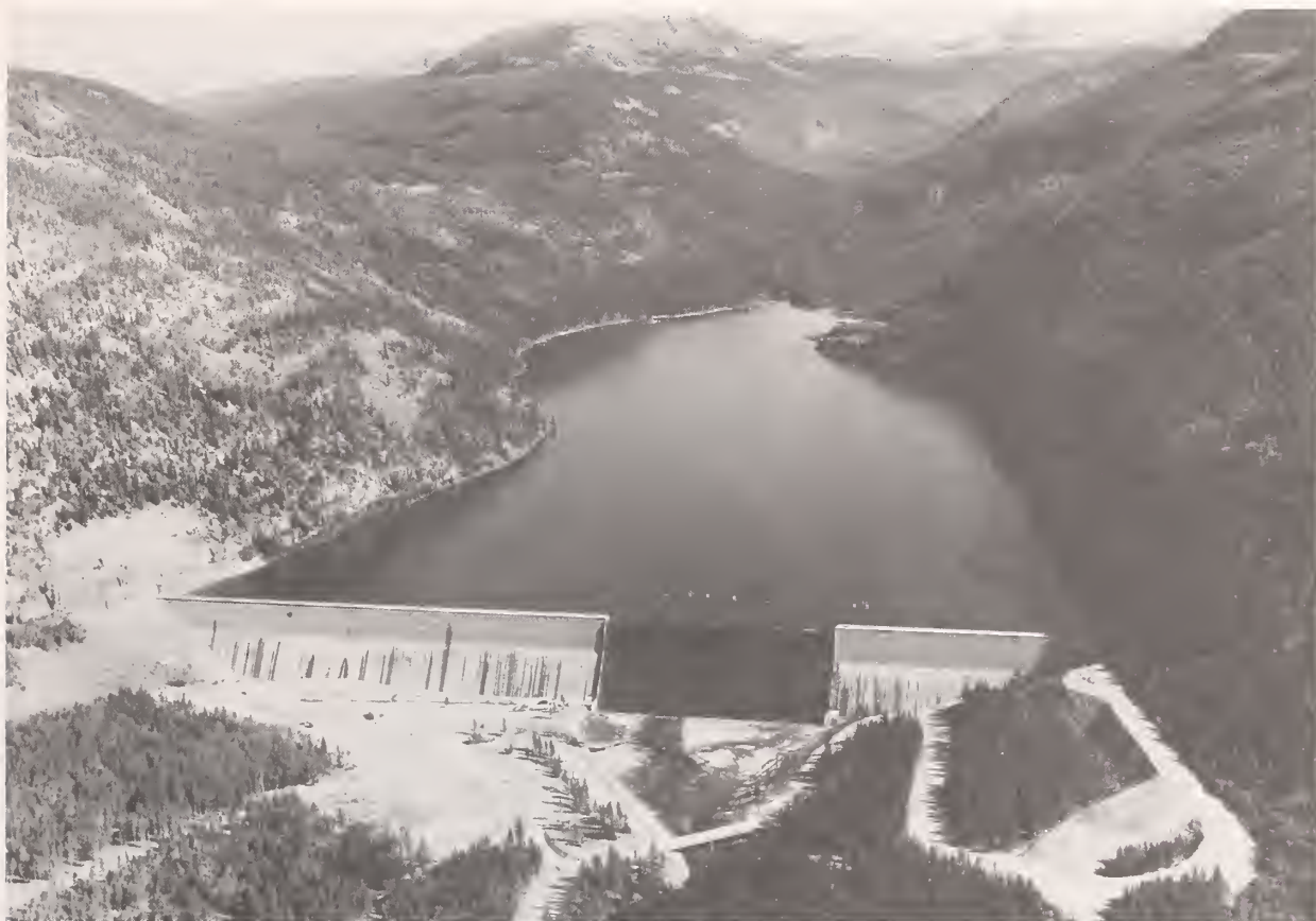
Aerial view of Upper Stillwater which is the world's largest roller-compacted concrete dam. It is part of the Central Utah Project (Bonneville Unit) and is 120 miles southeast of Salt Lake City on Rock Creek (near Duchesne, Utah). (Photo credit: Gayla Heaton, Bureau of Reclamation.)
