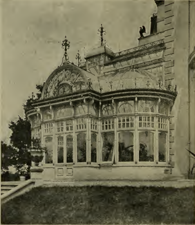
ERECTED AT ORPINGTON, KENT.
