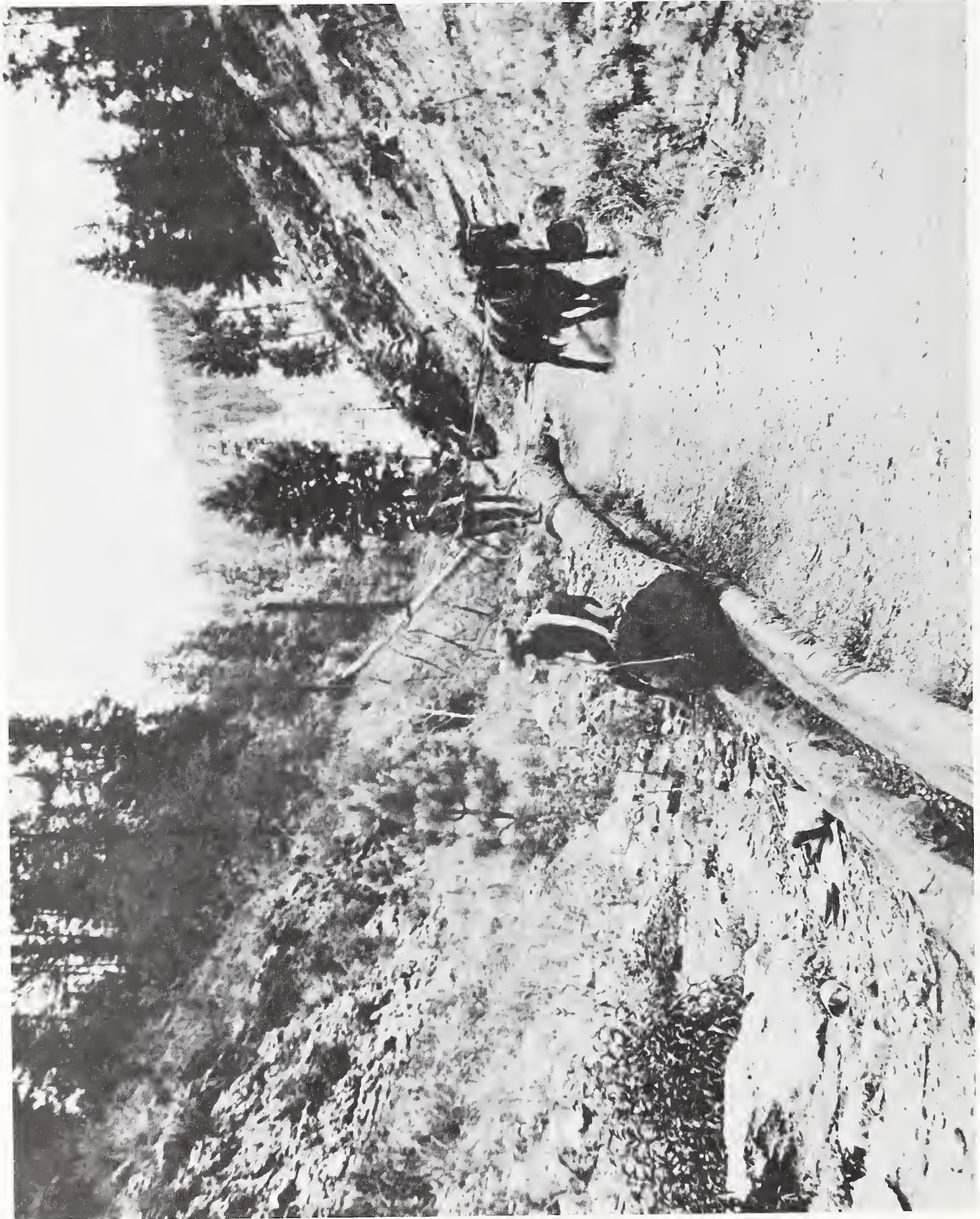
Figure 52. Log chute or skidway in action, with boy "greasing the skids." June 26, 1928. By E. S. Shipp. USDA Forest Service photo 233058.
