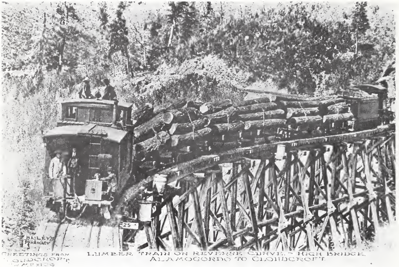
Figure 38. Log train on the "S" trestle below Cloudcroft, ca. 1910, showing the complex mechanical detail of steam reilroading. A layer of grevel is used to protect the ties end stringers from sperks. By Bailey Pharmacy.
