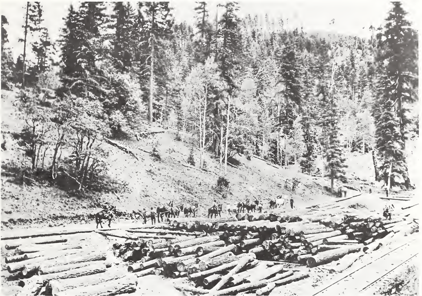
Figure 19. Logging crew with horses going into the woods from Water Canyon. The skidway disappearing up the side valley and the neatly stacked "cold decks" of logs are typical of the railroed reloaded points. June 28, 1928. By E. S. Shipp. USDA Forest Service photo 233051.
