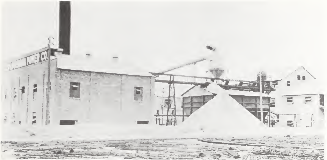
Figure 29. Georgia E. Breece Lumber Co. sawmill (right) and Texas-Louisiana Power Company steam power plant. The mill waste fed the steam boilers of the power plant, which in turn powered the sawmill as well as an electric light plant for the towns of Alamogordo and Le Luz. June 30, 1928. By E. S. Shipp. USDA Forest Service photo 233358.
