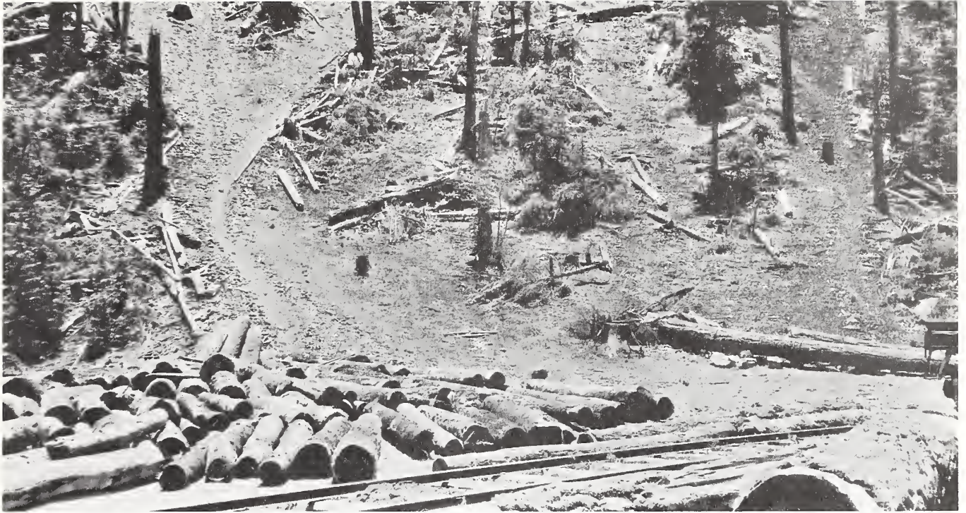
Figure 53. Log skidway along Southwest Lumber Co. railroad in Hubbell Canyon. June 27, 1928. By E. S. Shipp. USDA Forest Service photo 233034.
