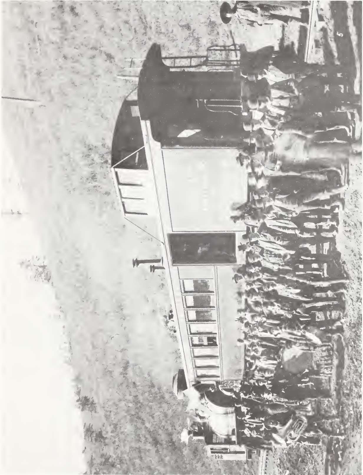
Figure 45. Dedication Day of the A&SM, celebrated at Toboggan on November 16, 1898. The elegant car combined the functions of passenger coach, baggage-mail-express car, and caboose in one vehicle, a necessity on the steeply graded railroad. By Bushong & Feldman. Museum of New Mexico photo 14914.
