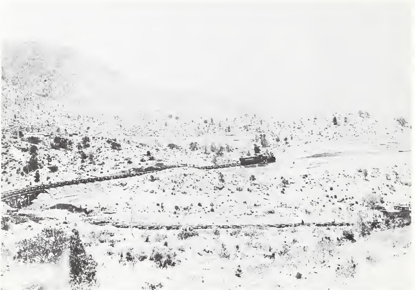
Figure 40. In early 1902, the brand new Shay patent geared locomotive, number 105, pulled a 334-ton train of 41 empty log cars from Alamogordo to Toboggan. The train was stopped for the photographer on the "S" curva between El Valla and Pinto. Baldwin-Lima-Hamilton Corp. collection.
