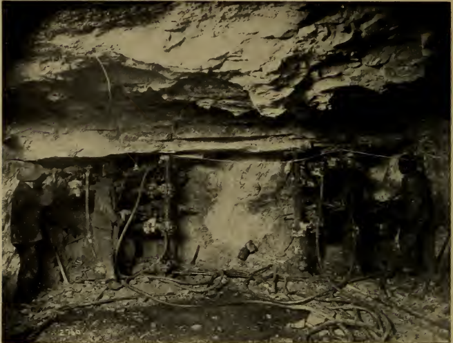
FIG. 4. Driving a modern tunnel with machine-drills.
