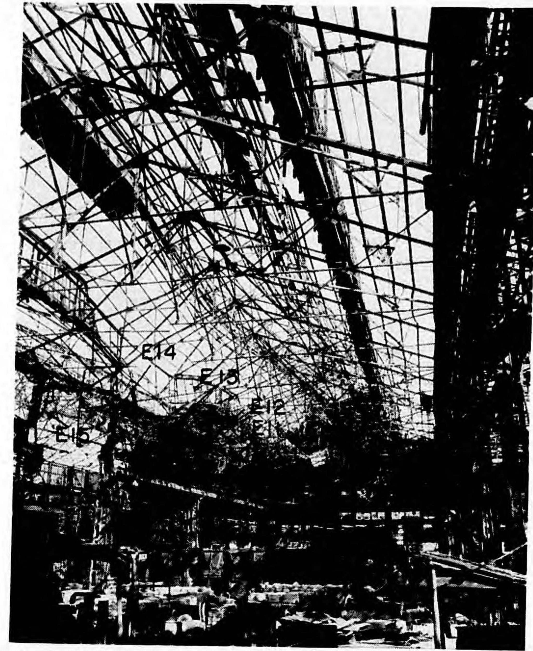
Photo 12.—Building 301b; roof damage between Columns E15 and E16 looking NE.
