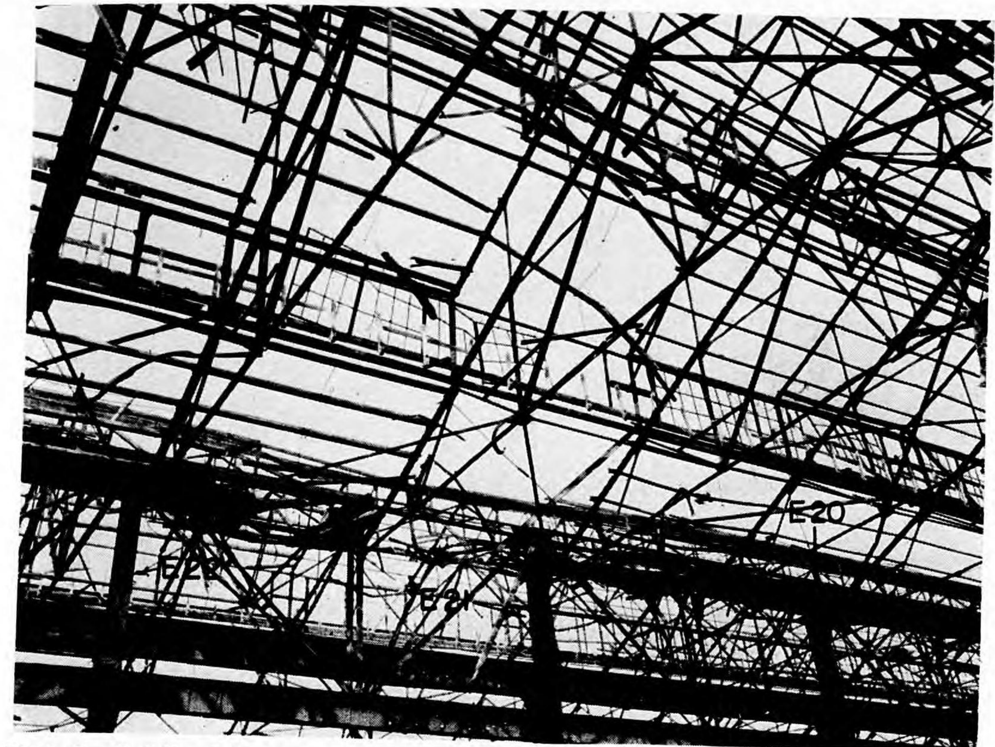
Photo 7.—Building 301b; roof damage caused by Bomb 18 adjacent to Column E21 looking N.
