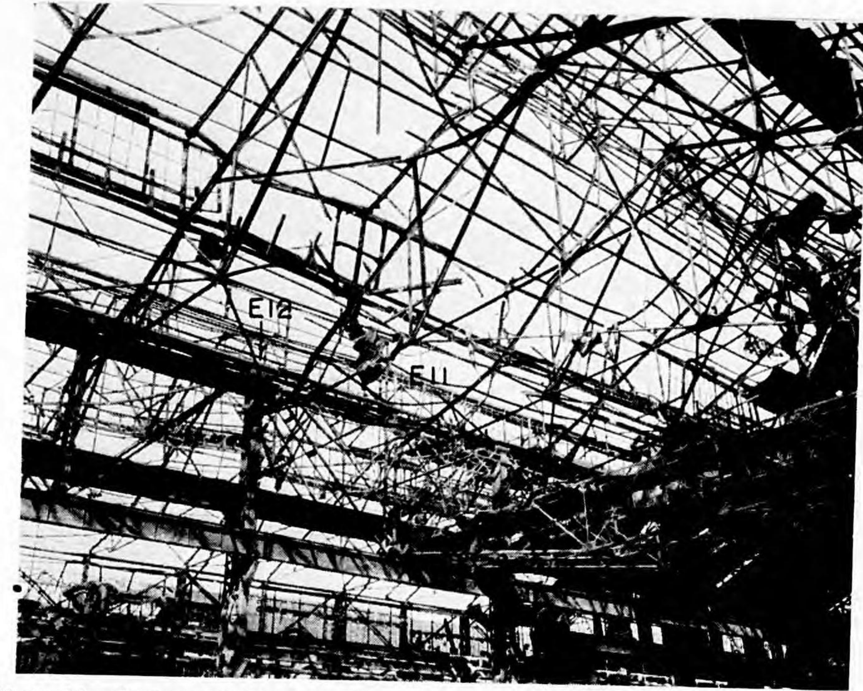
Photo 11.—Building 301b; roof damage between Columns E12 and E11 looking N.
