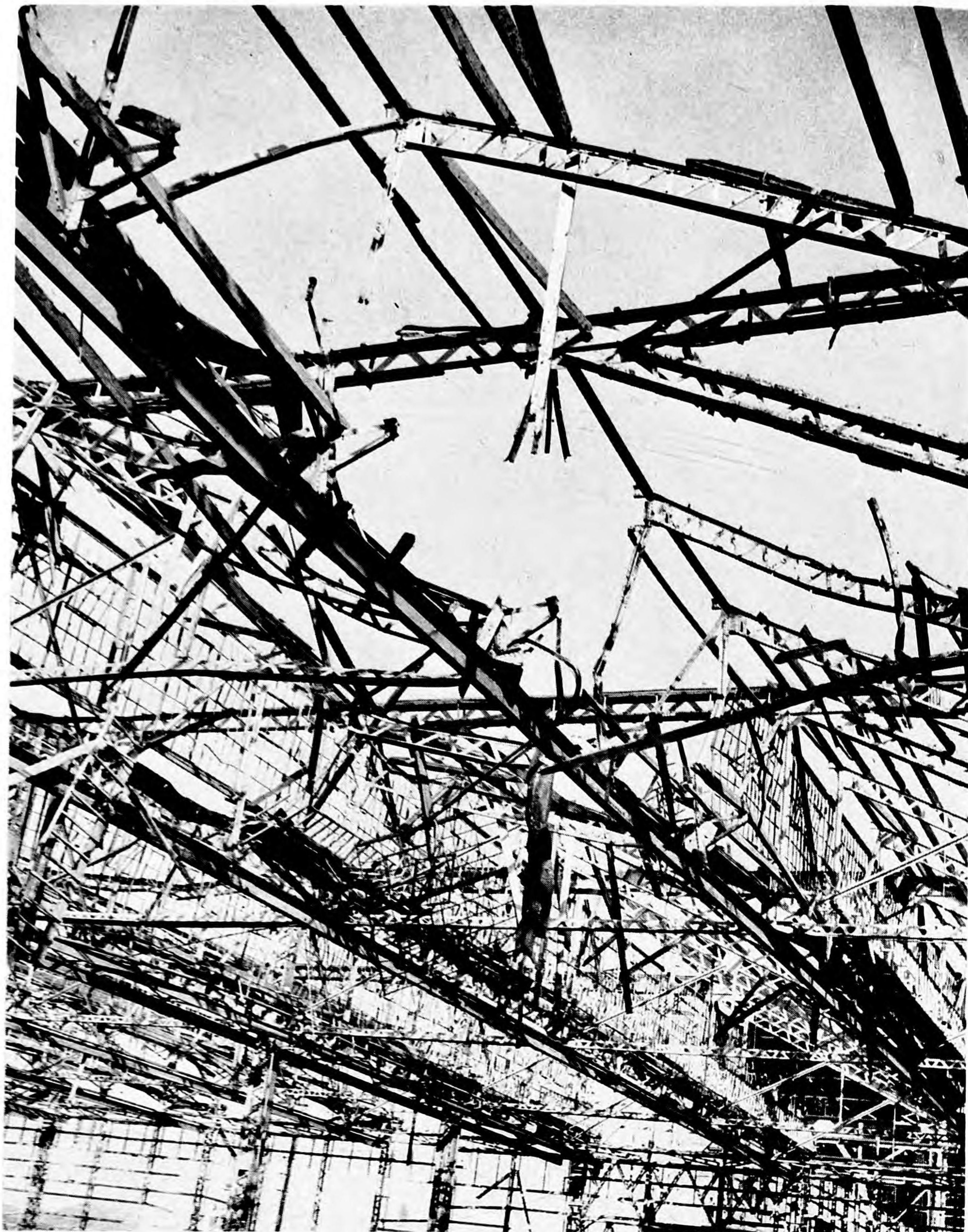
Photo 15.—Building 3, Bomb 28; roof damage; heavy members intact.
