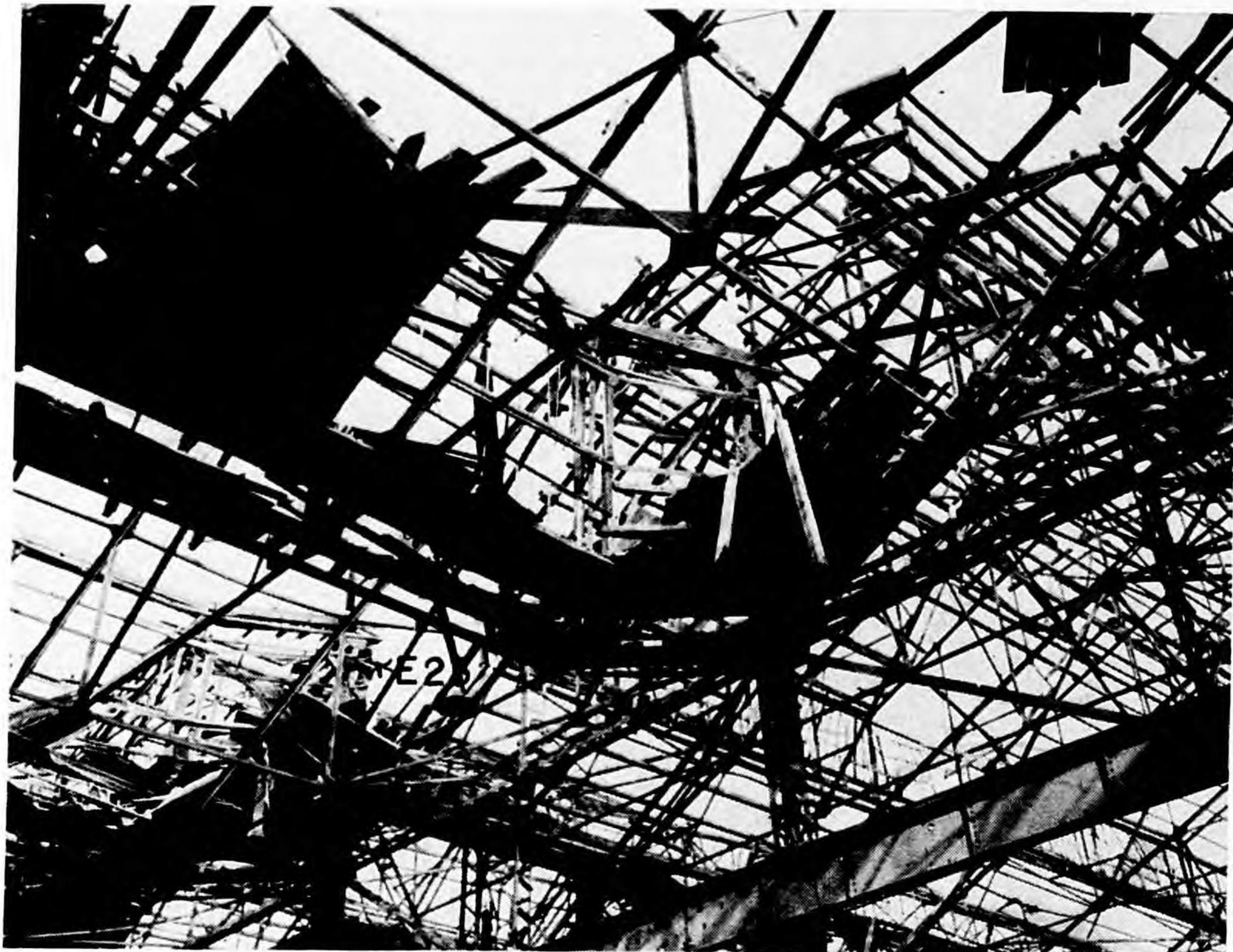
Photo 5.—Building 304; damage to truss connecting to Column E23 looking NNW.
