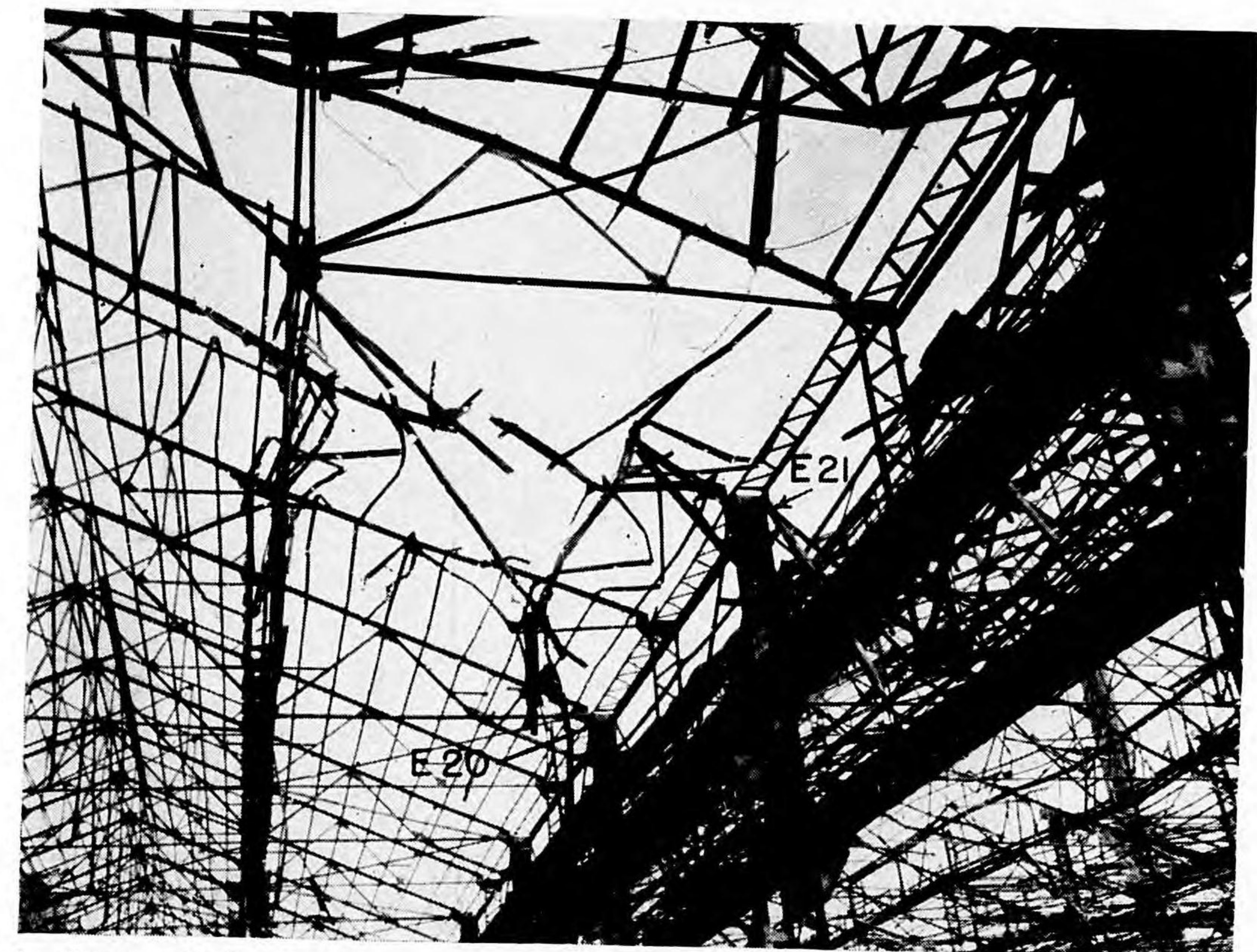
Photo 8.—Building 301b; damage caused by Bomb 19 to roof trusses adjacent to Column E21 looking NE.
