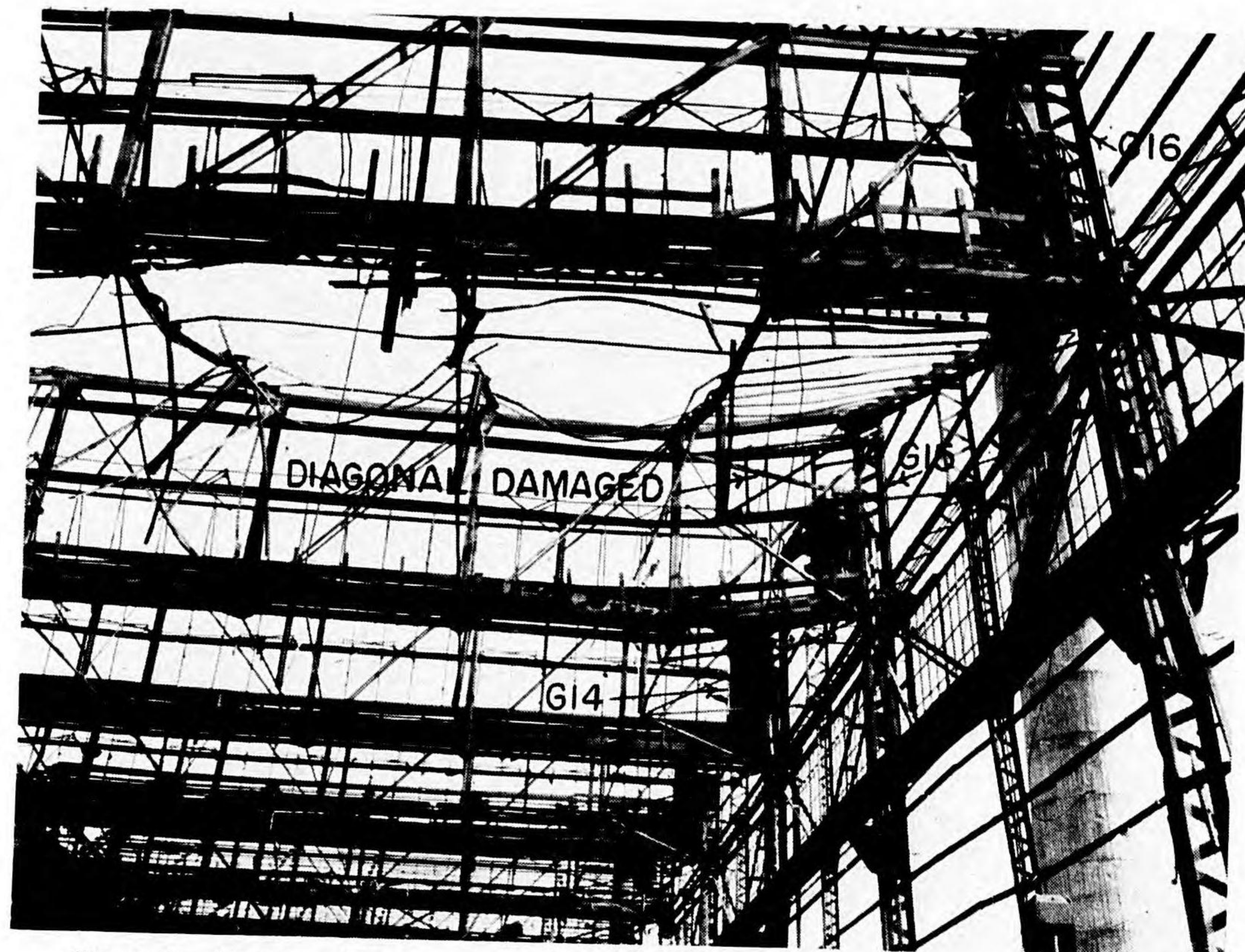
Photo 2.—Building 301a, sagging of truss connecting to Column (G15) looking NE.
