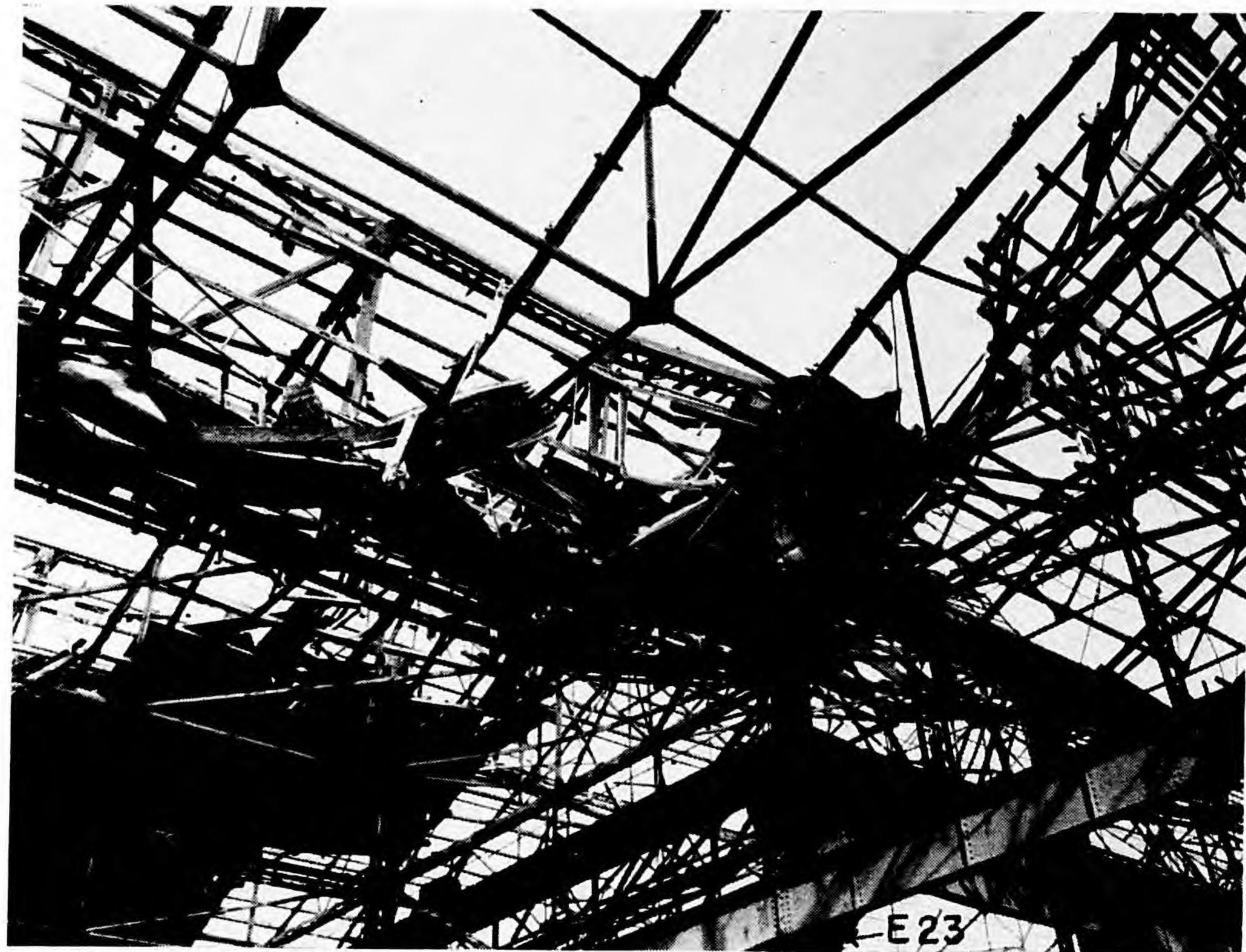
Photo 6.—Building 304; damage to truss Connecting to Column E23 looking N.
