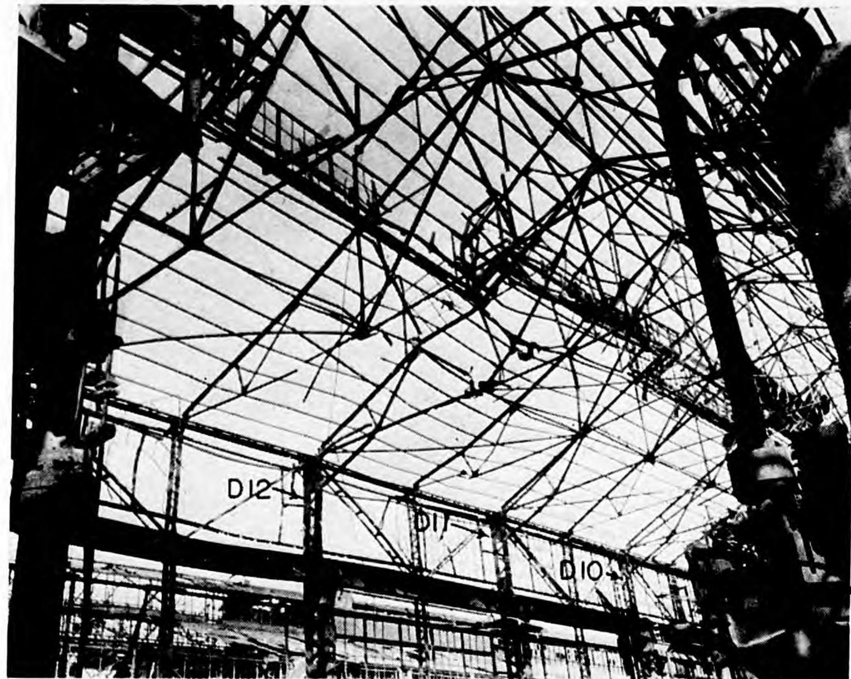
Photo 13.—Building 301b; damage to crane girder and roof members between Columns D13 and D11 looking NNW.
