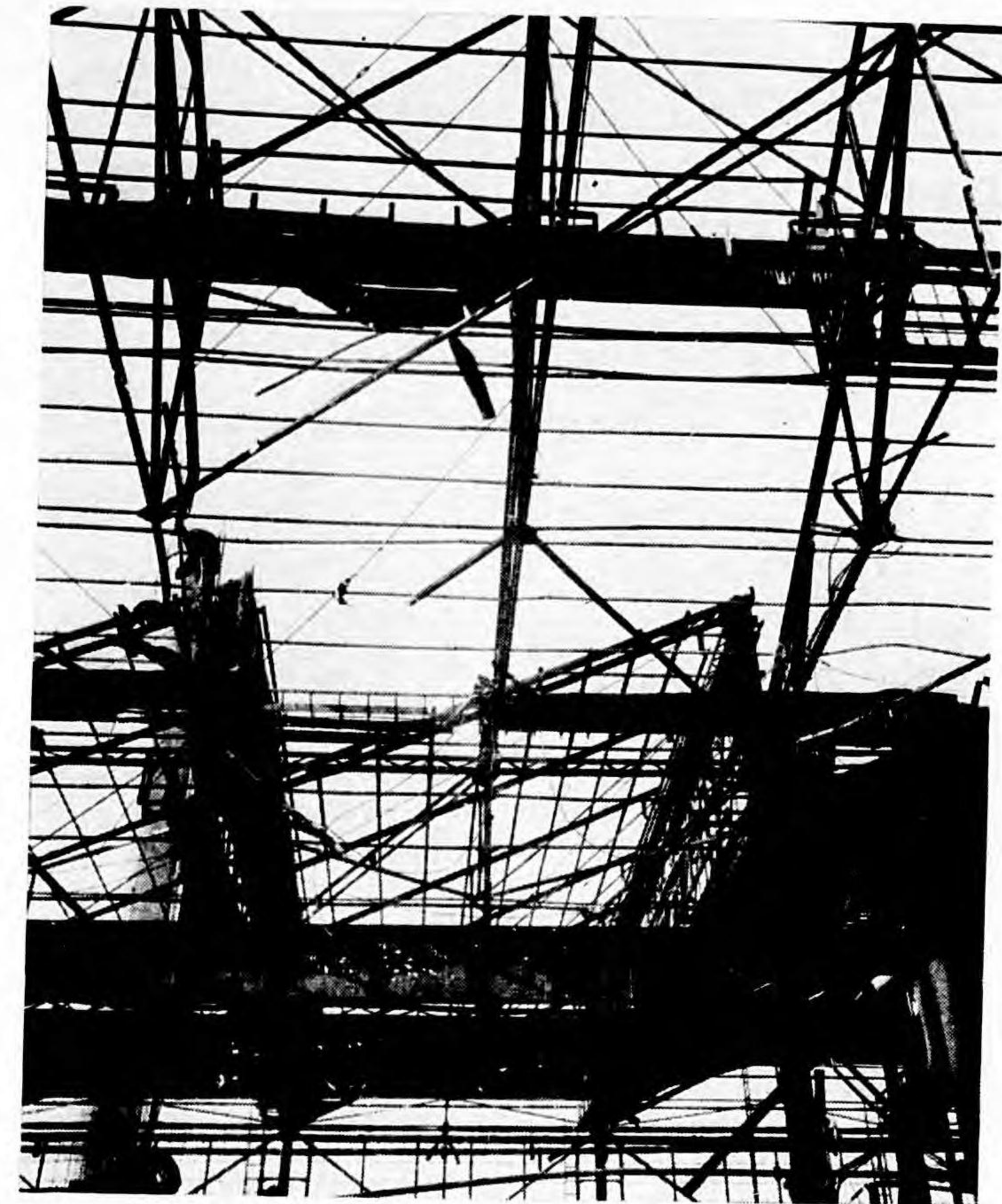
Photo 19.—Building 302a; damage to roof trusses and crane girders between Columns B13 and B12 looking NW.
