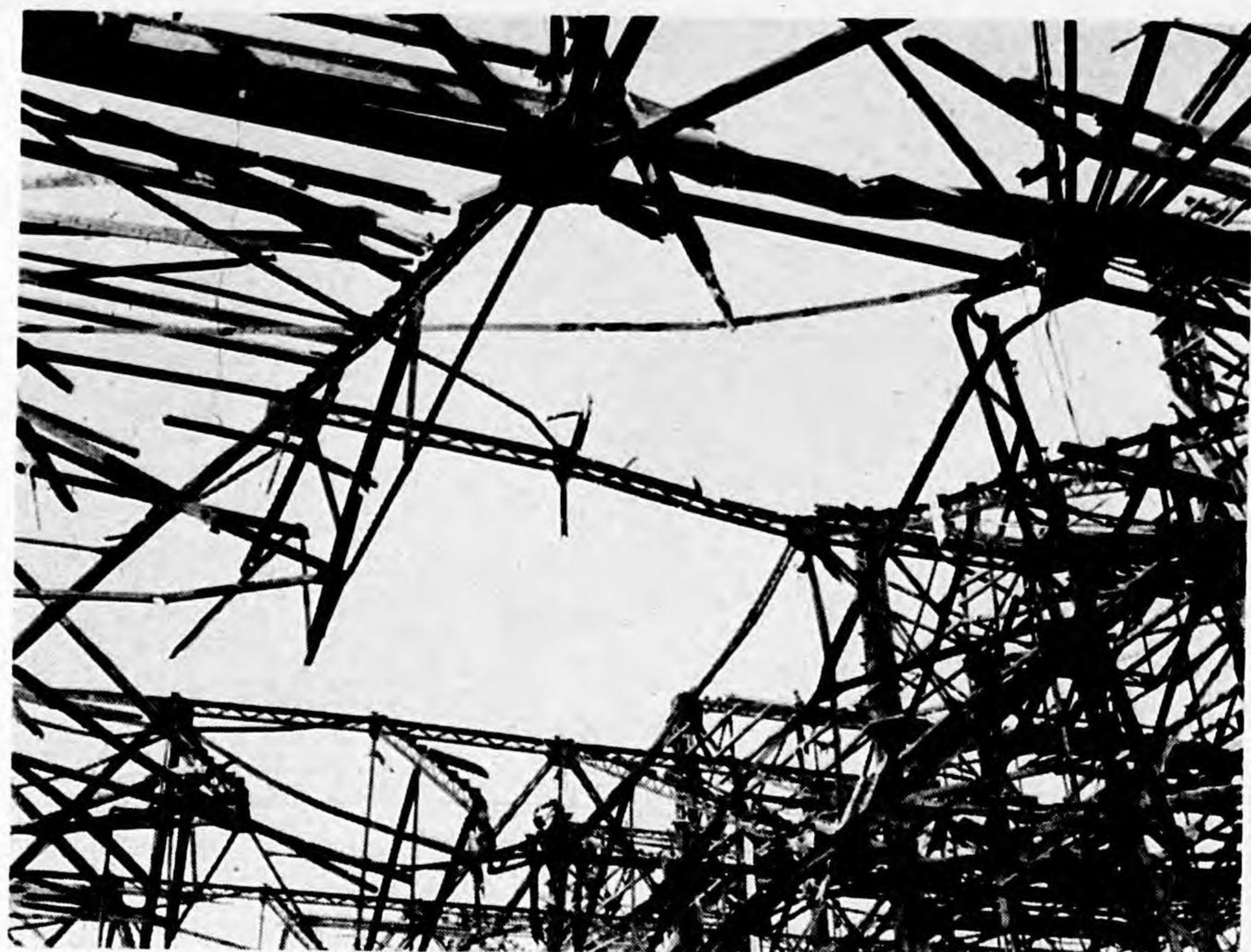
Photo 7.—Building 2, Bomb 8; damage to roof steel.
