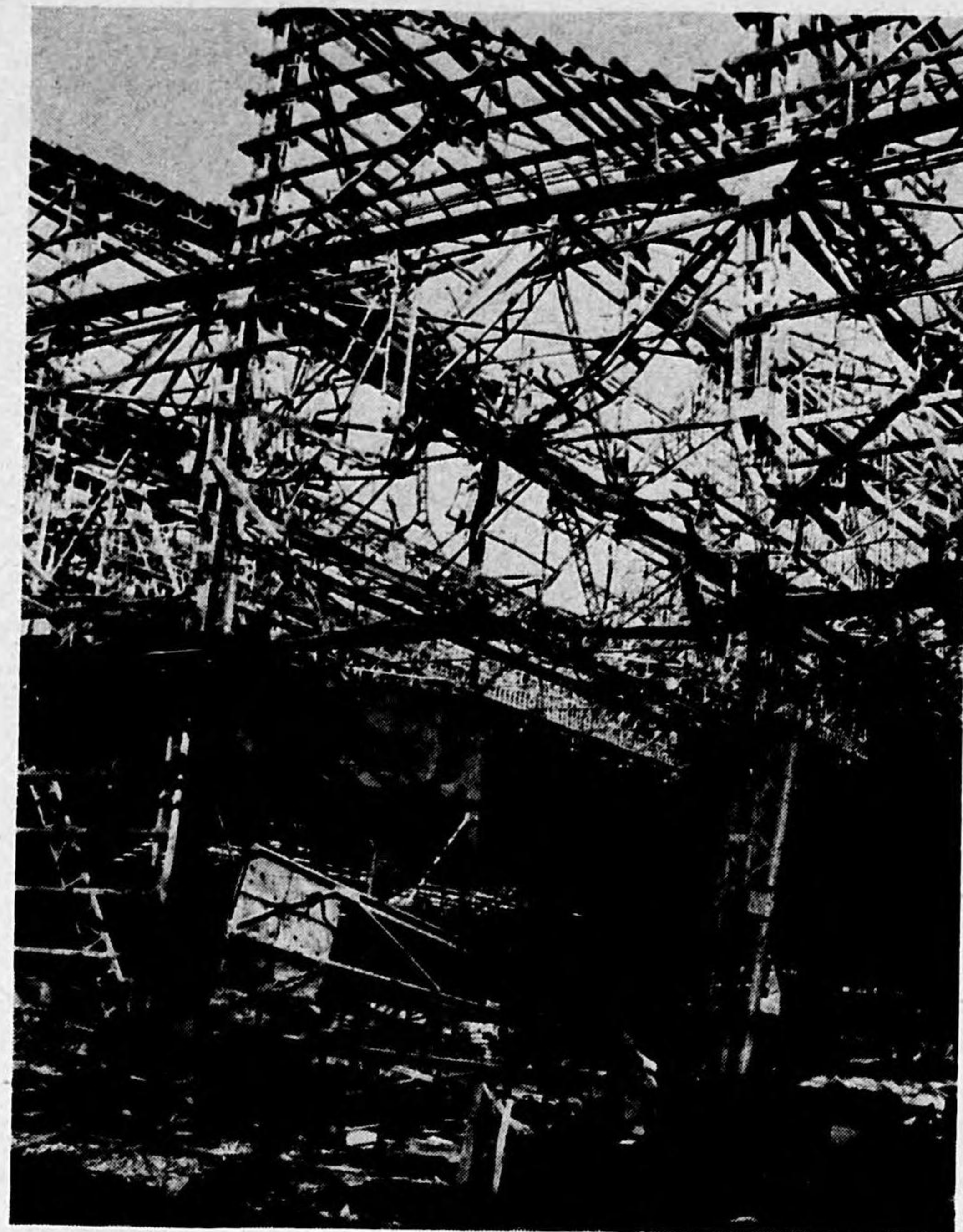
Photo 1.—Building 1, Bombs 1 and 2; damaged exterior column and roof steel.
