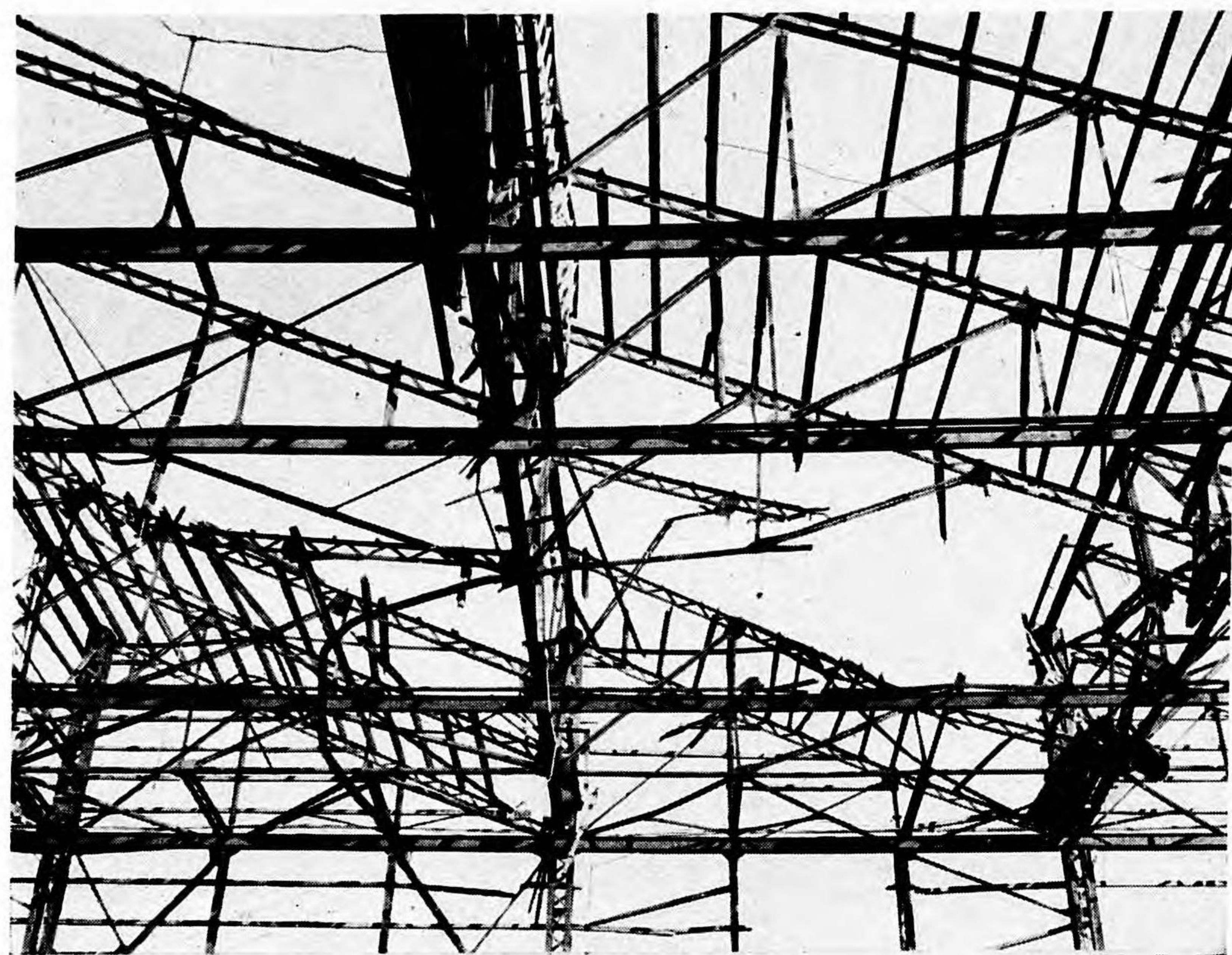
Photo 4.—Building 2, Bomb 4; damage to roof steel.
