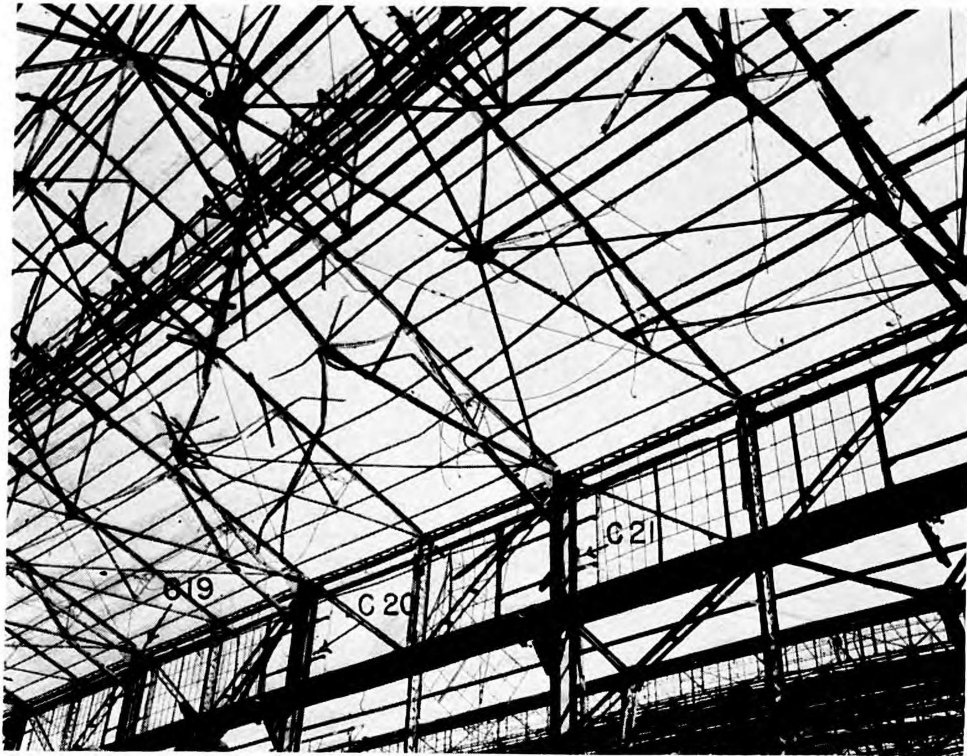
Photo 17.—Building 302a; damage to roof trusses adjacent to Columns C21 and C20 looking ENE.
