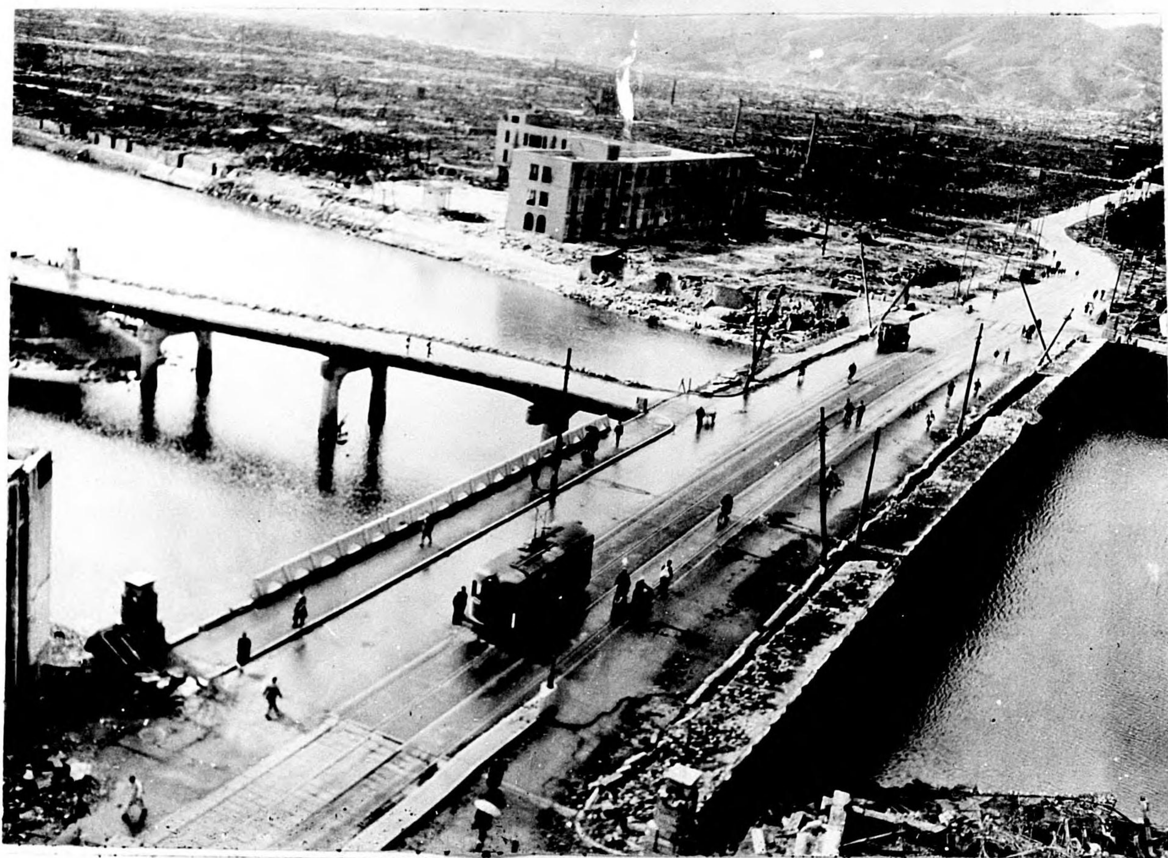
Photo 173. Hiroshima. Intersection of two bridges, approximately 930 feet from GZ. All damage caused by blast.
