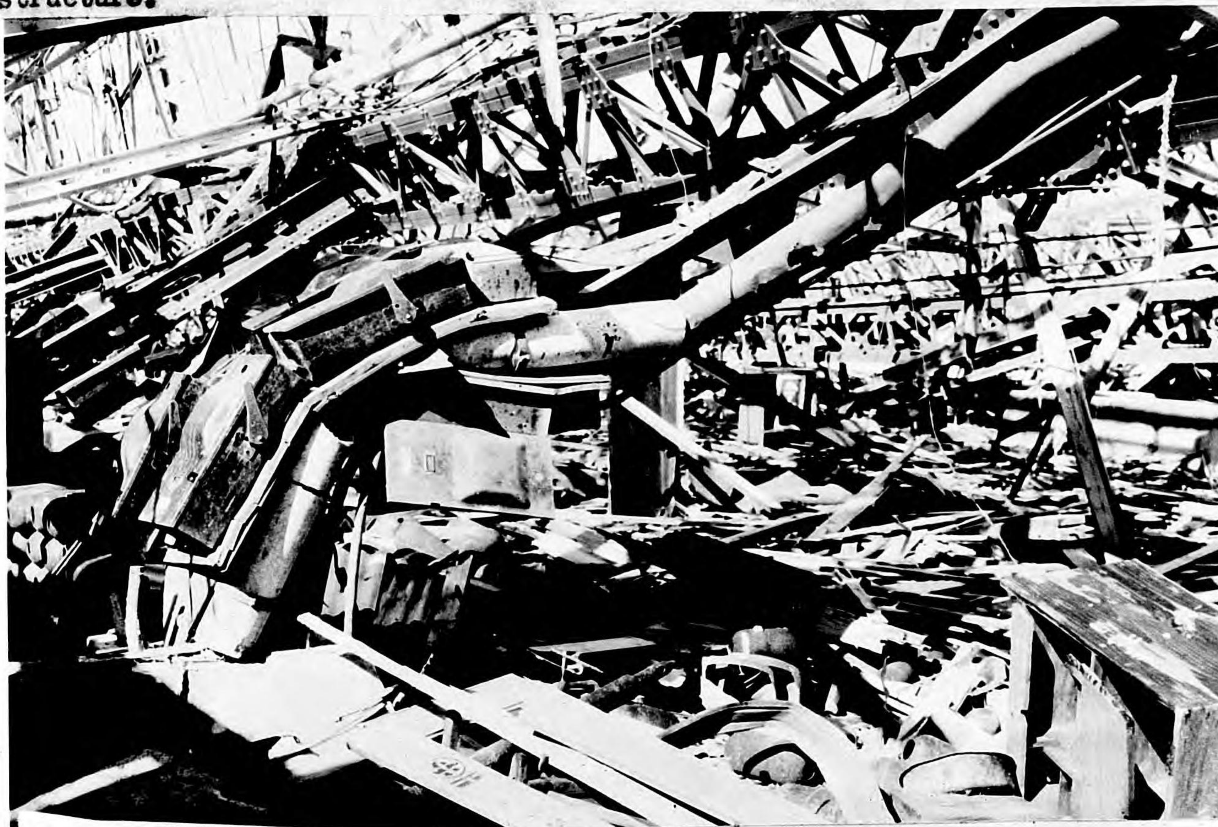
Photo 139. Nagasaki, 4,200 feet from GZ. Typical utility damage in steel- structure.
