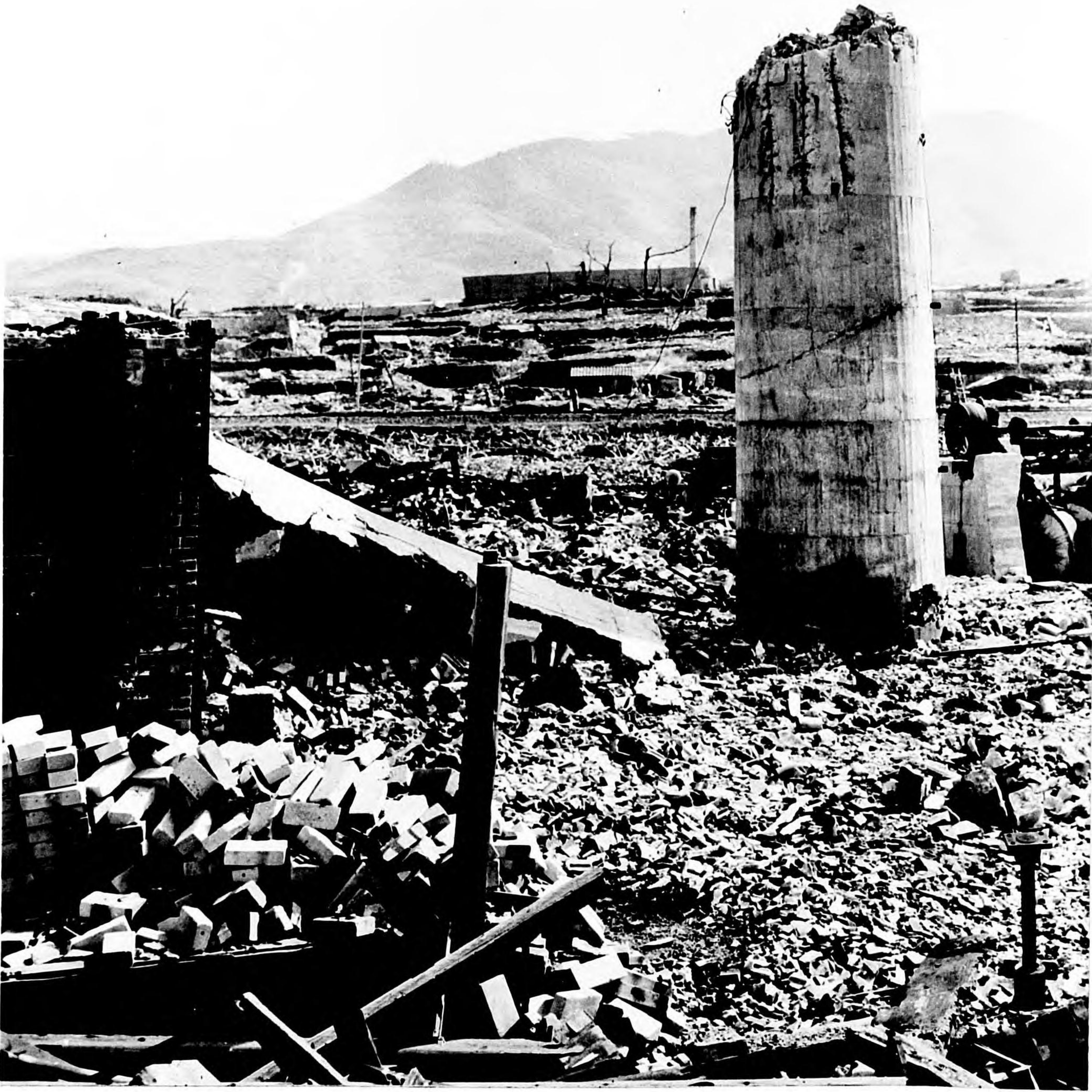
Photo 158. Nagasaki. Area west of railroad and highway in fork of Urakami River. Concrete stack, four feet in diameter and 70 feet high, fell to north-west. Brick kiln at left of photo.
