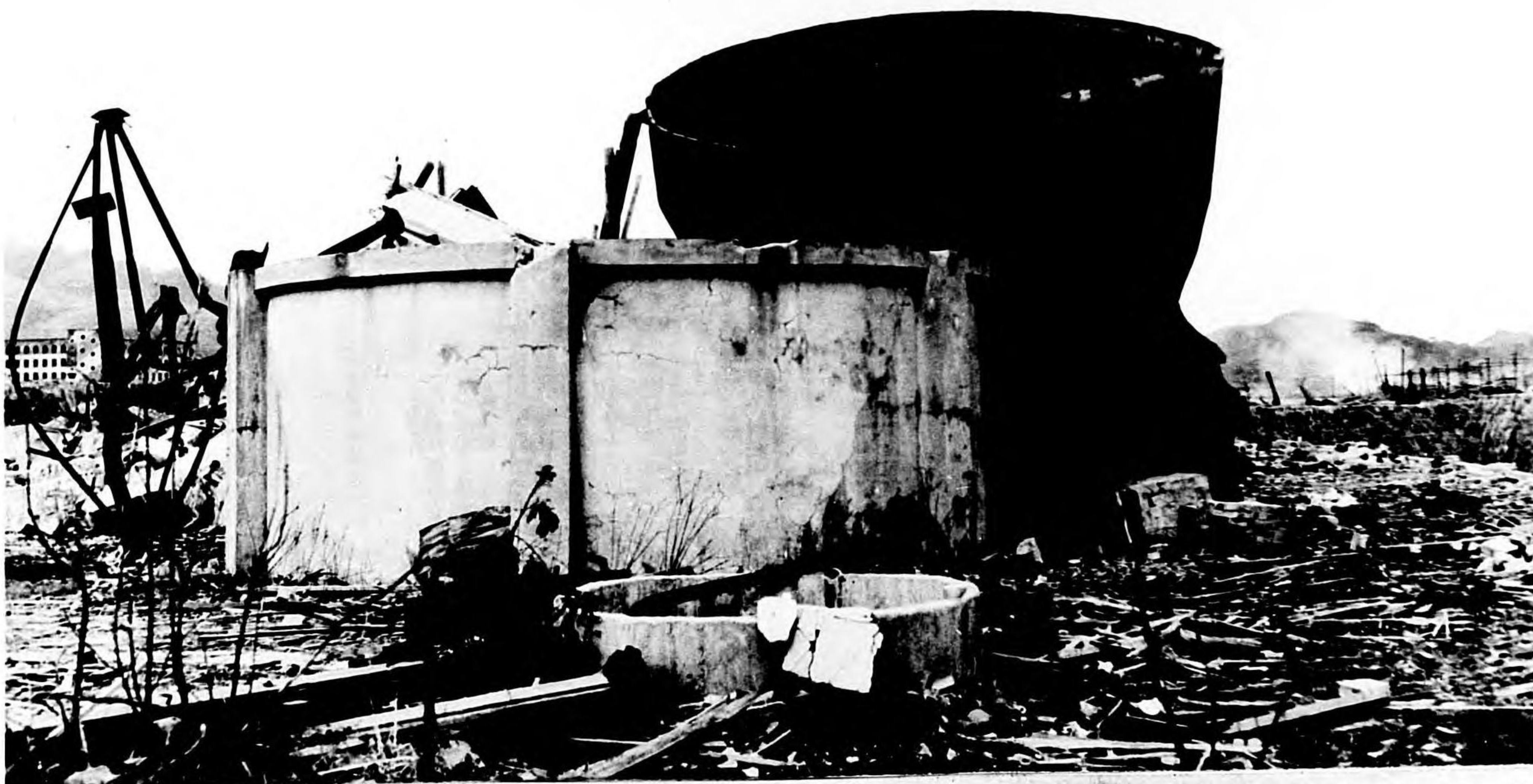
Photo 141. Nagasaki, 1,100 feet from GZ. Oxygen holder destroyed by blast and fire.
