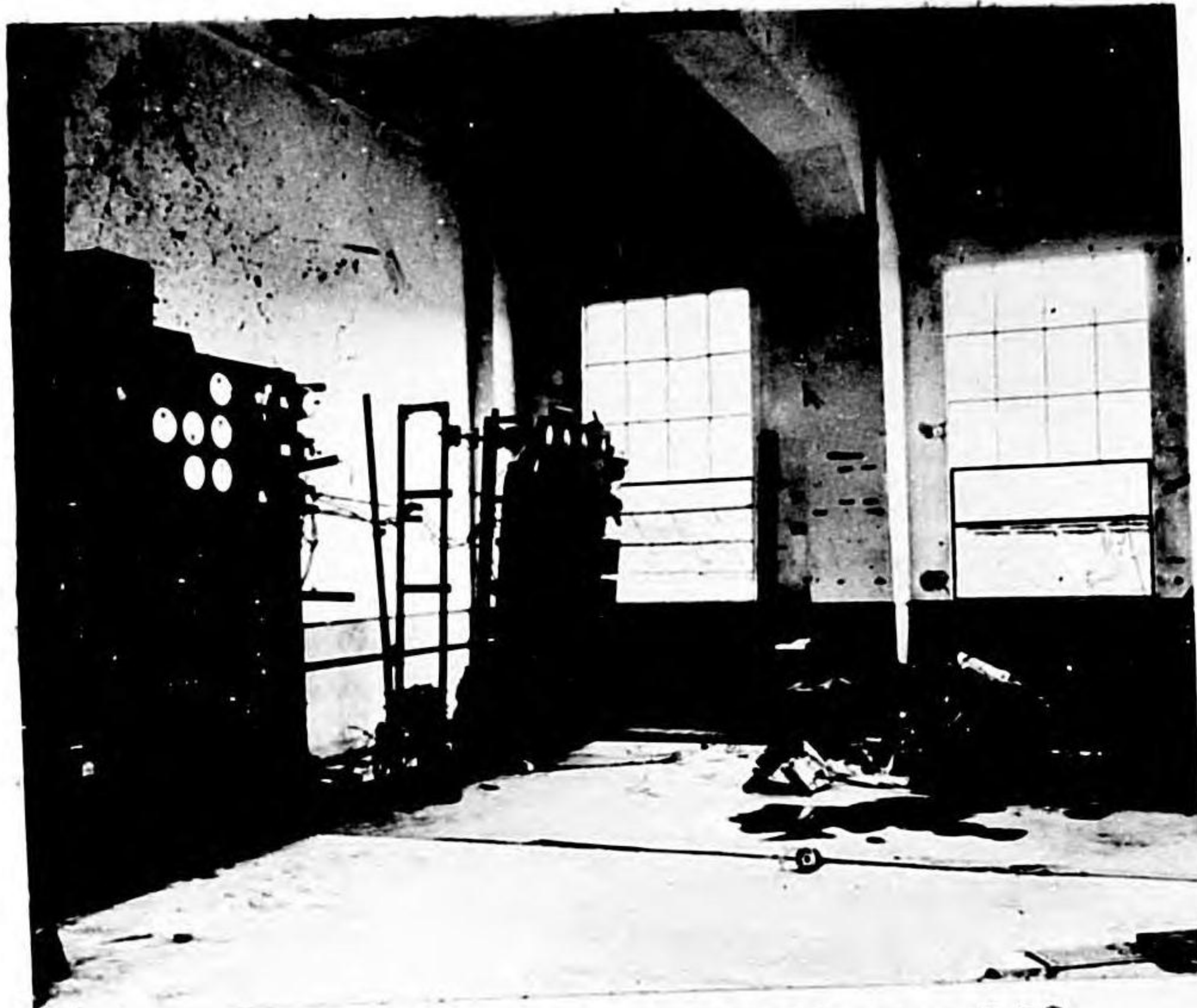
Photo 181. Same as Photo 180. Interior of switch room.
