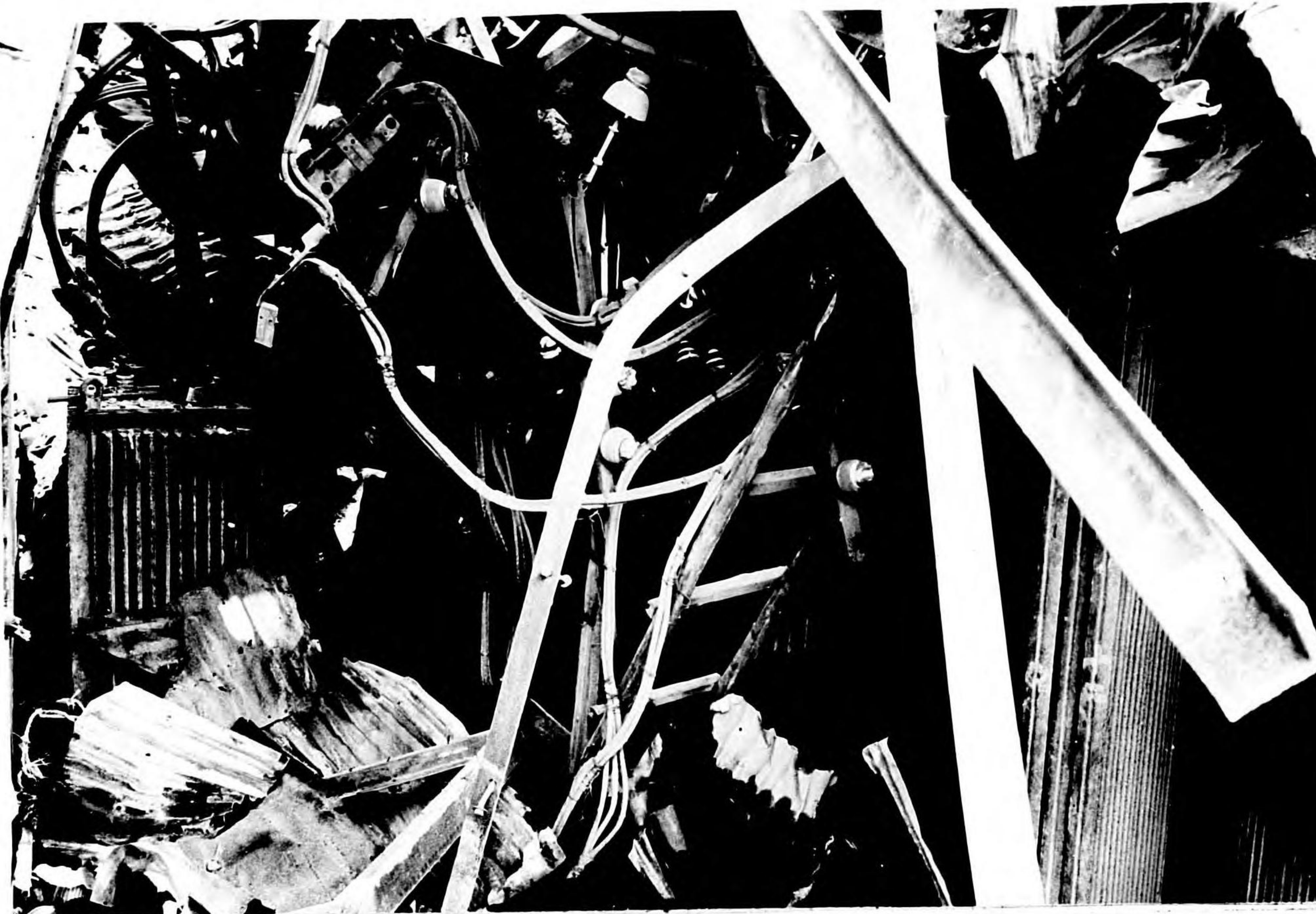
Photo 131. Nagasaki, 3,800 feet from GZ. Debris on transformers for electrical furnace.
