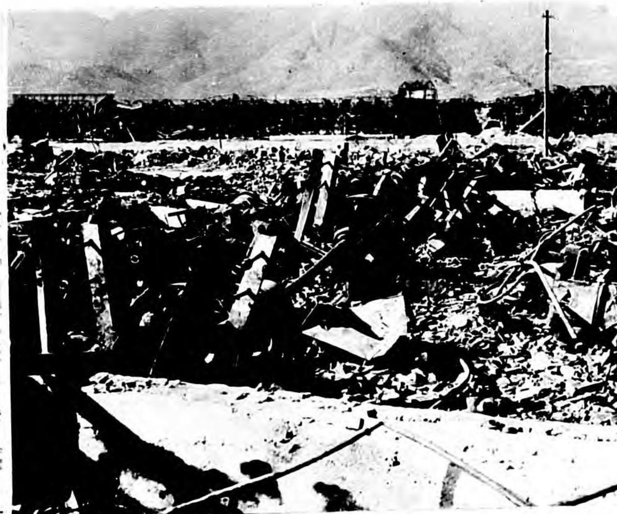
Photo 172. Nagasaki. Same as Photo 171. Wood-frame buildings totally damaged by blast and machine tools totally damaged by debris and fire.
