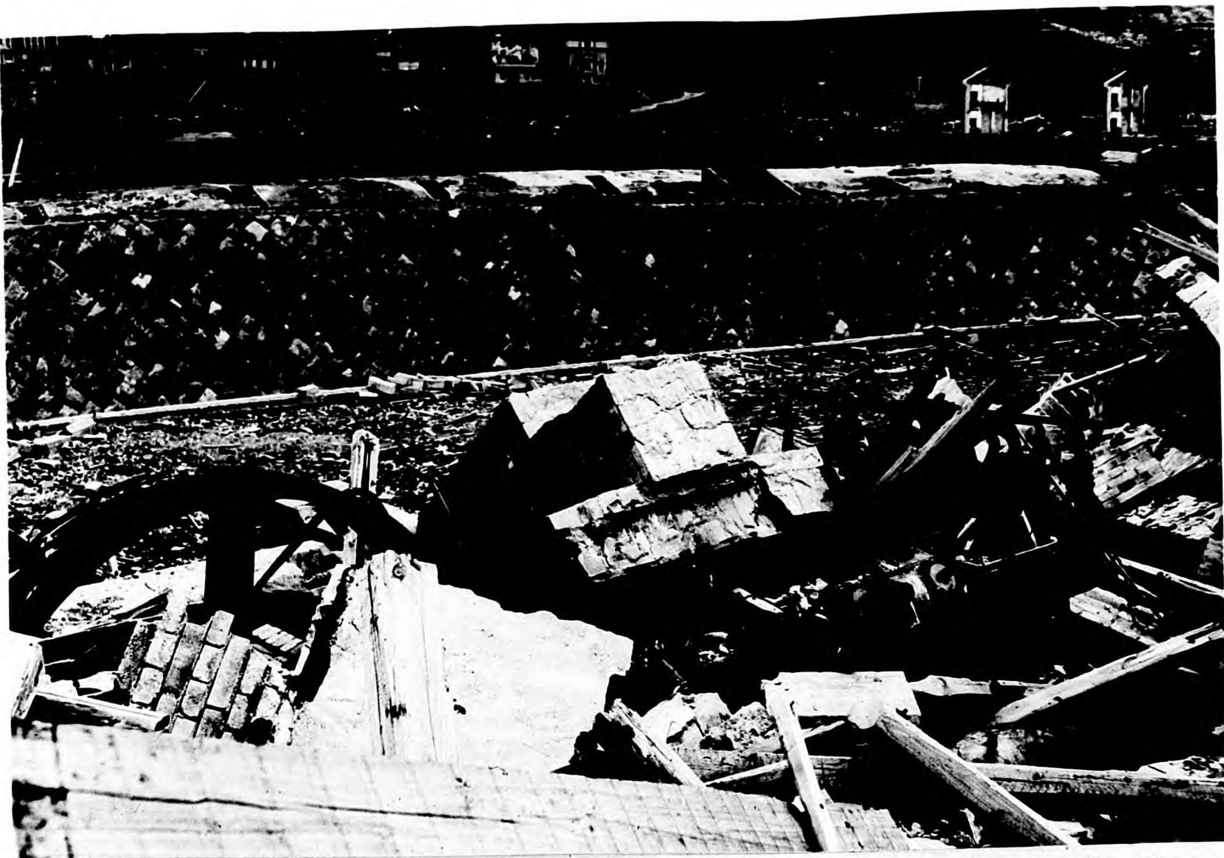
Photo 140. Nagasaki, 1,100 feet from GZ. Oxygen compressors heavily damaged by debris.
