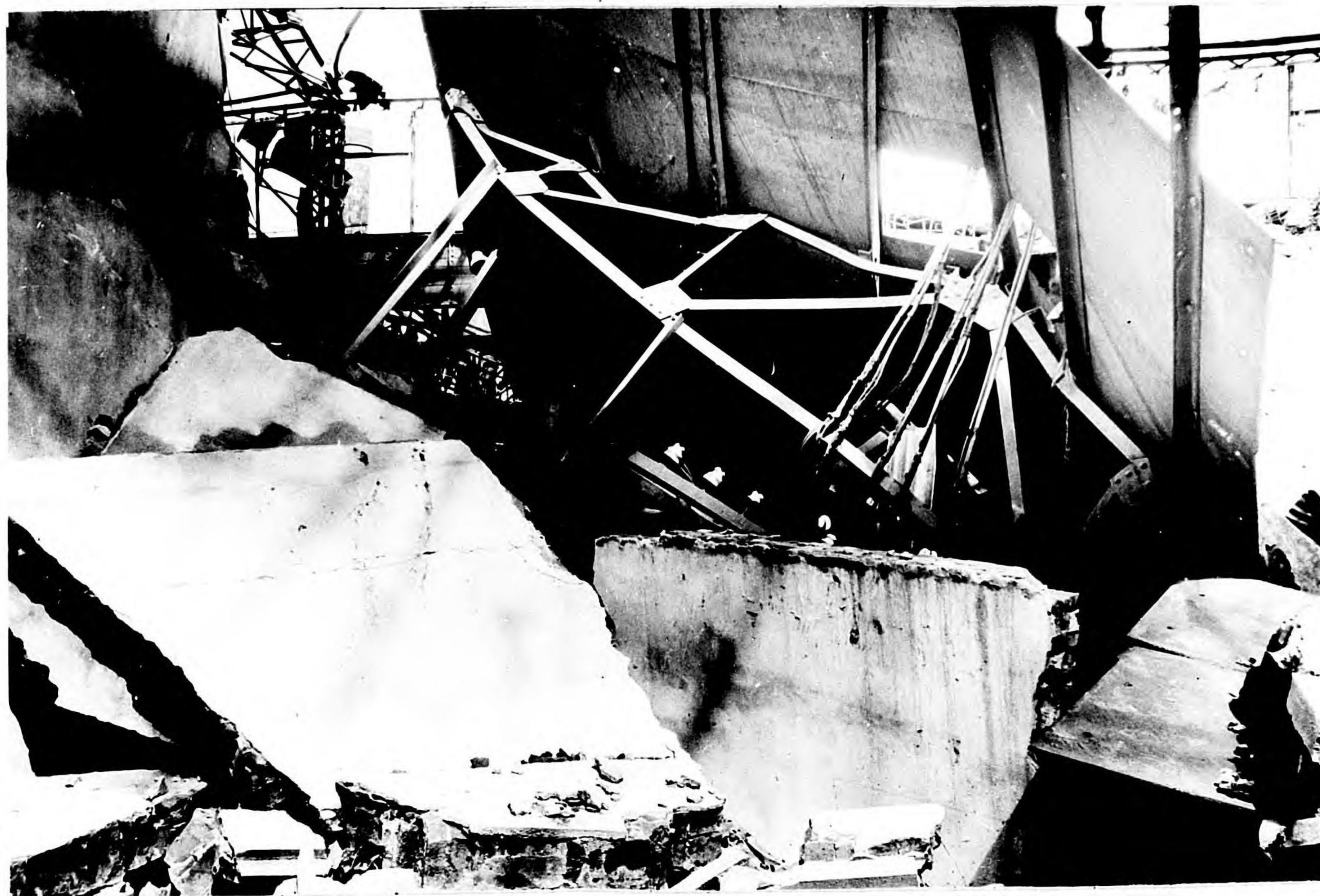
Photo 132. Nagasaki, 3,800 feet from GZ. Bus structure damaged by blast.
