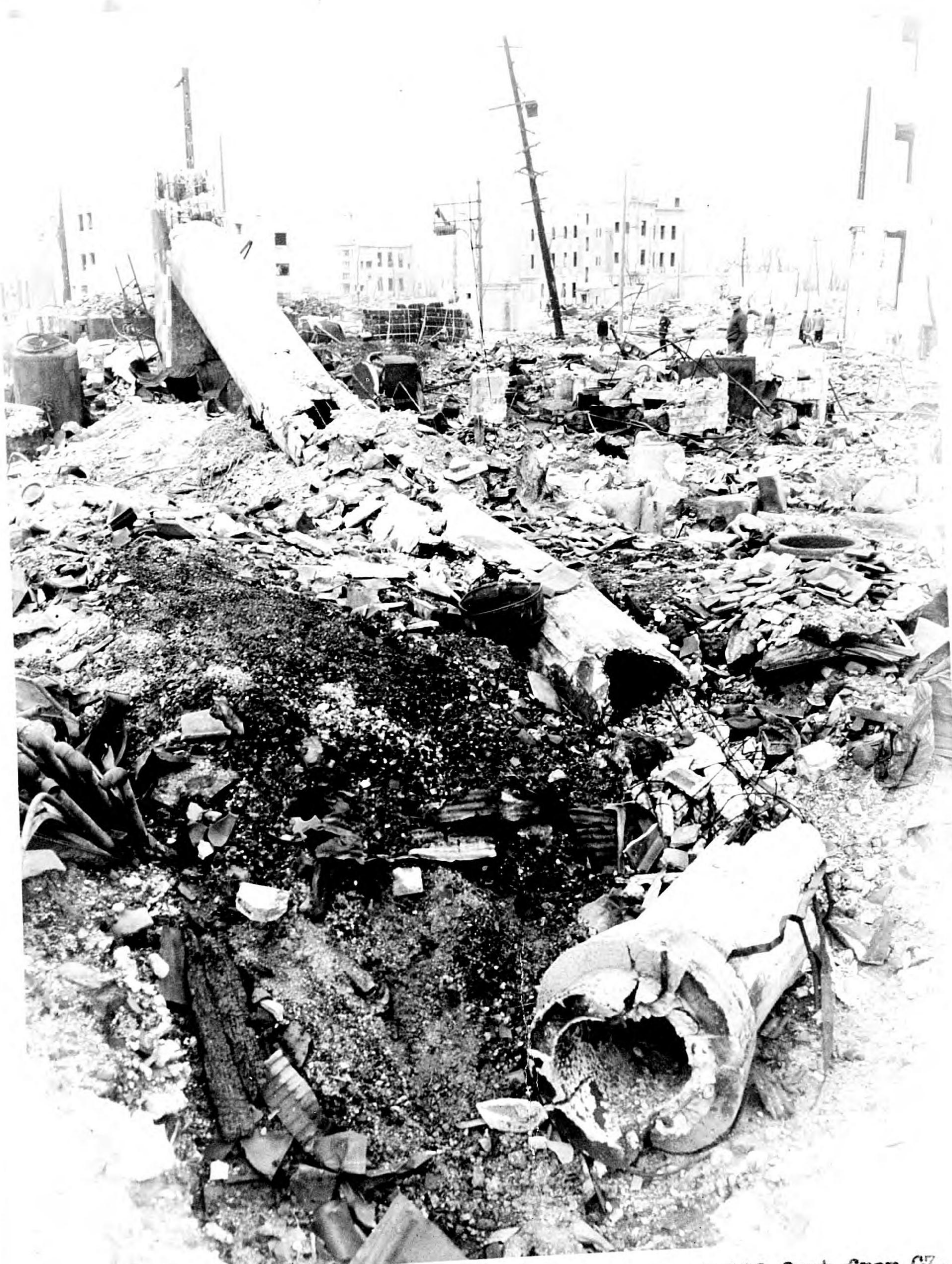
Photo 174. Hiroshima. Reinforced-concrete stack, 1,100 feet from GZ, 60 feet high, 4 feet in diameter, sheared off at 12 feet.
