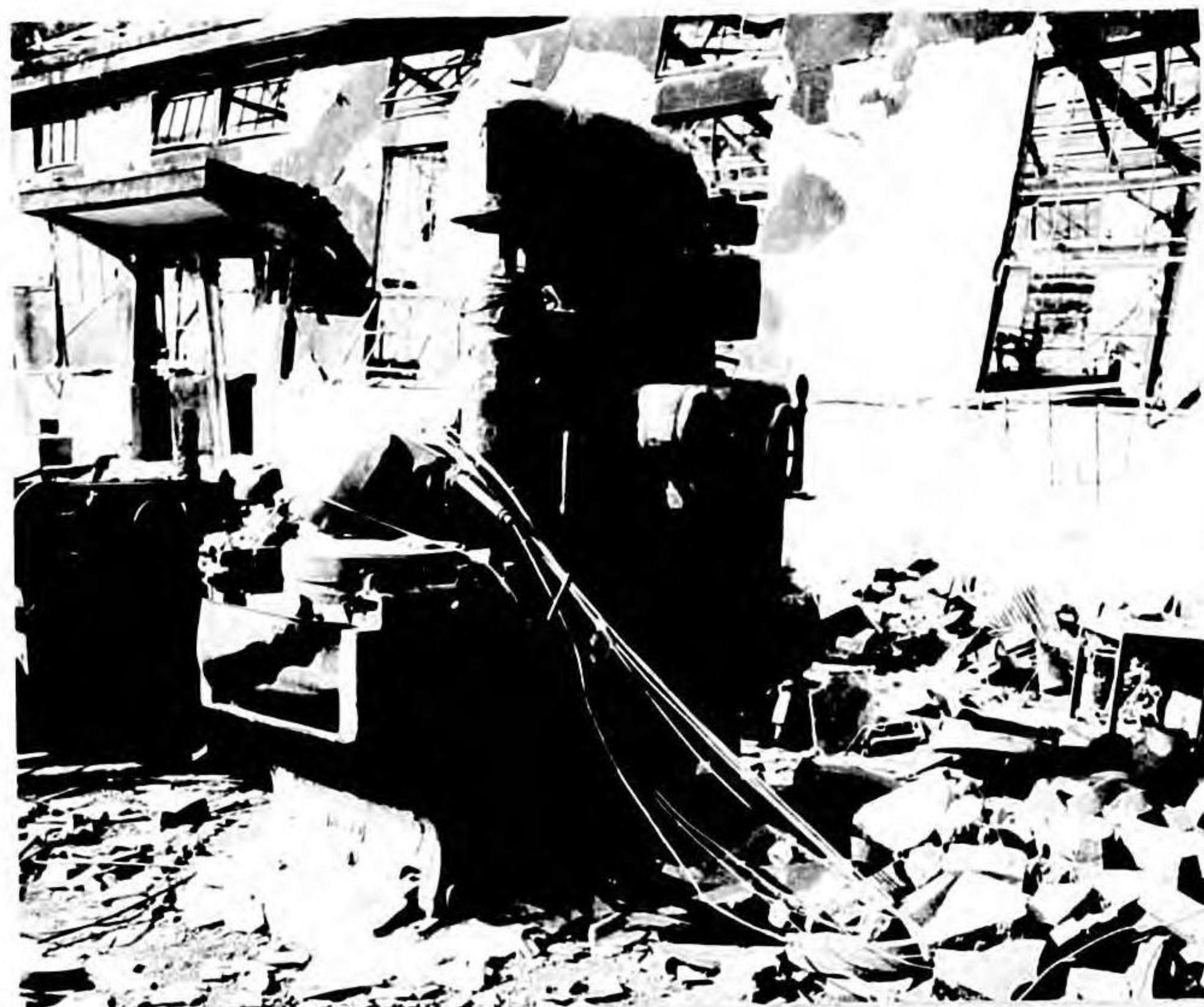
Photo 136. Nagasaki, 3,700 feet from GZ. Vertical miller damaged by fire.
