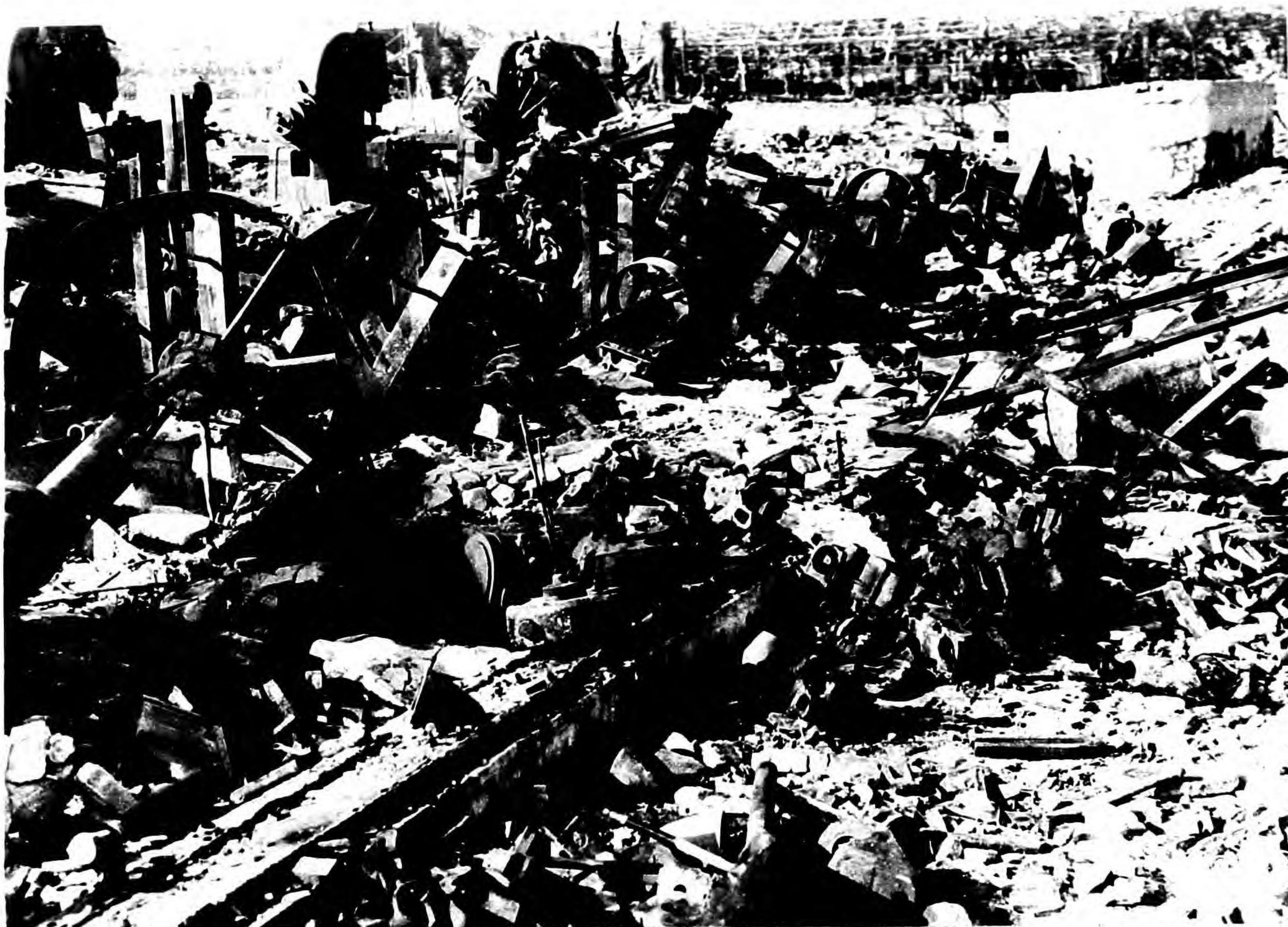
Photo 168. Nagasaki. Mitsubishi Boys Industrial School. Wood-frame building used for industrial purposes totally damaged by blast and fire. Machine tools totally or heavily damaged by blast, debris, and fire.
