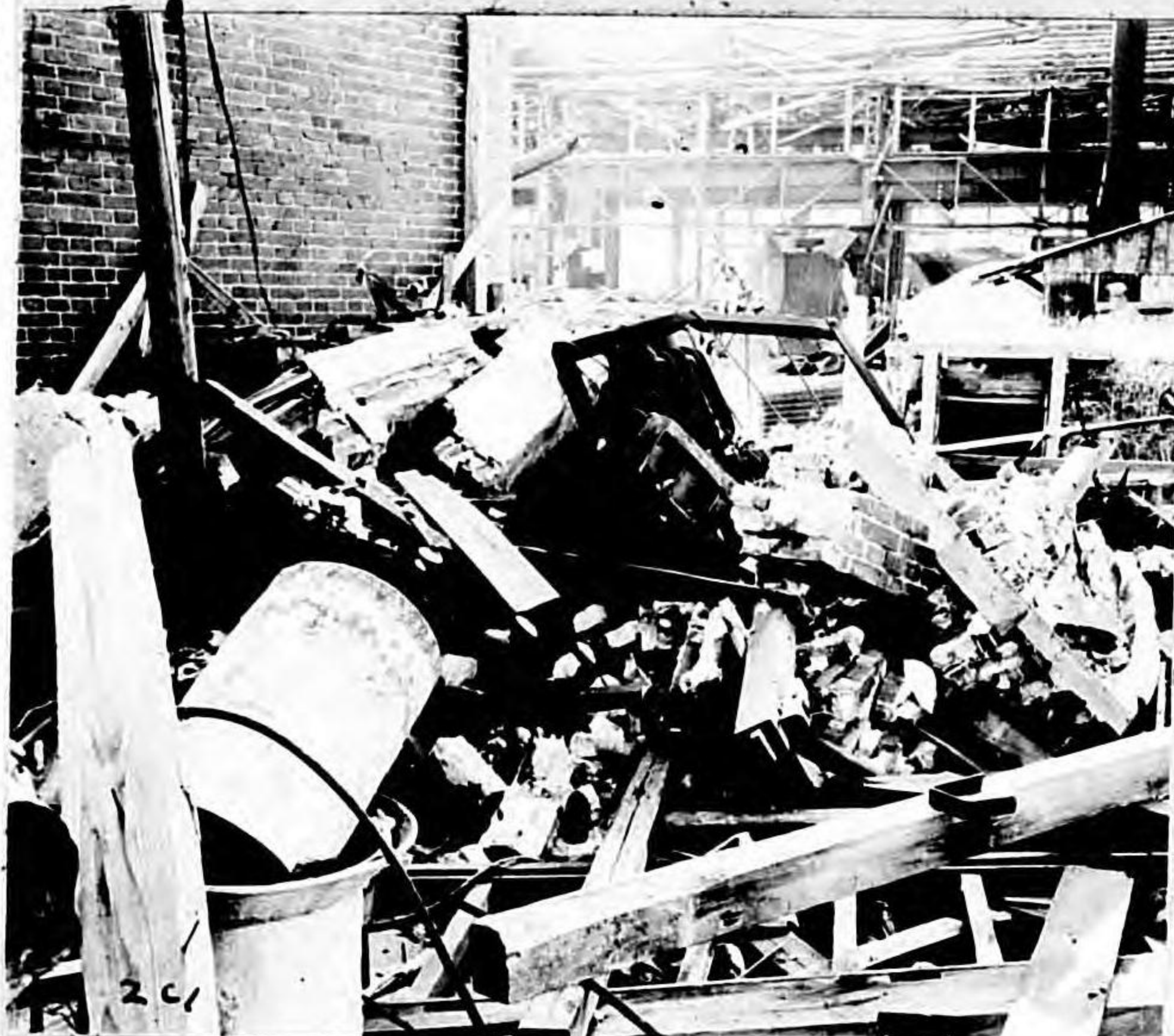
Photo 130. Nagasaki, 3,800 feet from GZ. Transformers overturned but undamaged by blast and debris.
