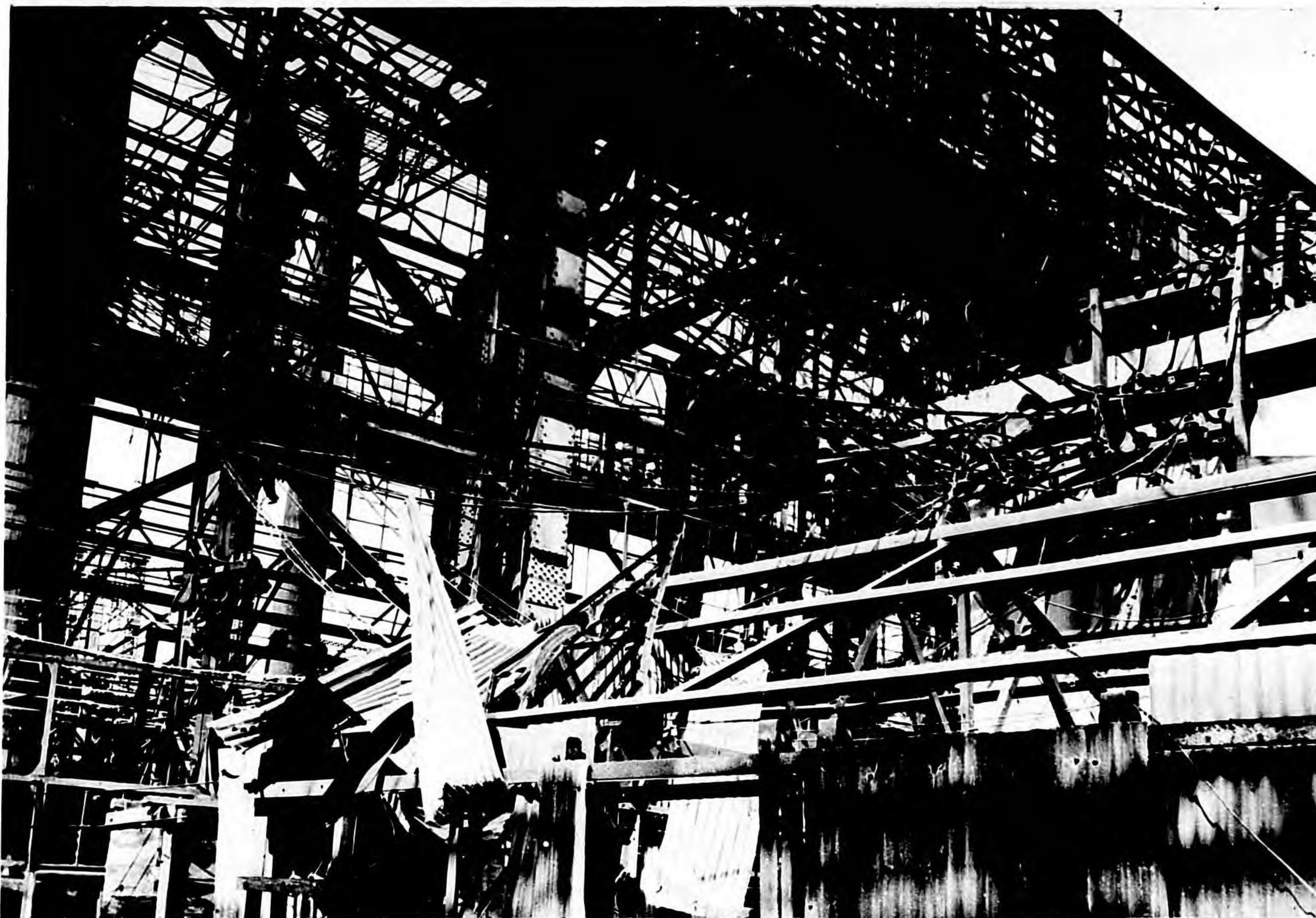
Photo 134. Nagasaki, 3,900 feet from GZ. Typical arrangement of electrical wiring.
