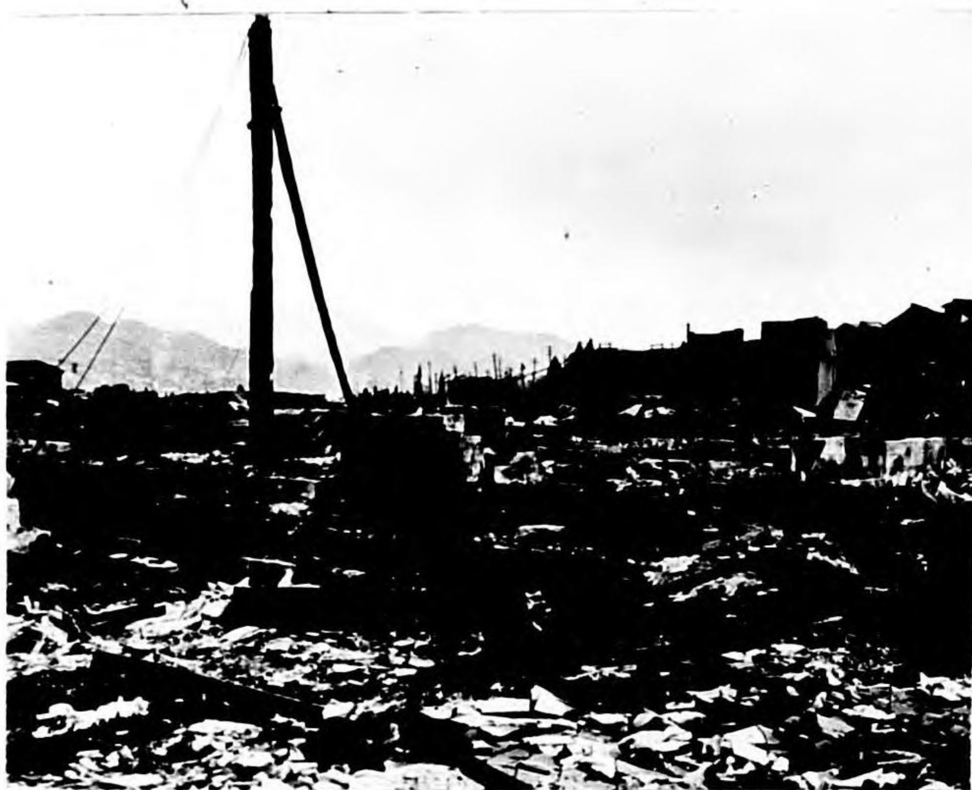
Photo 164. Nagasaki. Wood and steel-frame building of Standard-Vacuum Oil Works, 6,500 feet from GZ, totally damaged by blast and fire.
