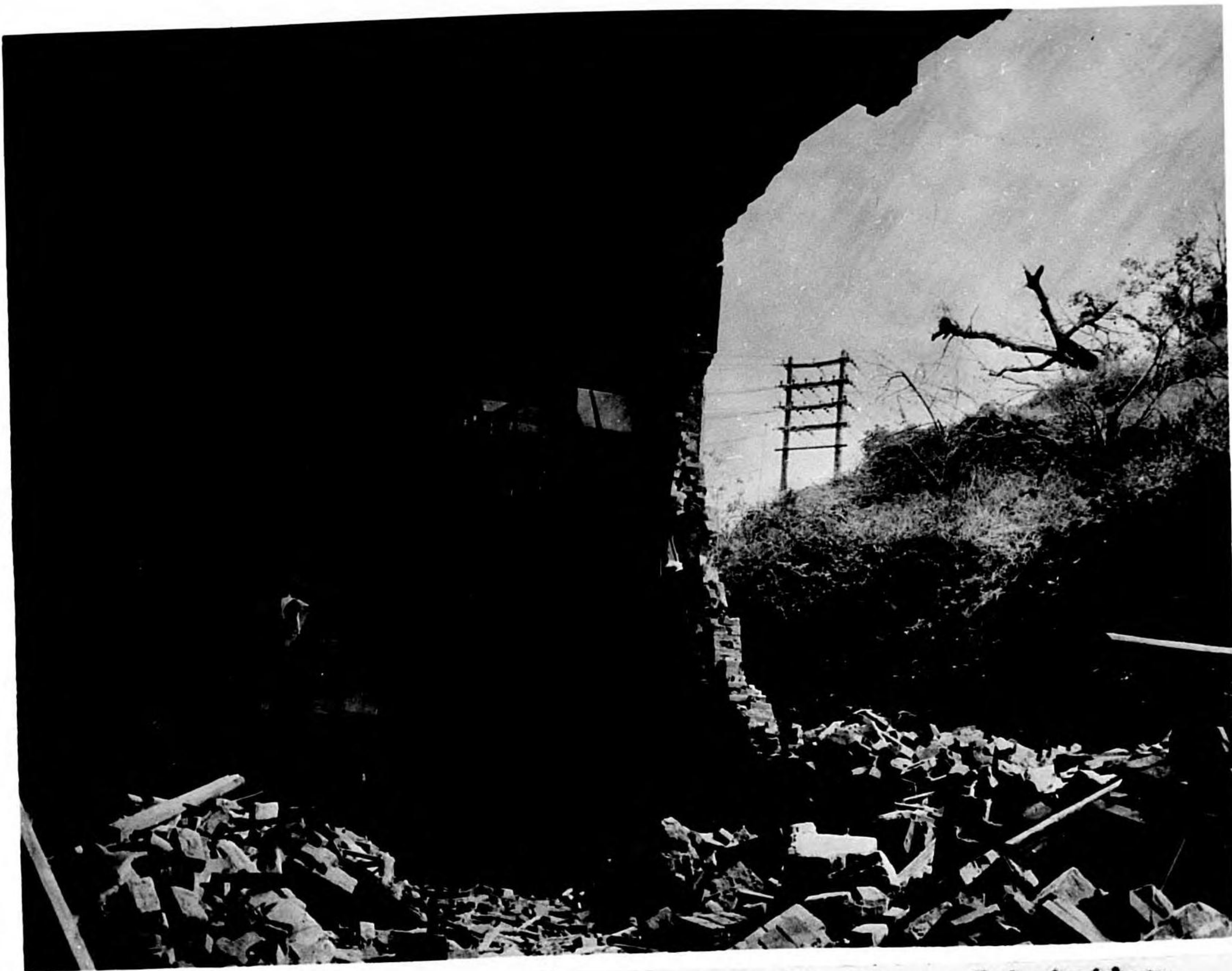
Photo 124. Nagasaki, 5,400 feet from GZ, Zenza Substation. Southeast corner of control and switch room.
