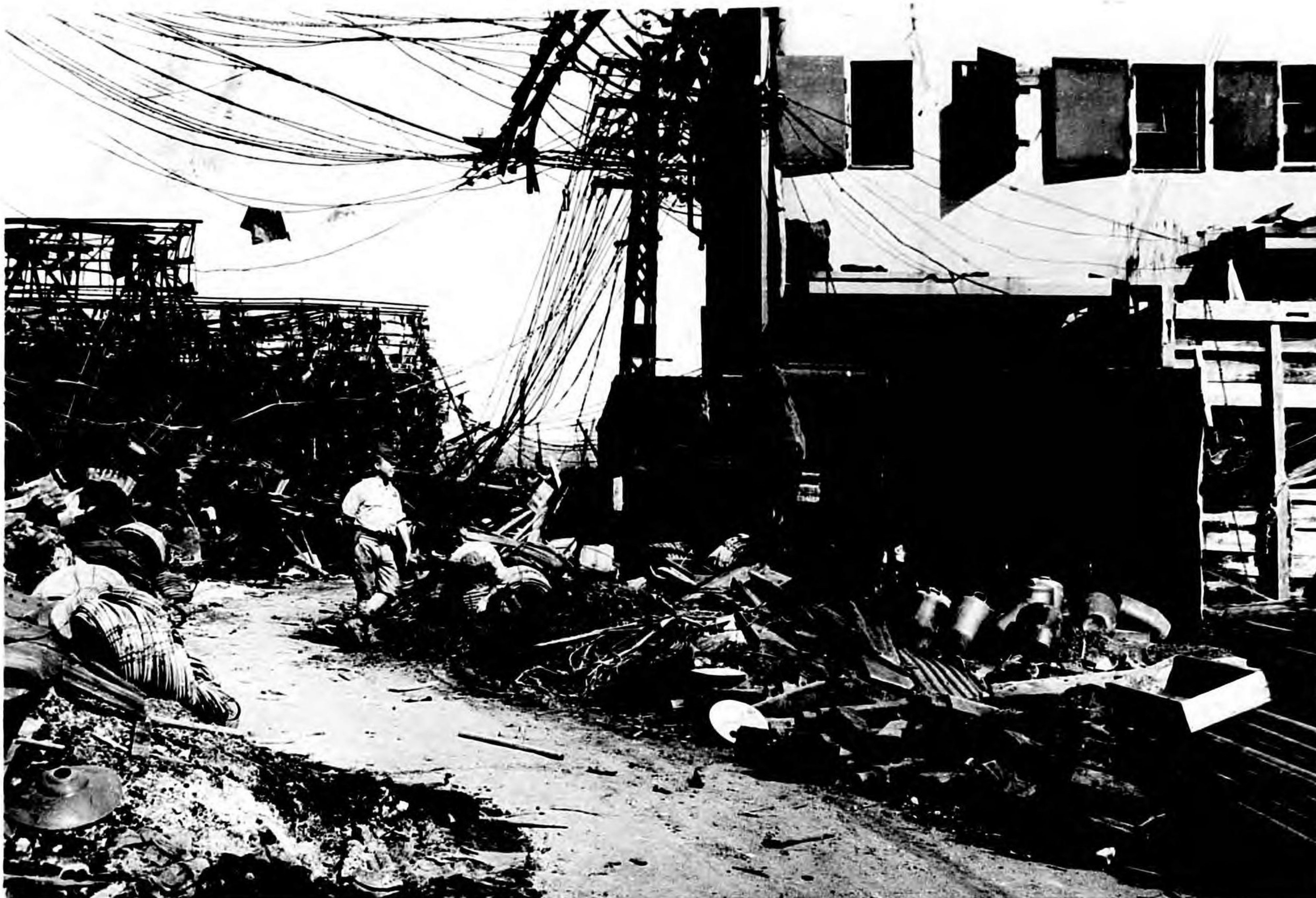
Photo 133. Nagasaki, 3,400 feet from GZ. Typical blast damage to overhead wiring.
