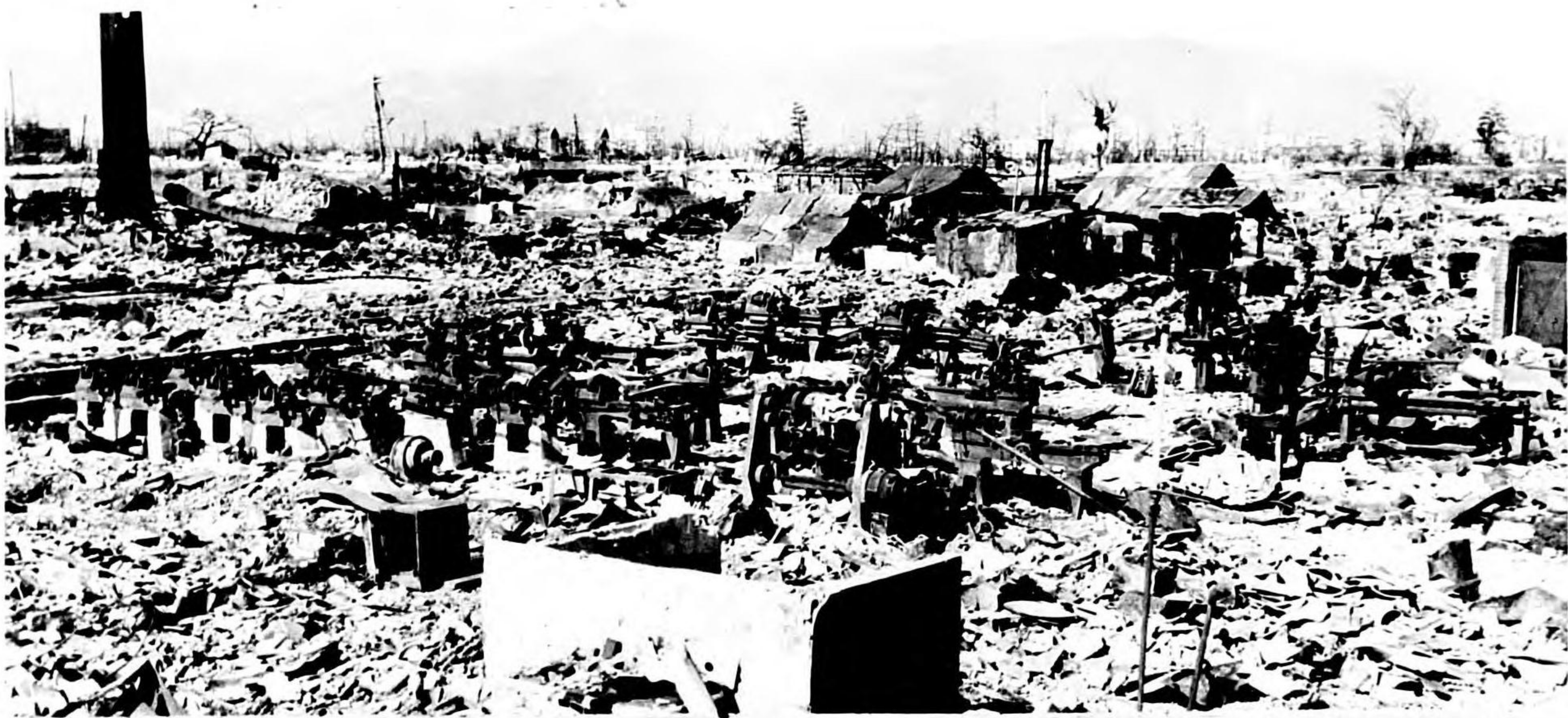
Photo 163. Hiroshima, 6,500 feet from GZ. Wood-frame, light-engineering shop structurally damaged by blast and then consumed by fire.
