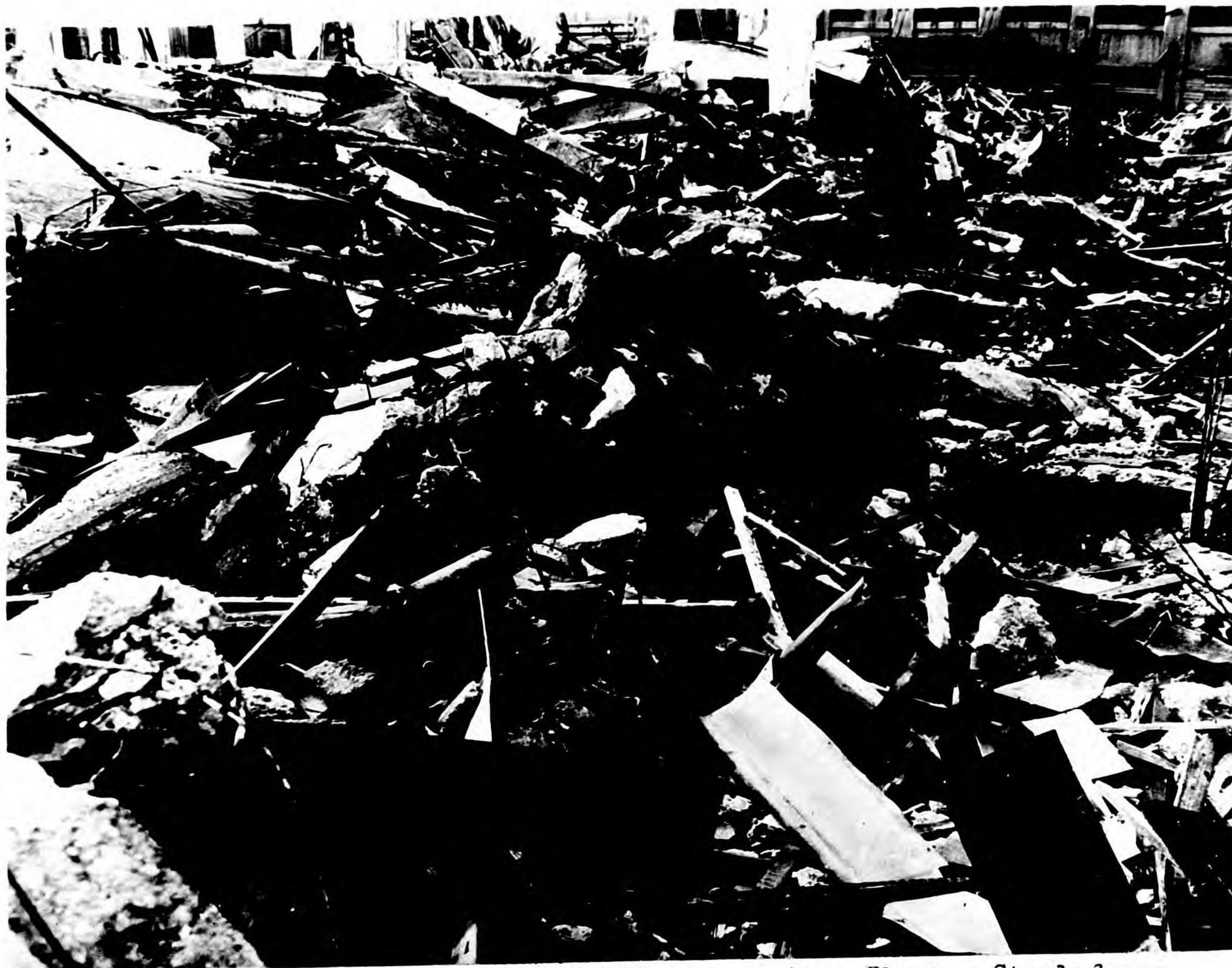
Photo 170. Nagasaki. Mitsubishi Steel and Arms Plant. Steel-frame building damaged by blast and machines totally damaged by collapse of reinforced-concrete roof.
