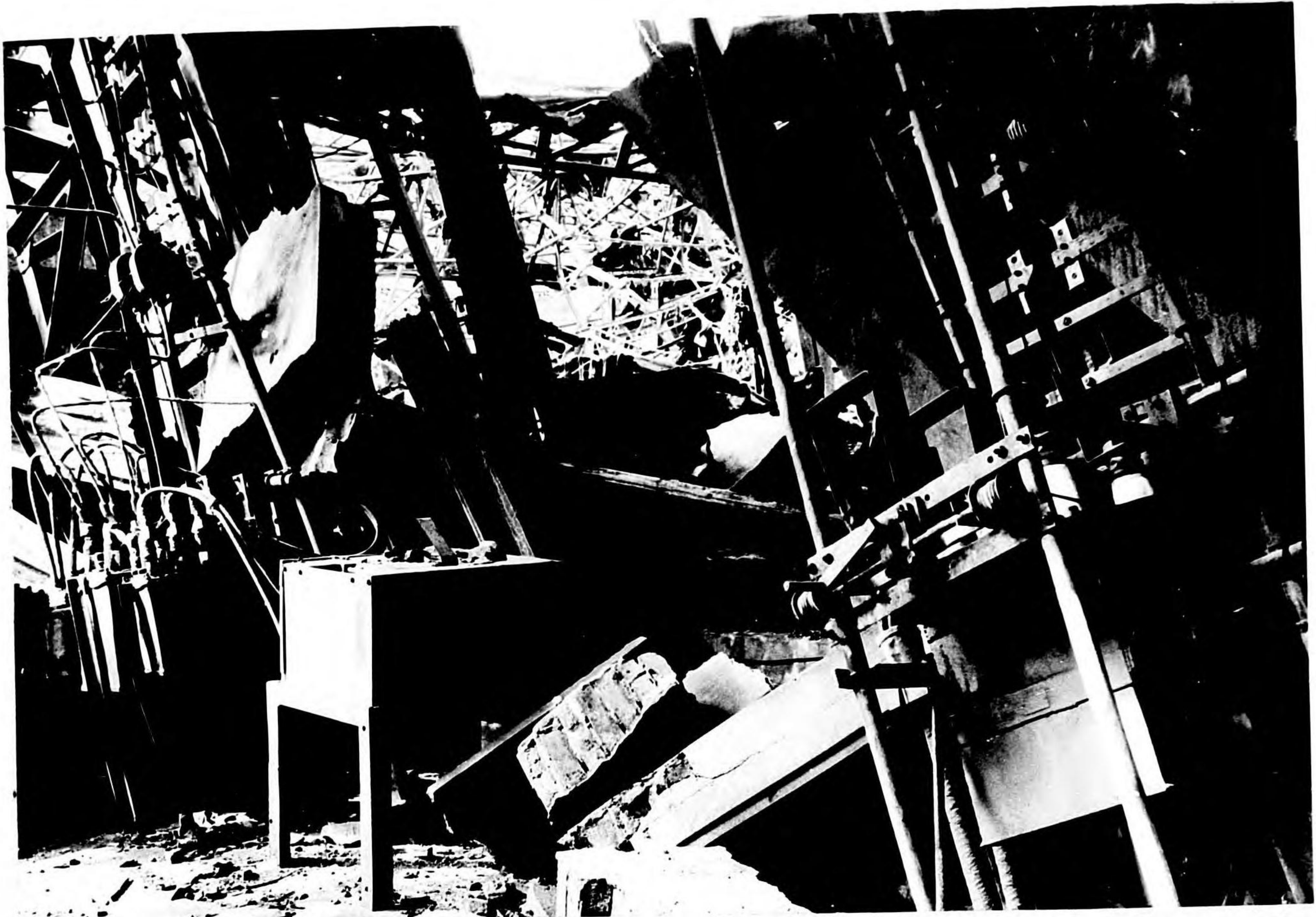
Photo 120. Nagasaki, 2,500 feet from GZ. Switchboard and circuit breakers heavily damaged by blast.
