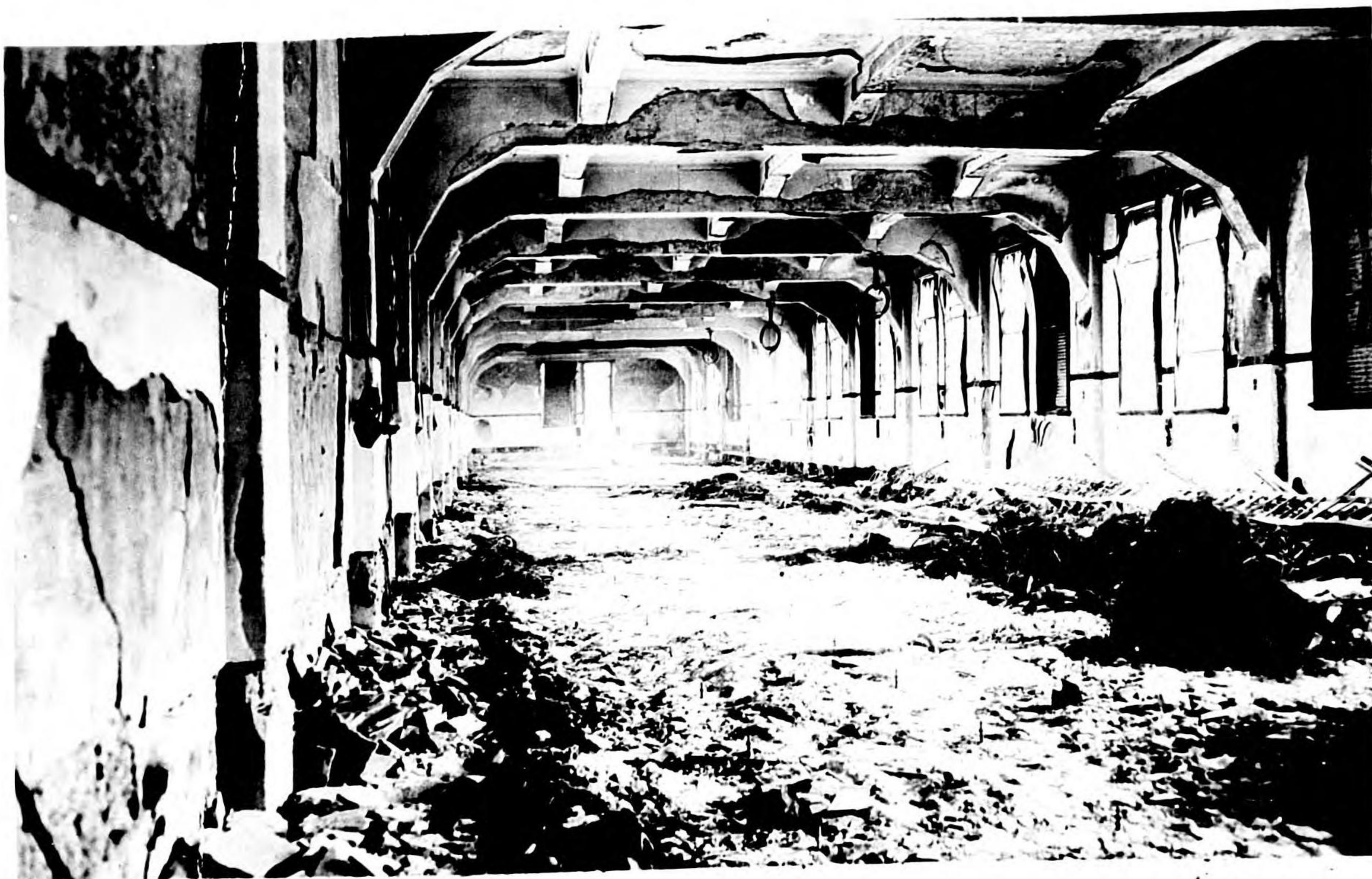
Photo 177. Hiroshima. Bureau of Telephones Central District exchange building. Damage to equipment in reinforced-concrete building 2,000 feet from GZ.
