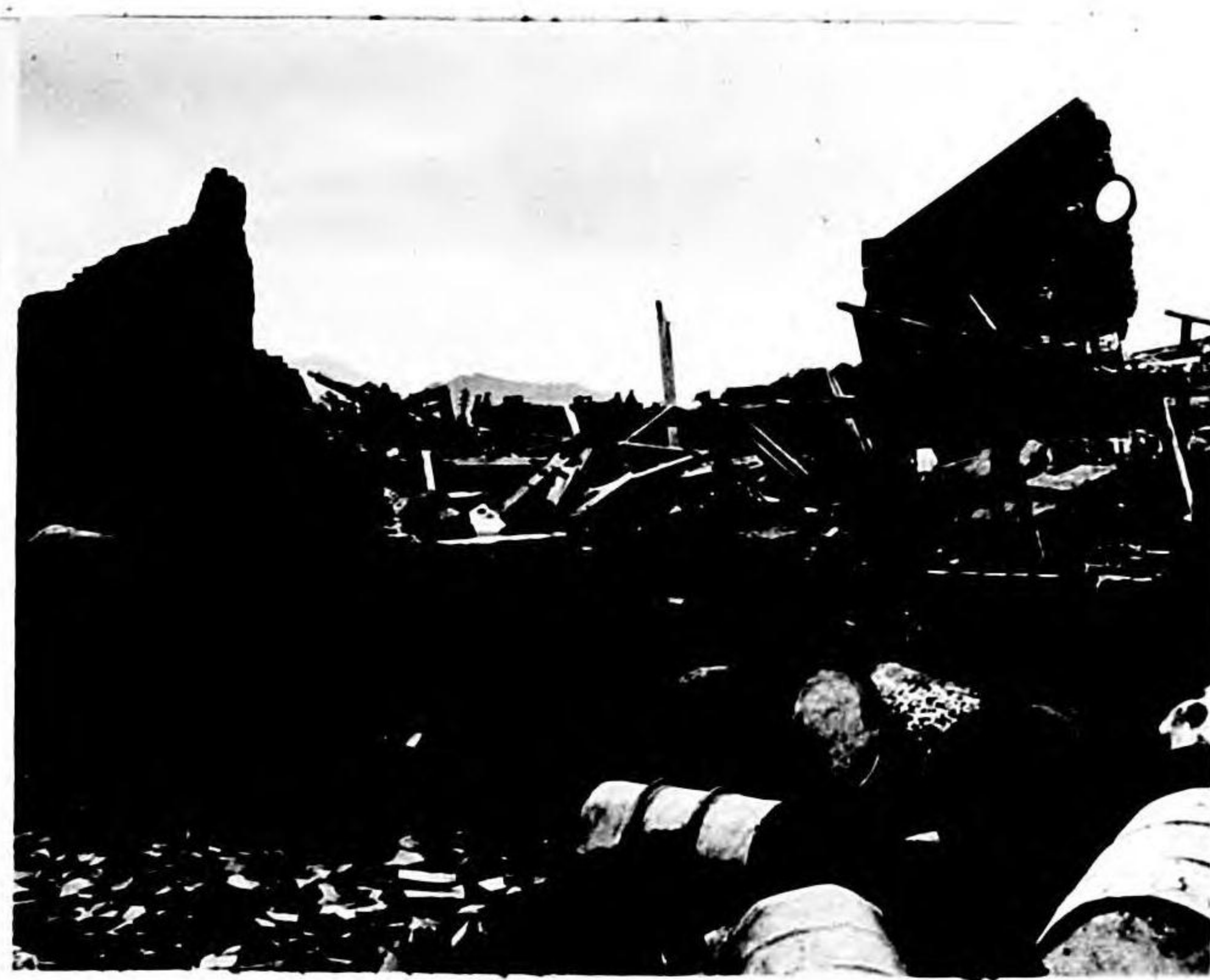
Photo 165. Nagasaki. Load-bearing brick wall and wood-frame construction of Standard-Vacuum Works totally damaged by blast.
