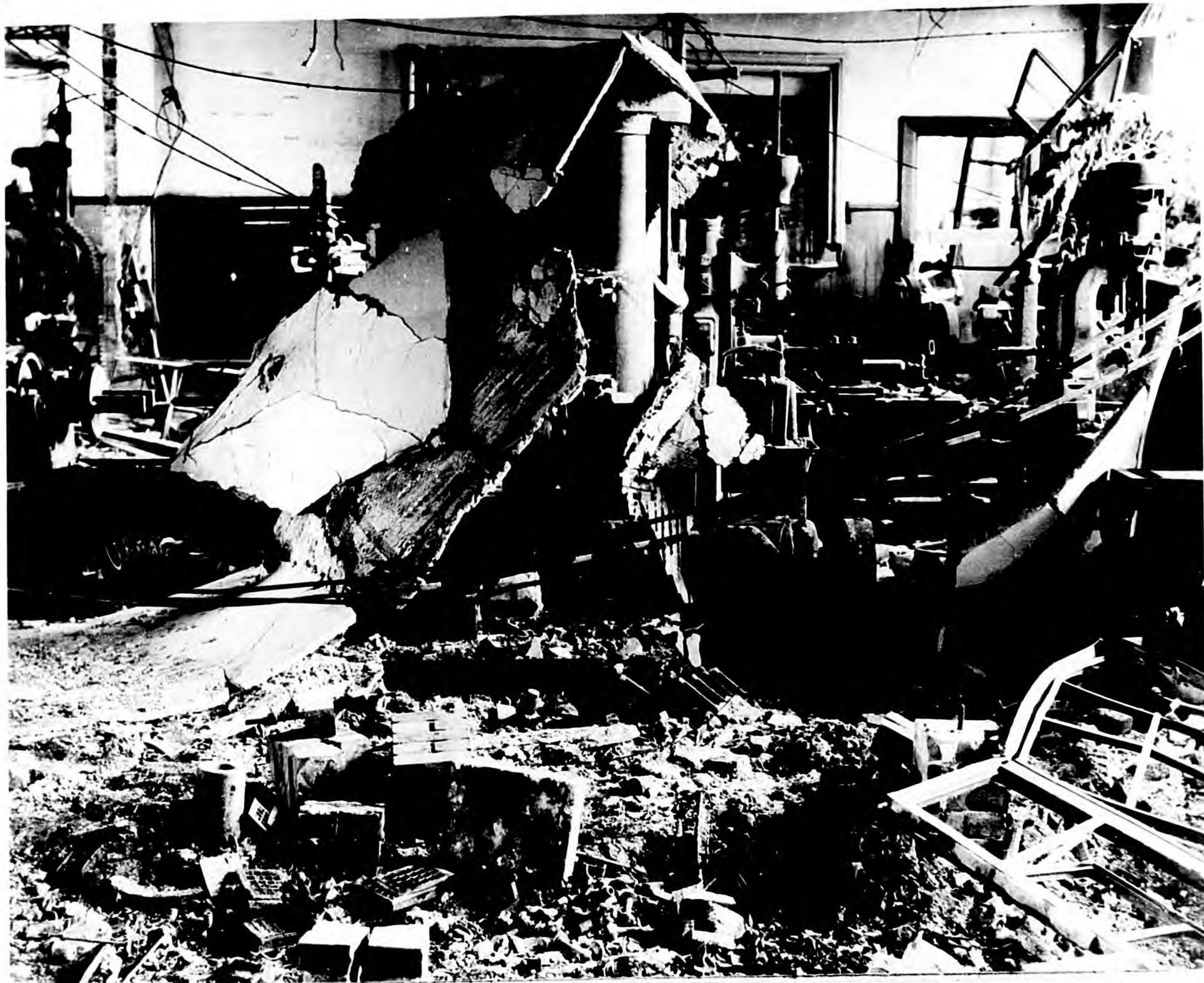
Photo 135. Nagasaki, 3,700 feet from GZ. Radial driller on first floor damaged by debris and fire.
