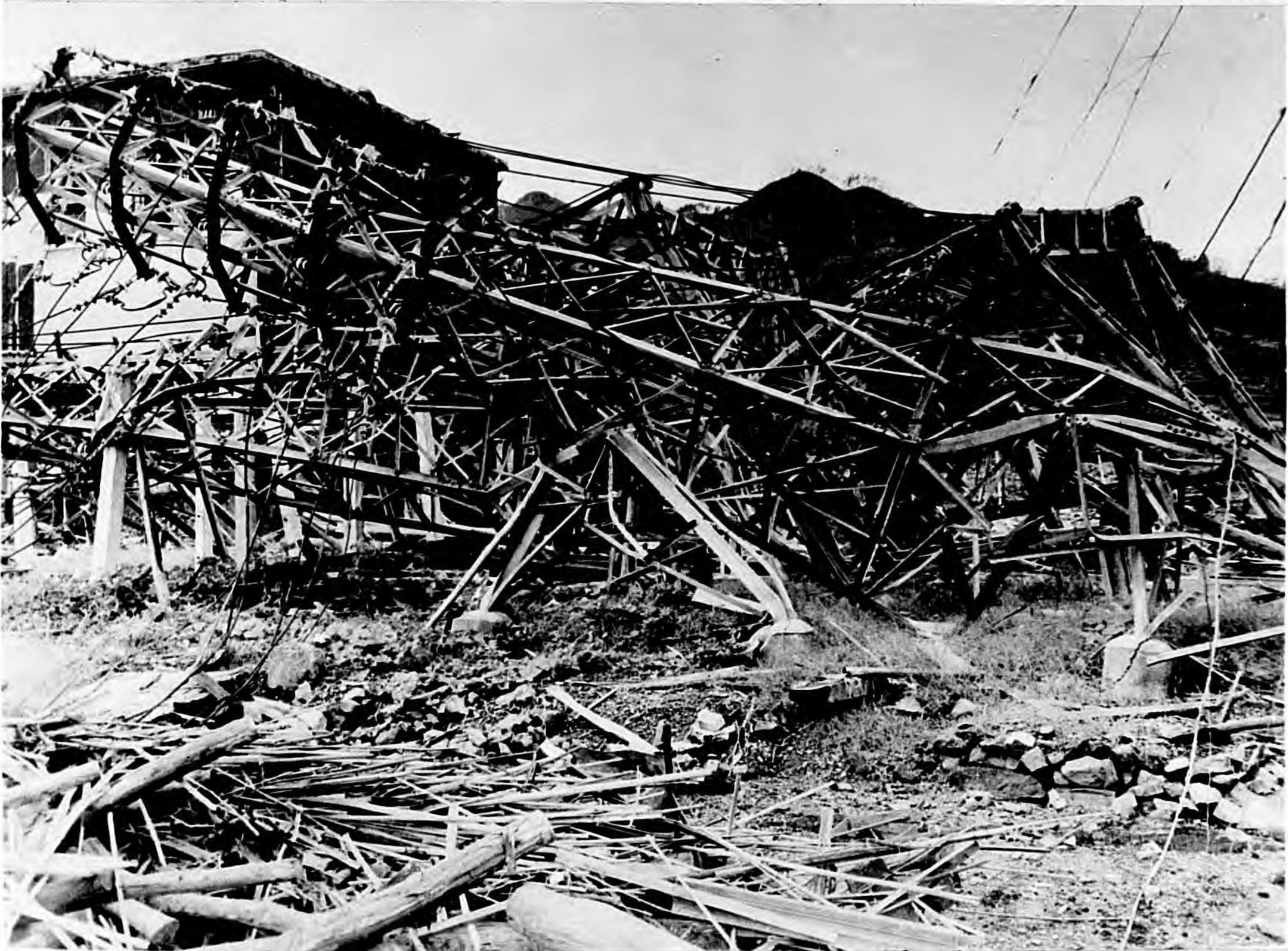
Photo 123. Nagasaki, 3,600 feet from GZ, Takenokube Substation. Damage to 3.5-kv switch rack and first tower.
