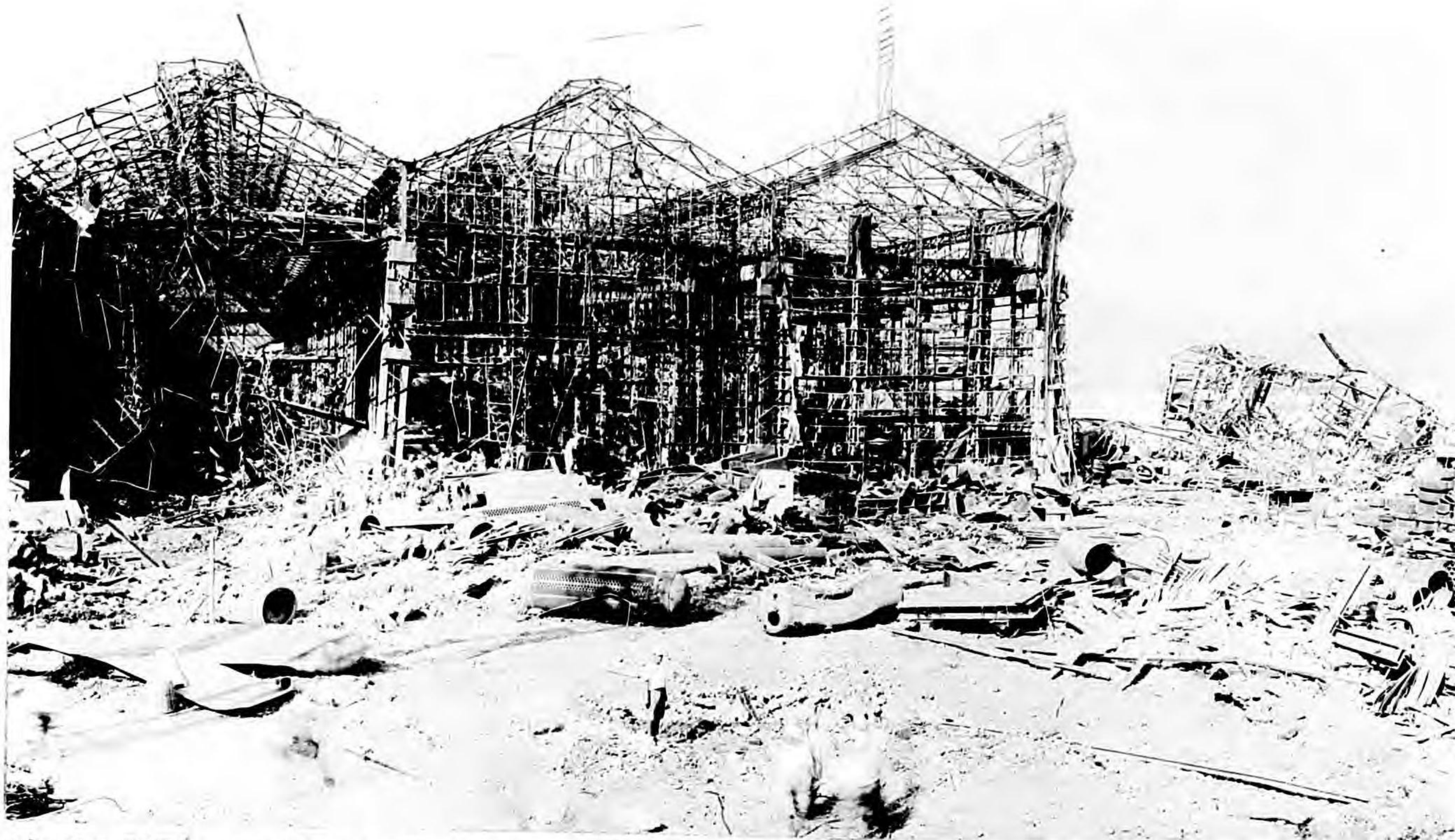
Photo 167. Akuncoura Engine Works. Steel-frame boiler shop which suffered heavy structural and superficial damage from high-explosive bombs, but little additional damage from atomic bomb.
