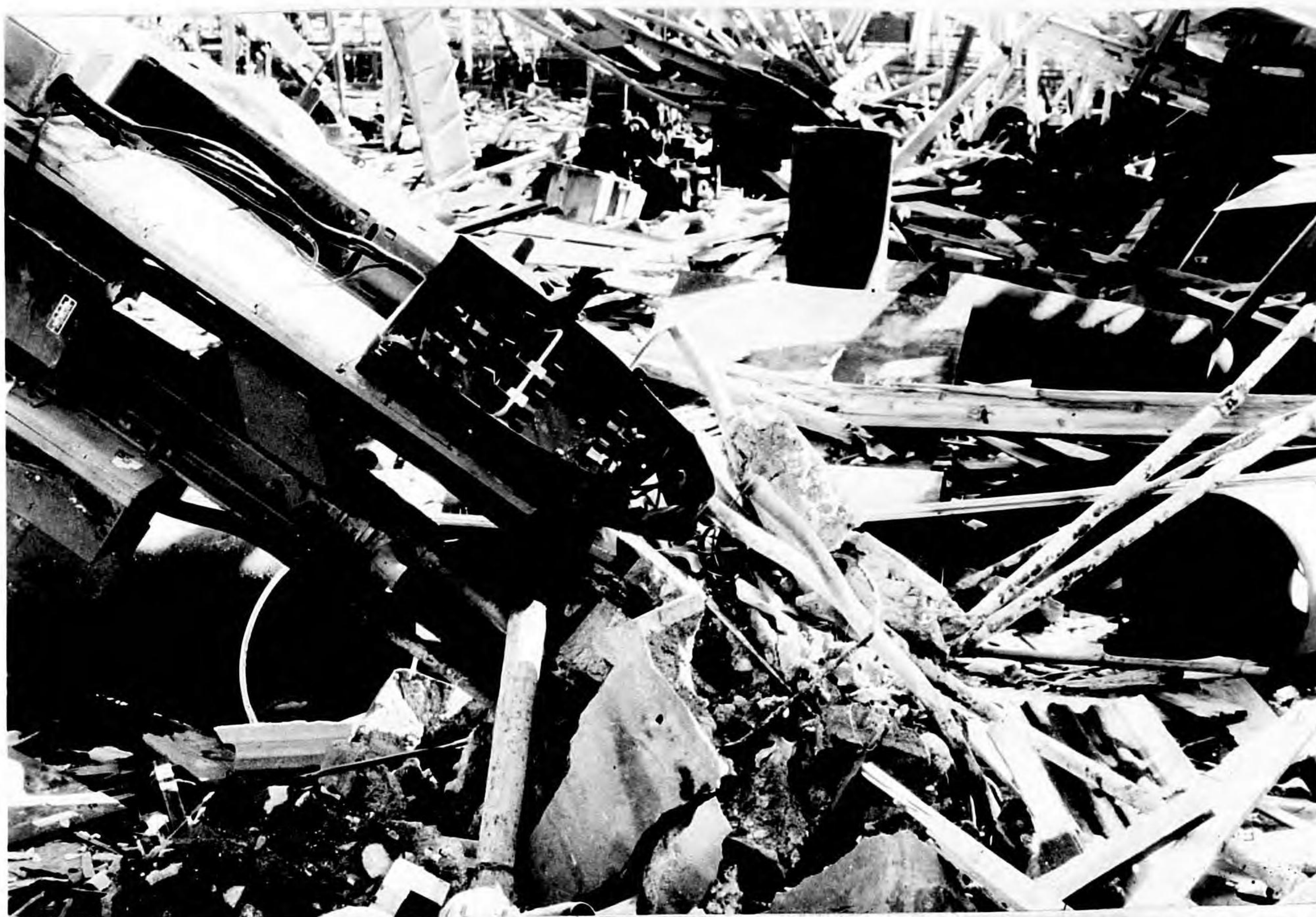
Photo 138. Nagasaki, 4,200 feet from GZ. Utilities destroyed by collapsed structure.
