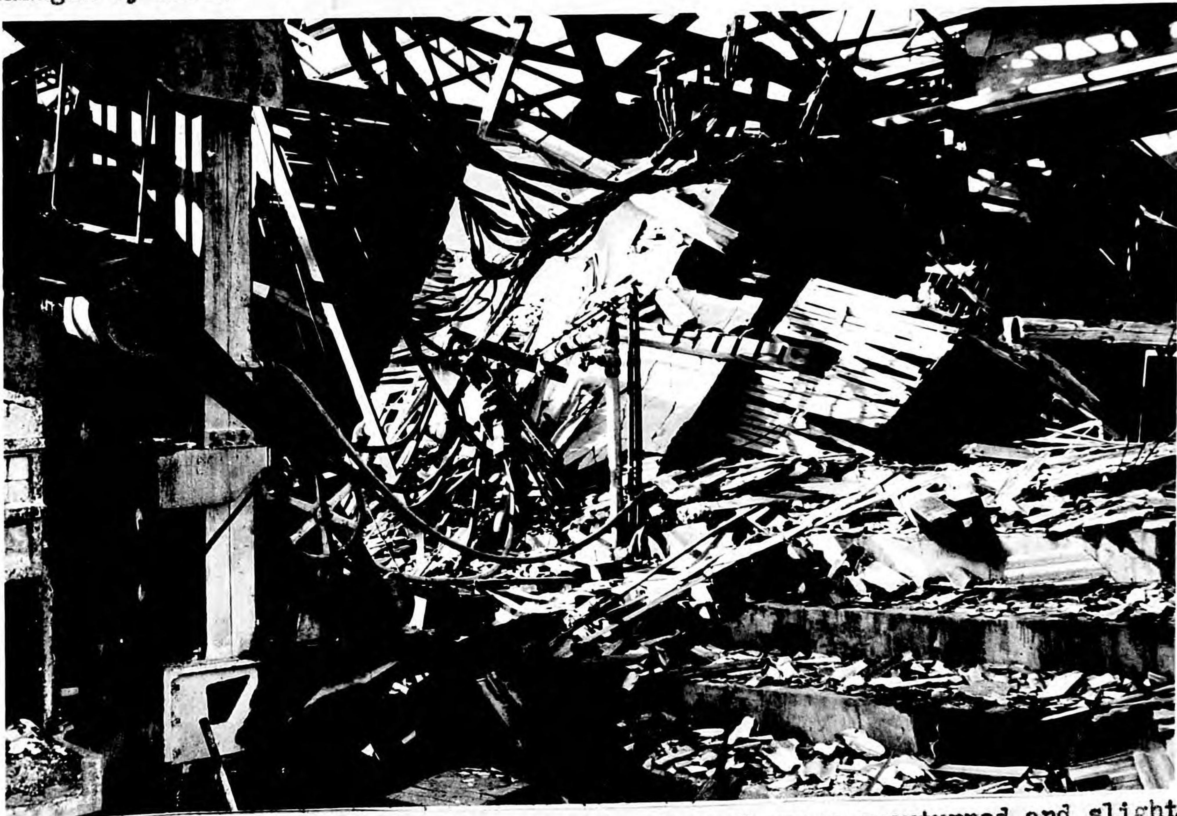
Photo 126. Nagasaki, 5,000 feet from GZ. Switchboard overturned by blast and damaged by fire.
