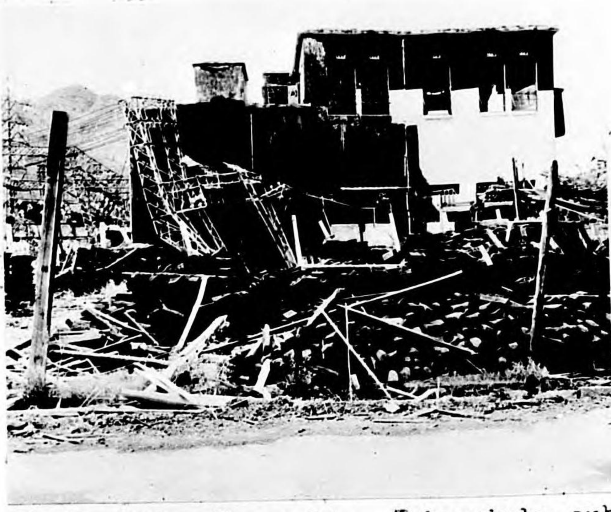
Photo 180. Nagasaki. Takenokubo substation, 3,600 feet from GZ. Unusually heavy concrete and steel construction withstood blast well.
