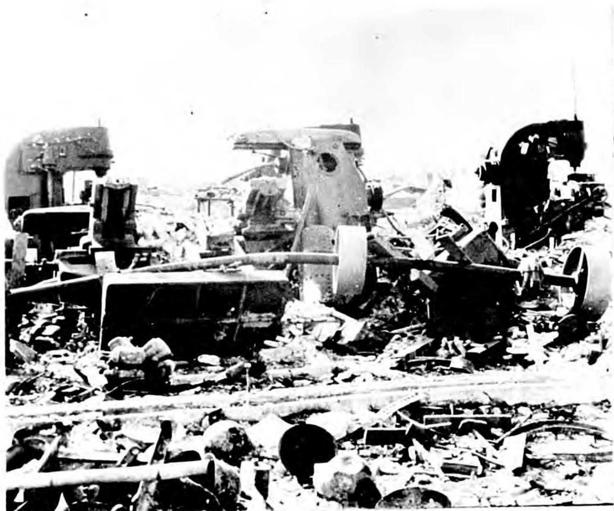
Photo 171. Nagasaki. Mitsubishi Boys Industrial School. Wood-frame building totally damaged by blast, but vertical millers still standing.
