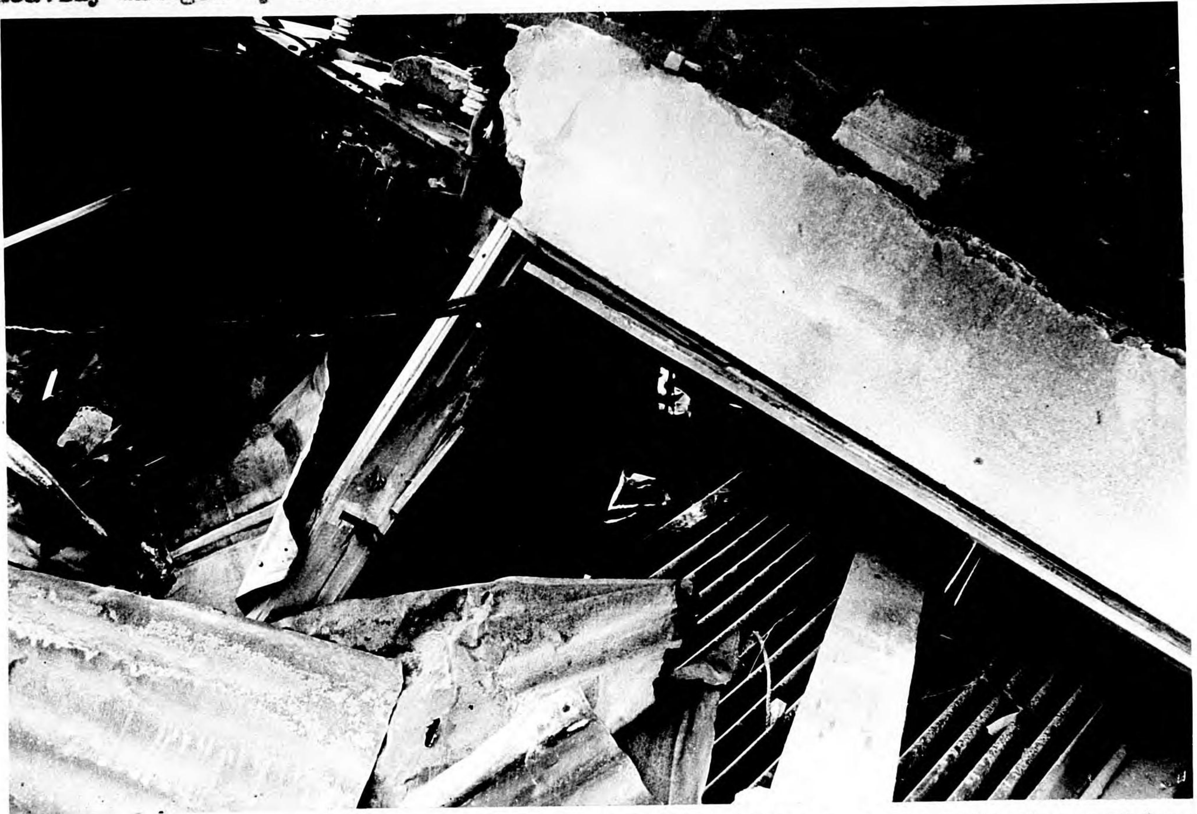
Photo 121. Nagasaki, 2,500 feet from GZ. Transformers slightly damaged by debris.
