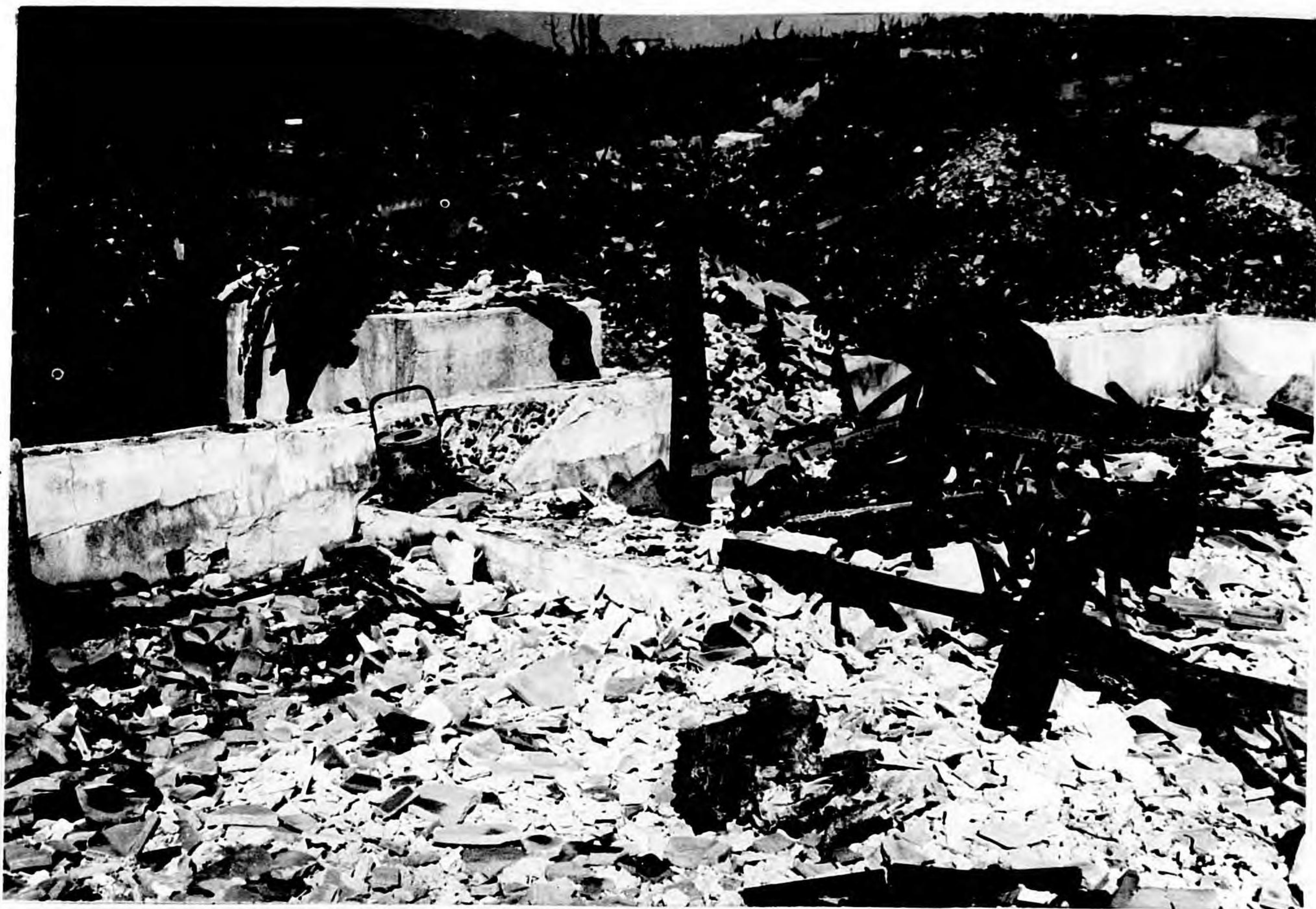
Photo 128. Nagasaki, 2,000 feet from GZ. Electrical system destroyed by fire.
