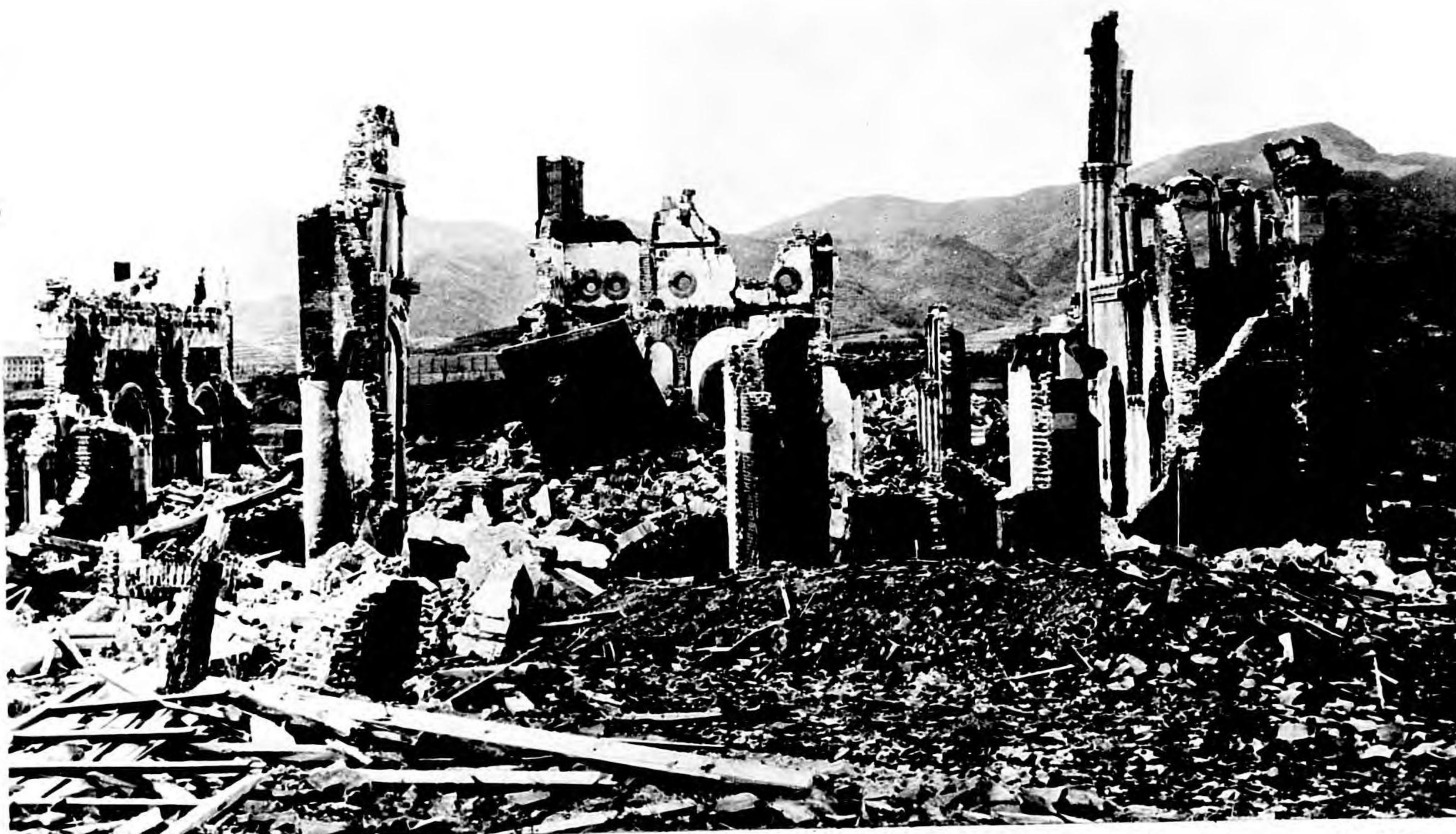
Photo 158. Nagasaki. Urakami cathedral. Brick and stone building, 1,800 feet from GZ, totally damaged by blast. Concrete dome from west tower resting in center of debris.
