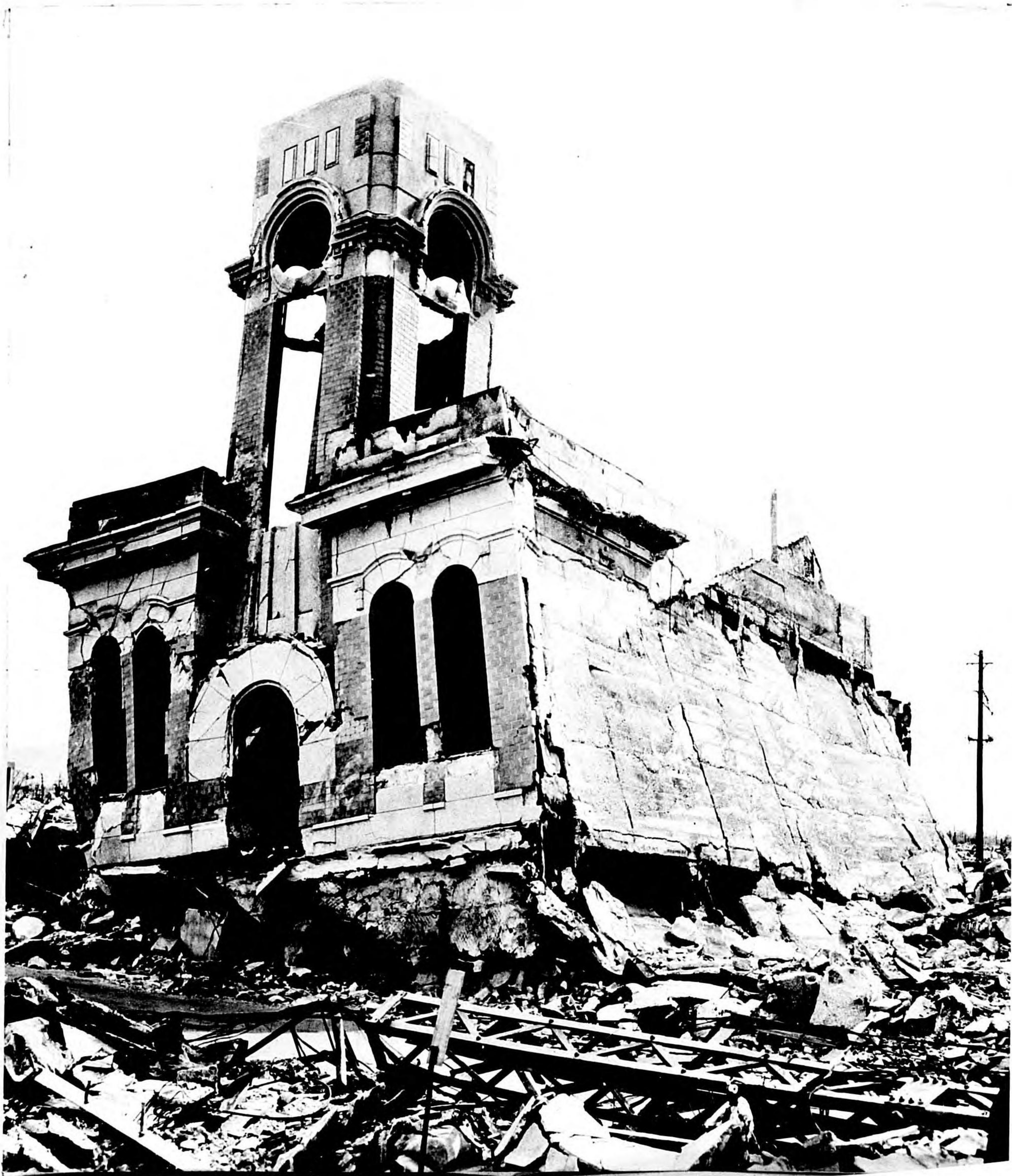
Photo 163. Hiroshima. Shimomura Watch Shop, 2,000 feet from GZ. Second story of steel-frame building resting on ground. Columns and walls of first story at right. Combustible debris burned.
