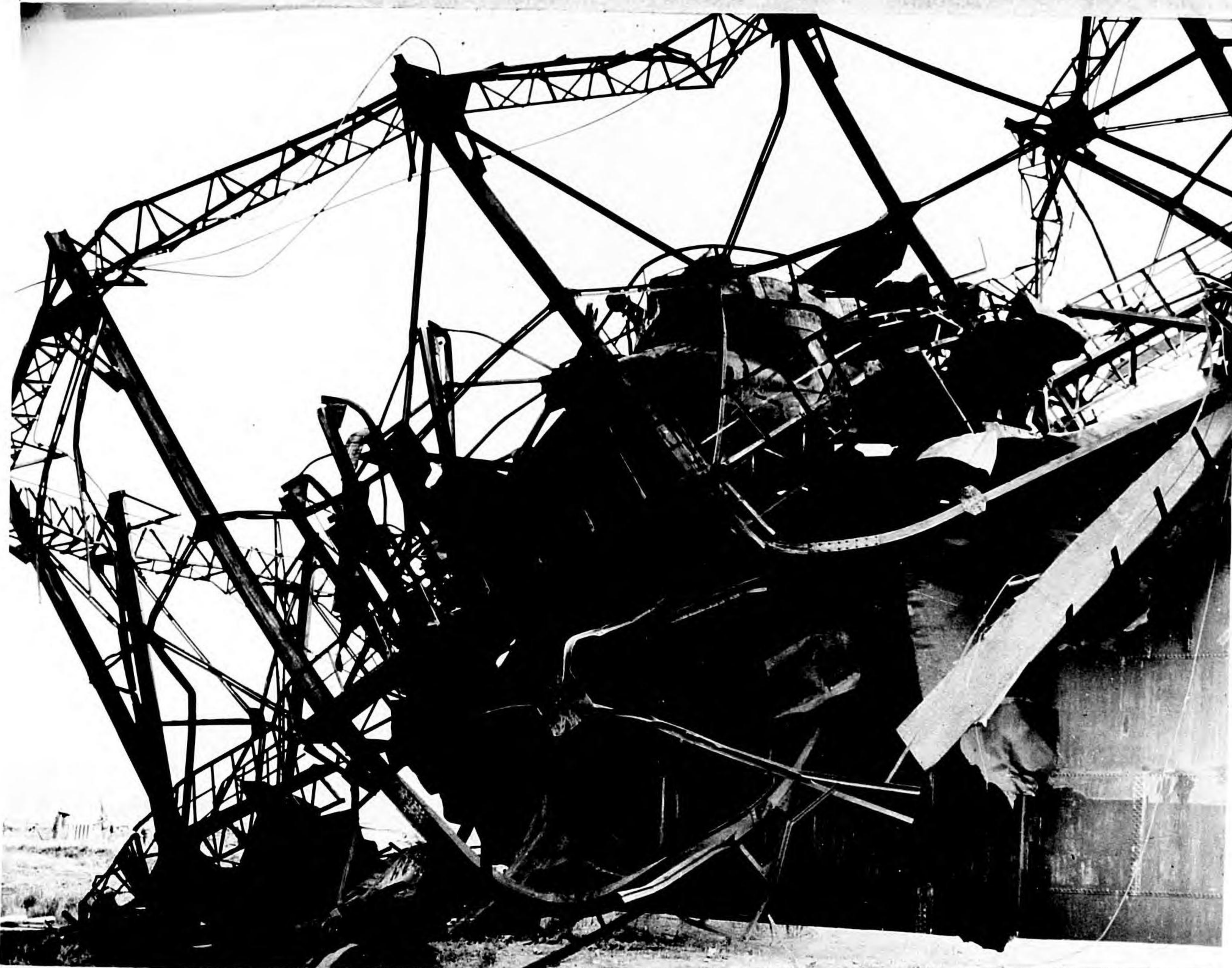
Photo 143. Nagasaki, 3,000 feet from GZ, Ohashi Gas Works. Damaged tank top of gas holder.
