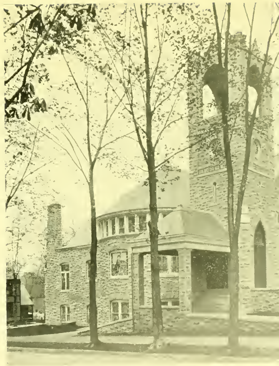
The New England Congregational Church, corner Circular and C.
