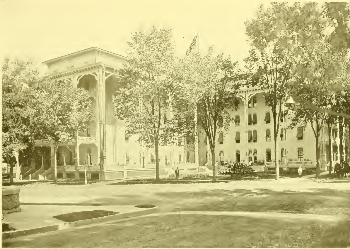
The Kensington Hotel on Union Avenue.
