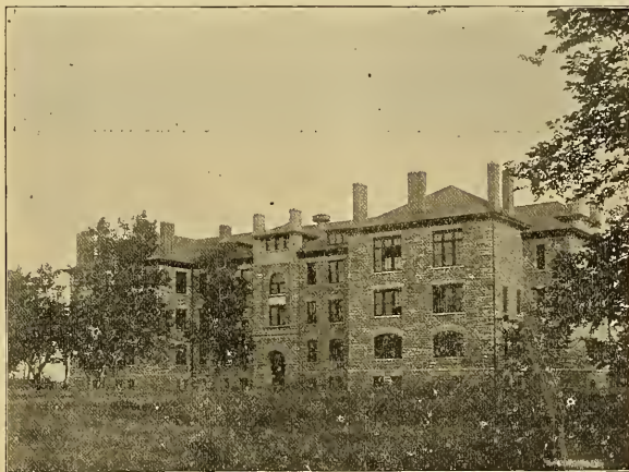
Chemical Laboratories. South Front.
