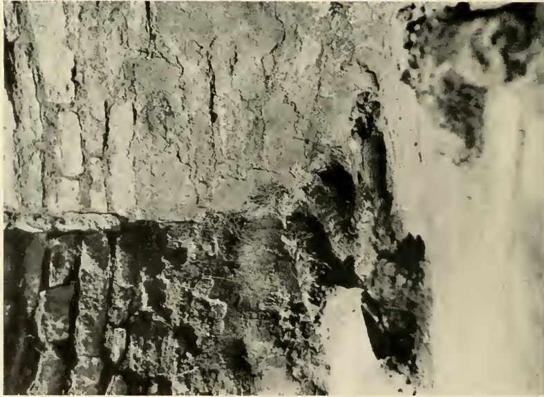
1. Showing charred beams in corner of Kiva KT-II, Kim Tiel.
