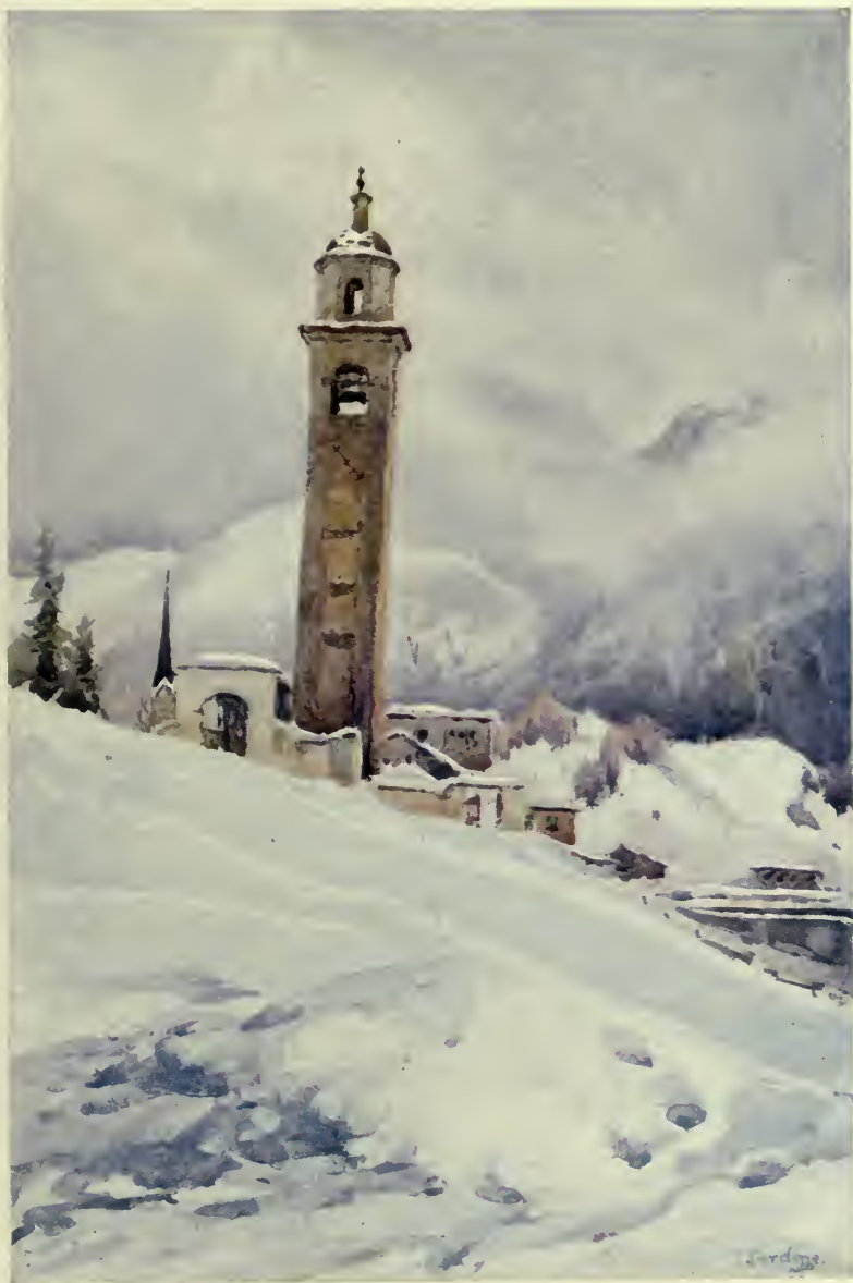
THE LEANING TOWER OF ST. MORITZ "OLD CHURCH."
