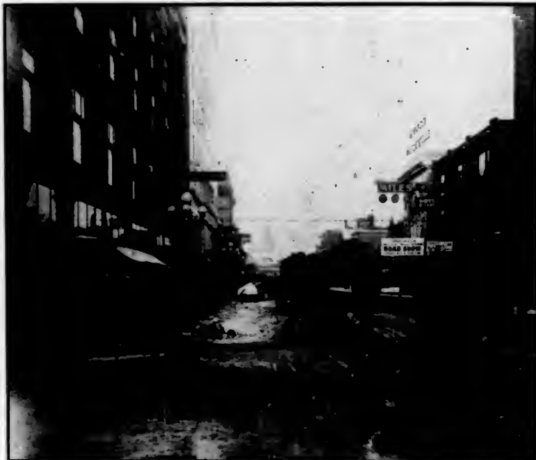
Seventh street looking from Nicollet avenue towards the two theatres.
