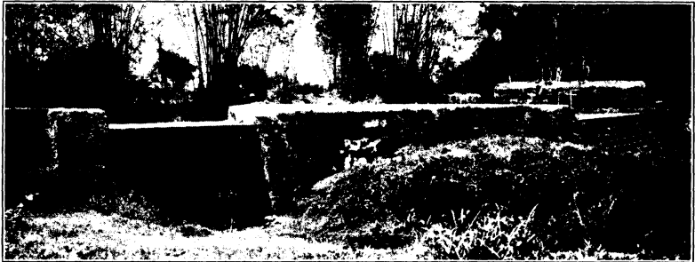
JULIAN DAM, IMUS ESTATE, 2 KILOMETERS SOUTH FROM IMUS, CAVITE DIVISION.
