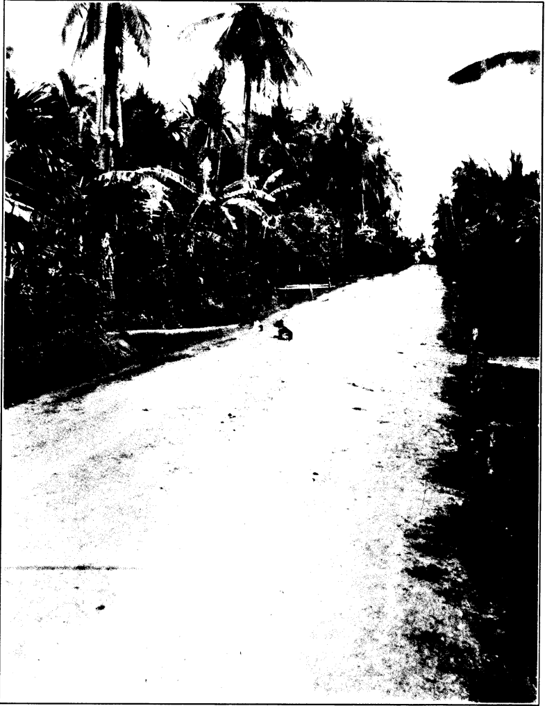
PLATE III.—BAY-SAN PABLO ROAD, LOOKING WEST—KILOMETER 52, LAGUNA.
