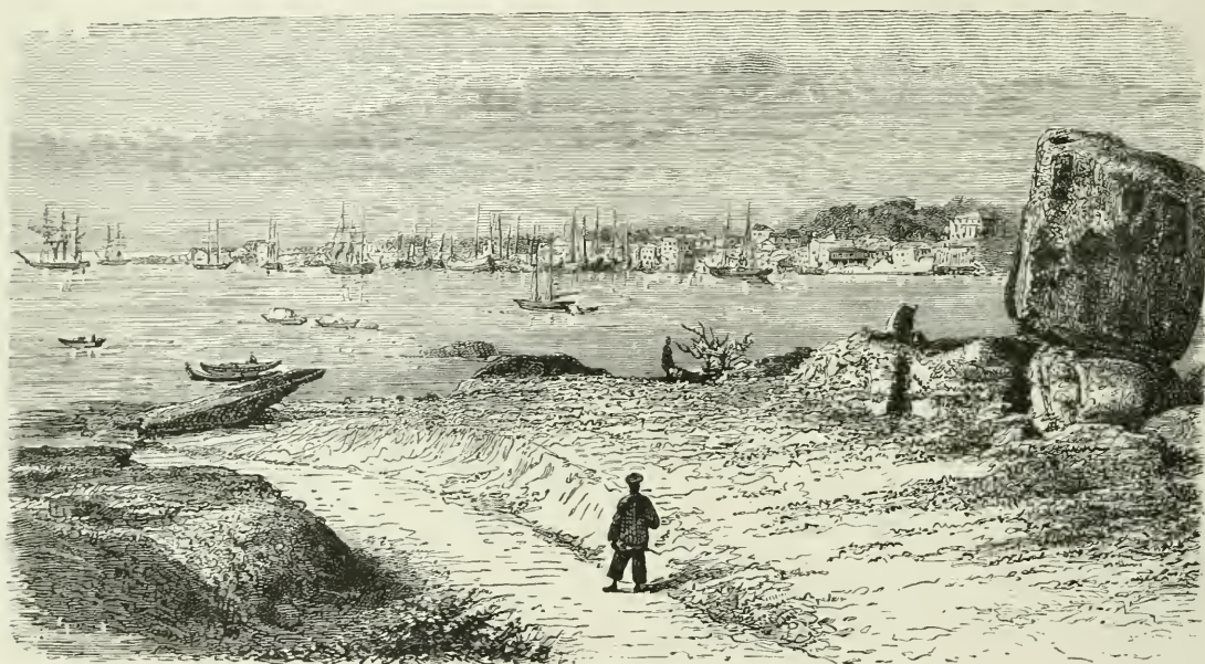
VIEW OF THE CITY OF AMOY, IN THE PROVINCE OF FO-KIEN.
