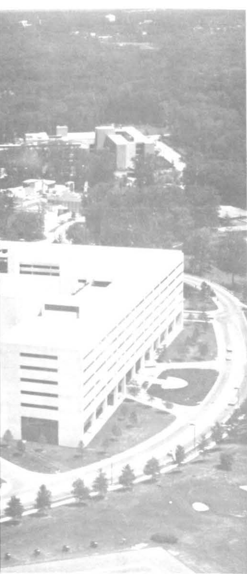
The 500-bed, 881,000-square-foot tertiary care facility at NNMC Bethesda opened in the winter of 1980. The Tower complex is presently being renovated and will be used for hospital support services. Bottom: Branch Dental Clinic at NAS Cecil Field.
