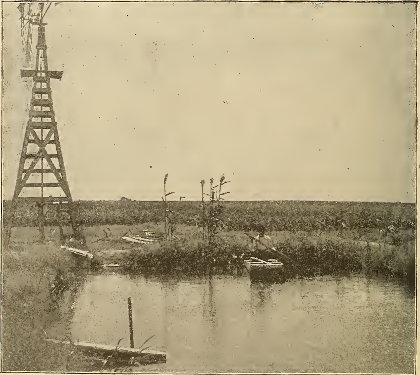
FIG. 2.—Reservoir and windmill pumping water from Dakota sandstone, about 18 miles south of Dodge, Kansas.
