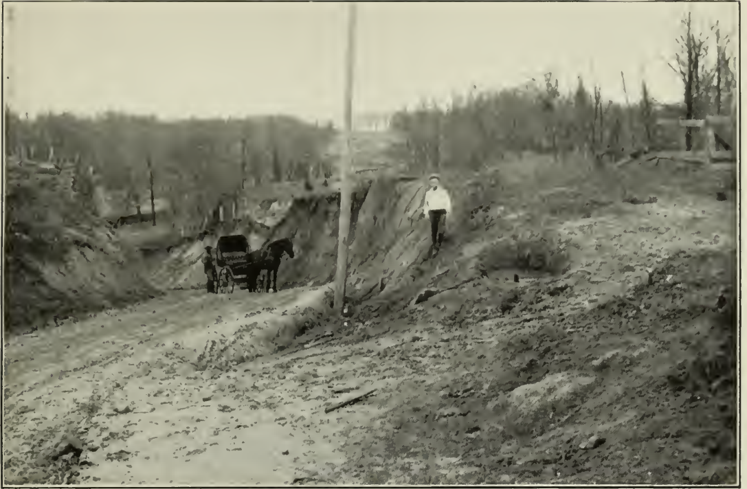
FIG. 1.—THE EVOLUTION OF A COUNTRY ROAD—1. APRIL 15, 1904. [At this point the road was straightened and placed on better ground.]
