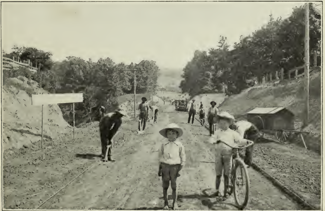
FIG. 2.—THE EVOLUTION OF A COUNTRY ROAD—2. MAY 18, 1904. [Finishing up the grade of the newly opened road.]
