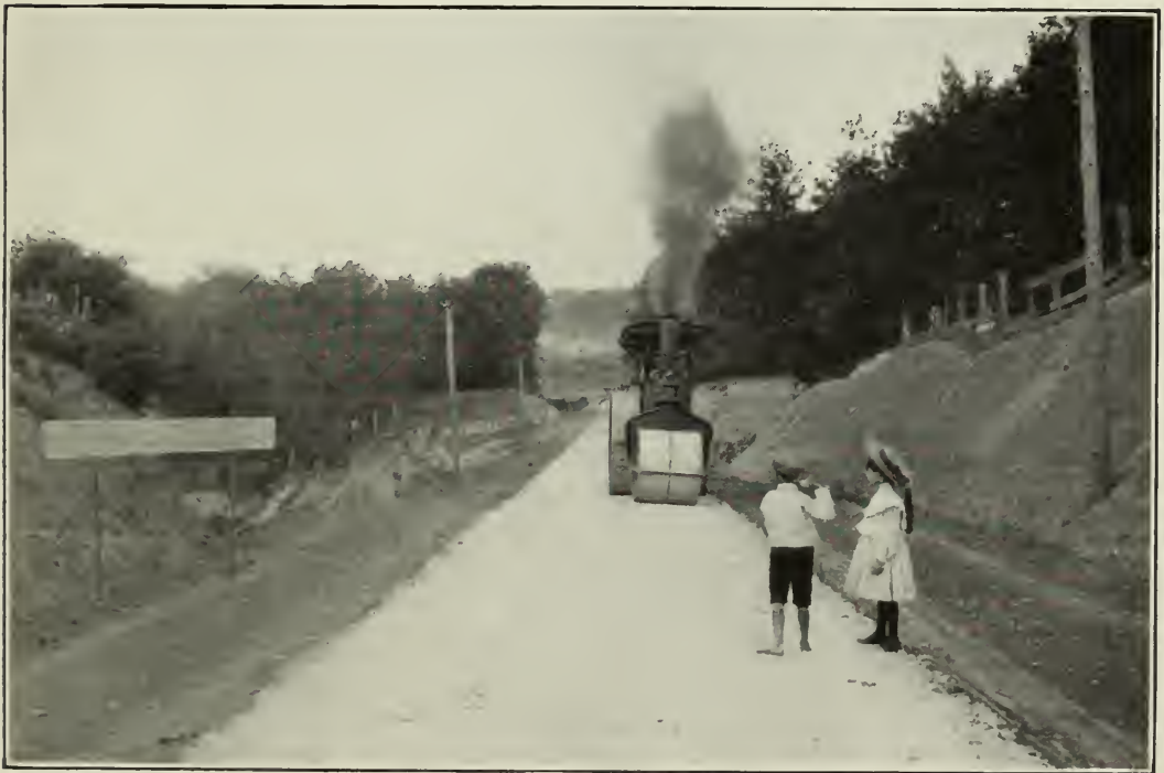
FIG. 2.—THE EVOLUTION OF A COUNTRY ROAD—4. MAY 19, 1904. [First course of stone, 4 inches thick, applied; now being rolled.]
