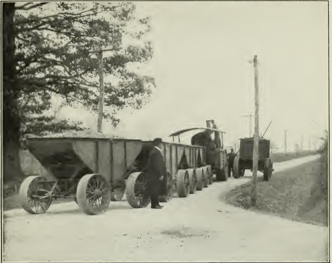
FIG. 1.—HAULING ROAD MATERIAL WITH TRACTION ENGINE. [Four cars, each nolding 5 cubic yards; engine taking water.]
