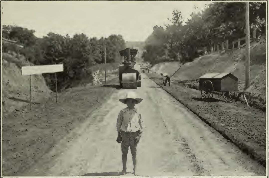
FIG. 1.—THE EVOLUTION OF A COUNTRY ROAD—3. MAY 18, 1904. [Rolling the grade with the 10-ton steam roller.]
