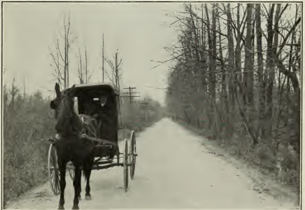
FIG. 2.—CAMPBELLS LEVEE ROAD IN JANUARY, 1905. [Road was improved in 1894; repairs have cost only $33 per mile per annum since.]
