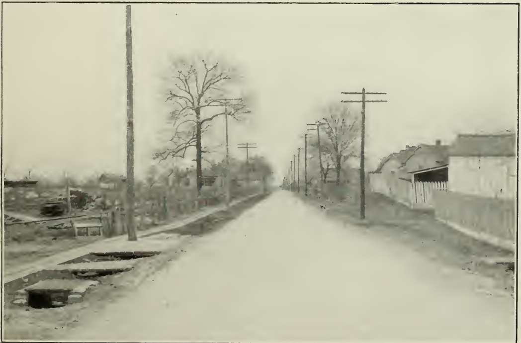
FIG. 2.—POPLAR CORNER ROAD, BUILT JUNE, 1901.
