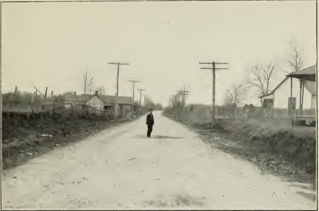
FIG. 1.—POPLAR CORNER ROAD, BUILT JUNE, 1901.
