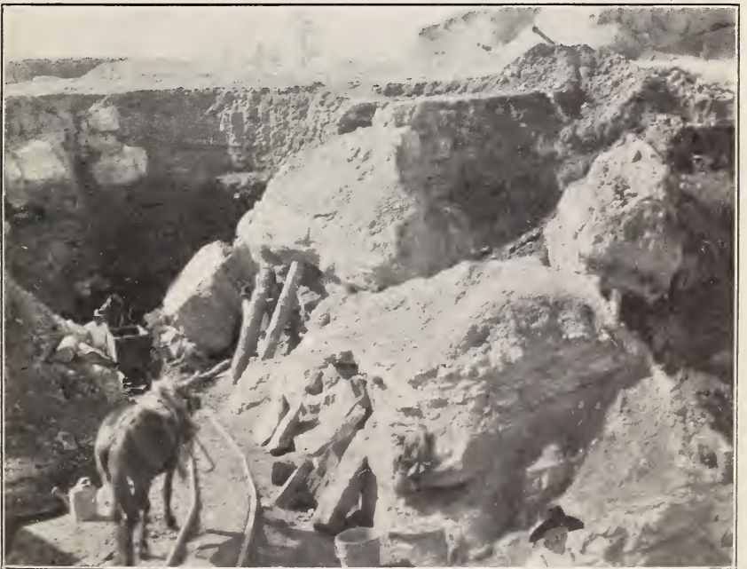
FIG. 2.—BROWN-ROCK MINING, SHOWING BOWLERS OF PHOSPHATIC LIMESTONE.
