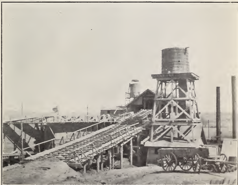
FIG. 2.—BROWN-ROCK PHOSPHATE PLANT, SHOWING HOOD OVER STACK AND SETTLING TANKS FOR FINELY DIVIDED PHOSPHATE.
