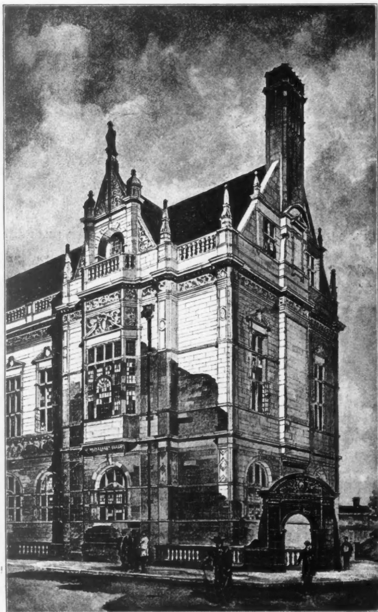
1516. Sheffield Town Hall, south-west angle , EDWARD W. MOUNTFORD, F.R.I.B.A., Architect.
