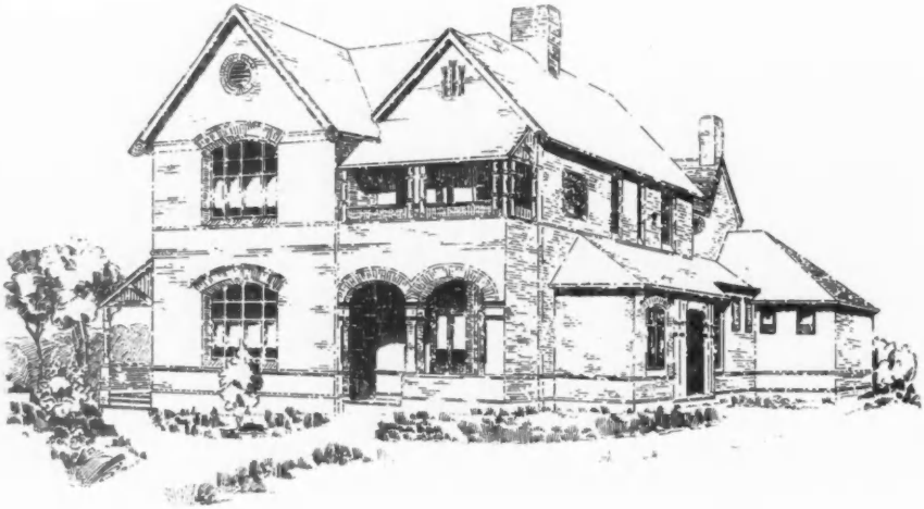
Residence at Potts Point, Sydney, J. B. BARLOW, Architect, Sydney.
