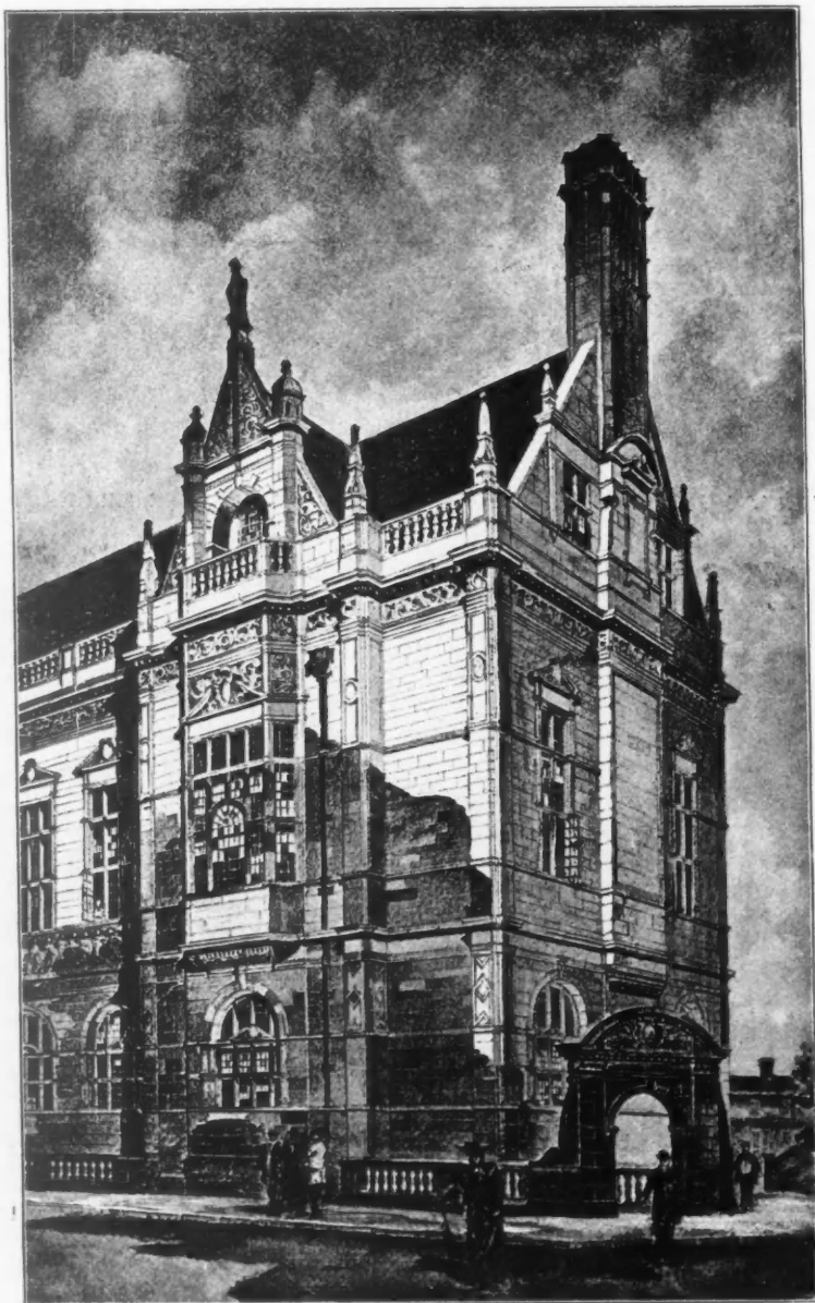
1516. Sheffield Town Hall, south-west angle , EDWARD W. MOUNTFORD, F.R.I.B.A., Architect.
