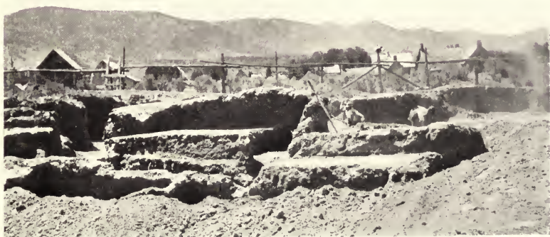
Superposed adobe dwellings, 16-19, with the floors of Rooms 18 and 19 plainly visible. The men are at work in the central court, near Kiva V.
