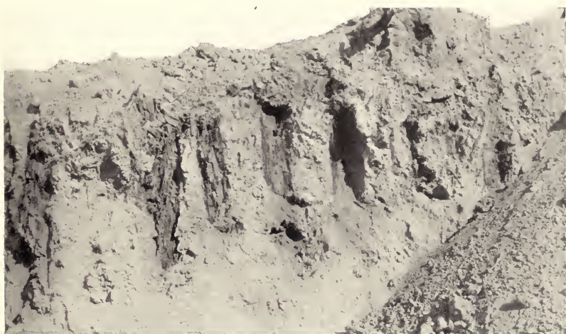
Decayed remains of large upright cedar posts which formed the west wall of Room 43.
