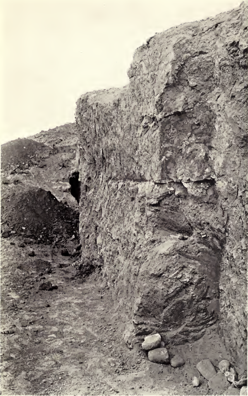
Outer west walls of Rooms 8 and 9, from the southwest. The layer of broken adobe shown in the middle of the photograph rests upon loose earth and débris and forms a foundation for the west wall of Room 9.
