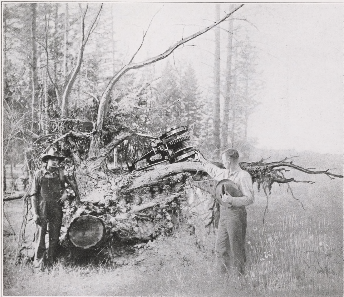
A giant fir, and yet hardly a root broken. The machine perched on the stump gives some idea of the size of the roots pulled out
