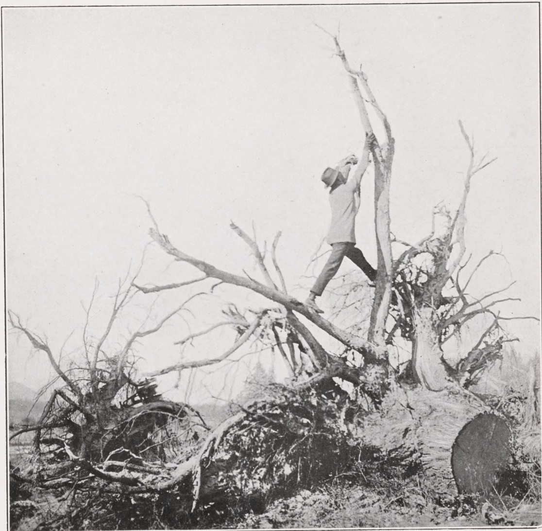
It took twelve minutes to yank this monster out with a 90-ton hitch. Note that the roots were pulled out—not broken off, to later interfere with plowing. Compare the length of the roots with the height of Pete Wilson, standing on the stump
