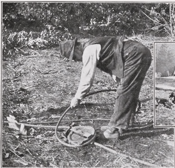
A power pulley (see above) is mighty easy to attach. Take out a pin, insert the cable, and in less than a minute you will be ready for work. There are no latches or springs to come loose and bother you. Each pulley introduced doubles the original power of the machine
