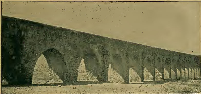
AQUEDUCT AT CHIHUAHUA.
