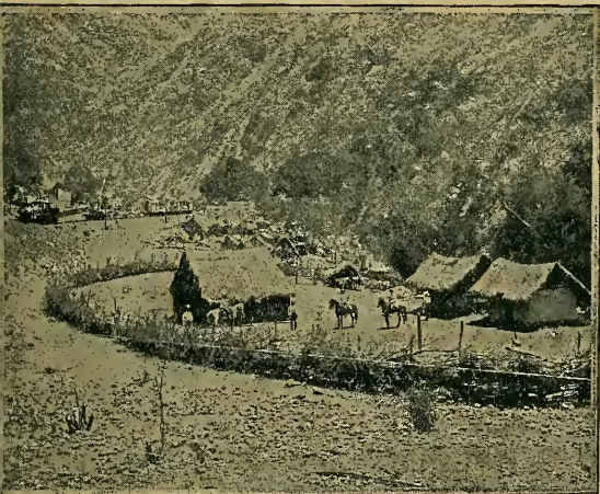
RAILWAY CONSTRUCTION CAMP, MEXICAN SOUTHERN RAILROAD.
