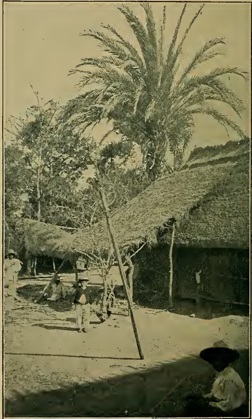
AT CUAUTLA, INTEROCEANIC RAILWAY.
