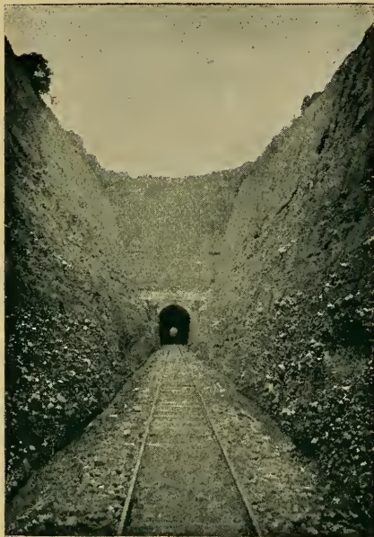
TUNNEL PORFIRIO DIAZ, INTEROCEANIC RAILWAY.
