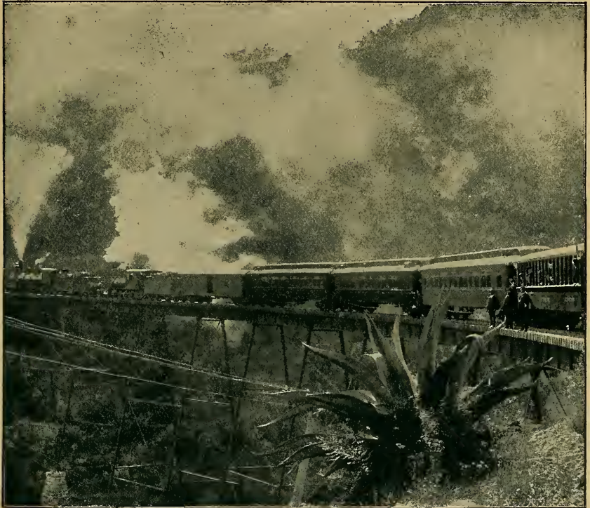
THE CURVED BRIDGE ABOVE DOS RIOS, MEXICAN NATIONAL RAILROAD.
