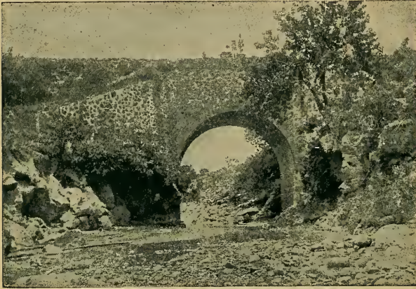
CULVERT NEAR ACAJETE, INTEROCEANIC RAILWAY.
