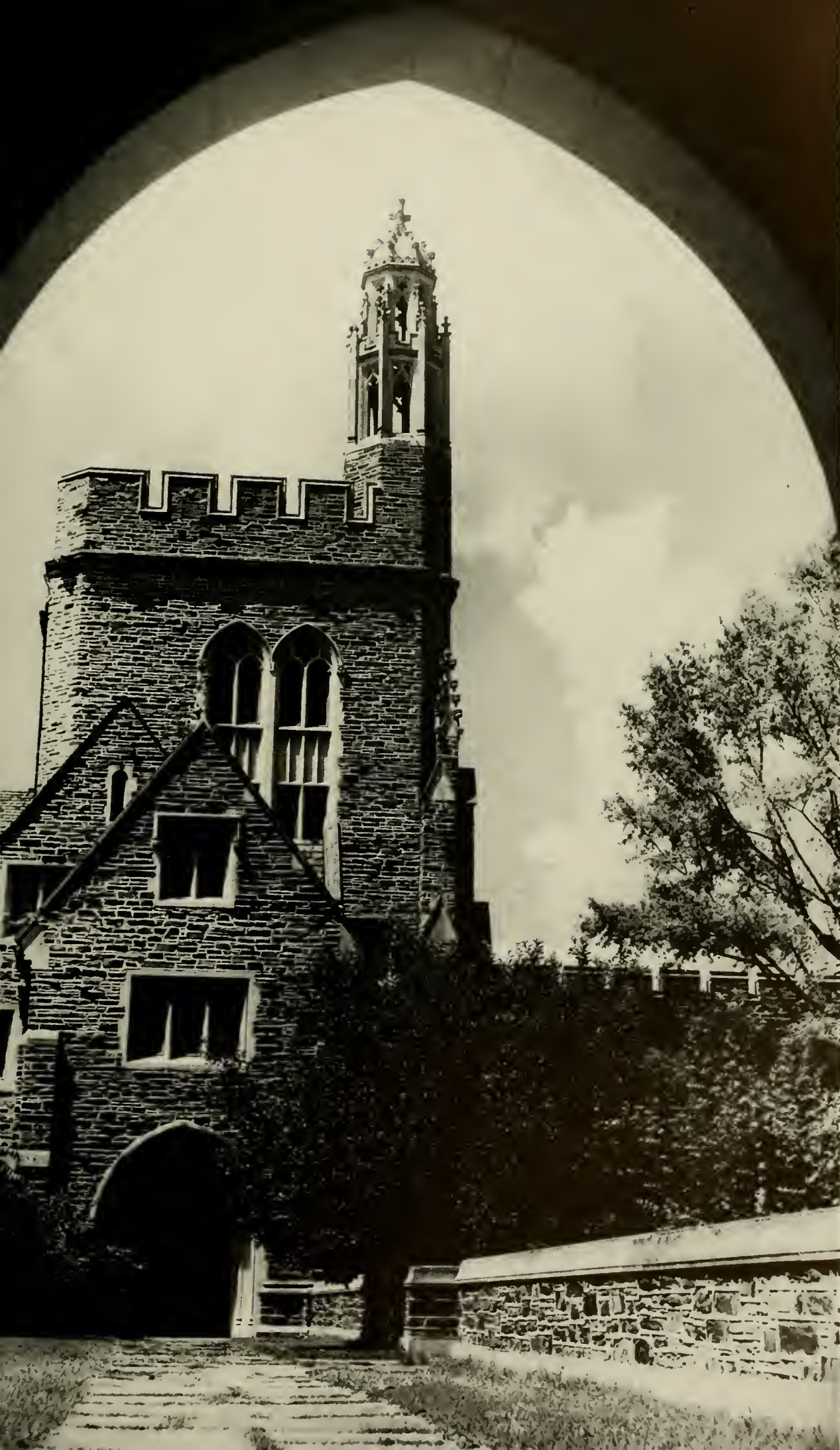
KILCO BELL TOWER—WEST CAMPUS
