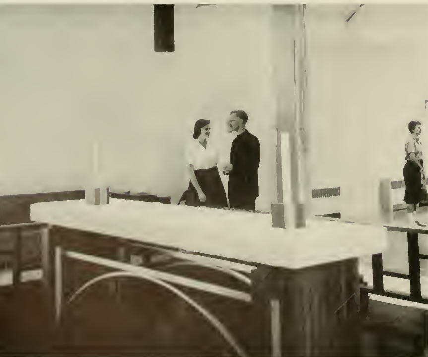
The newly constructed Episcopal Student Center
