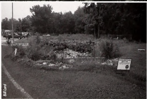
TOP TO BOTTOM: River Bend Mayor John Kirkland and Town Manager Eric Pearson are pleased with their stormwater wetland demonstration. • This stormwater wetland in River Bend directs runoff from U.S. 17 toward water-loving vegetation. • This outlet weir at Smithfield-Selma Senior High School wetland is equipped to measure flow and temperature of water leaving the wetland. • The Smithfield demonstration wetland removes pollutants from runoff, slows discharge of stormwater, and can limit flooding and erosion downstream.
