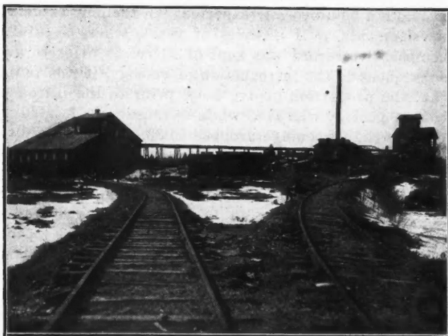
NO. 1 SHAFT AND 100-TON FLOTATION MILL MASSEY COPPER MINE
