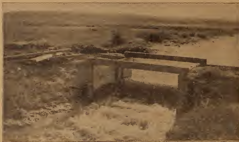
Measuring weir taken where a ditch comes through a dry field, showing the unbroken and unirrigated land as it is in this section
