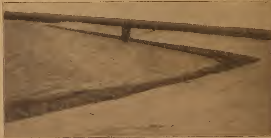
The dike of Clark's Lake of the North Platte Irrigation System, showing riprap of rock and concrete, with headgate for control of water supply
