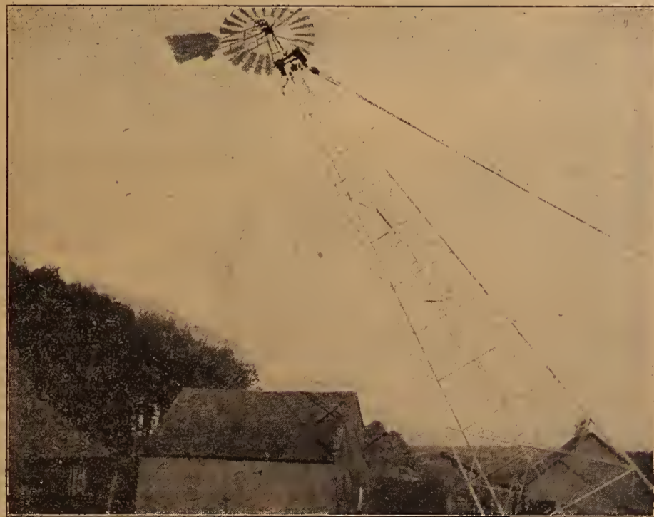
THE STEEL WINDMILL TOWER IS BEING RAISED INTO POSITION
