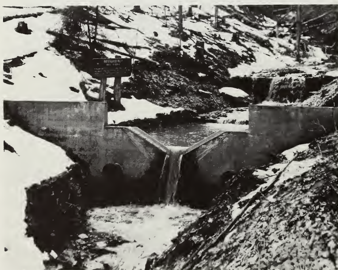
Weir installation to monitor water quality.
