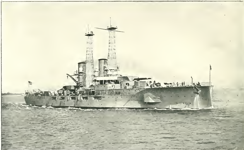
U.S.S. Delaware, Water-tube Boiler, Newport News, Va.
