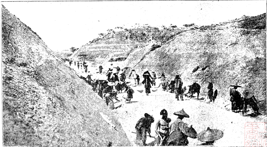
RAILROAD BUILDING IN CHINA: WORKING IN A CUT.—From a photograph of 1904.
