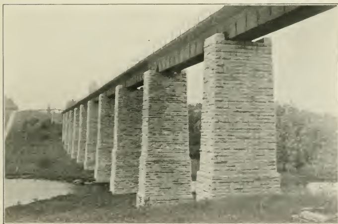
Grand Trunk Railway bridge, St. Marys : piers built of limestone. Perth County.
