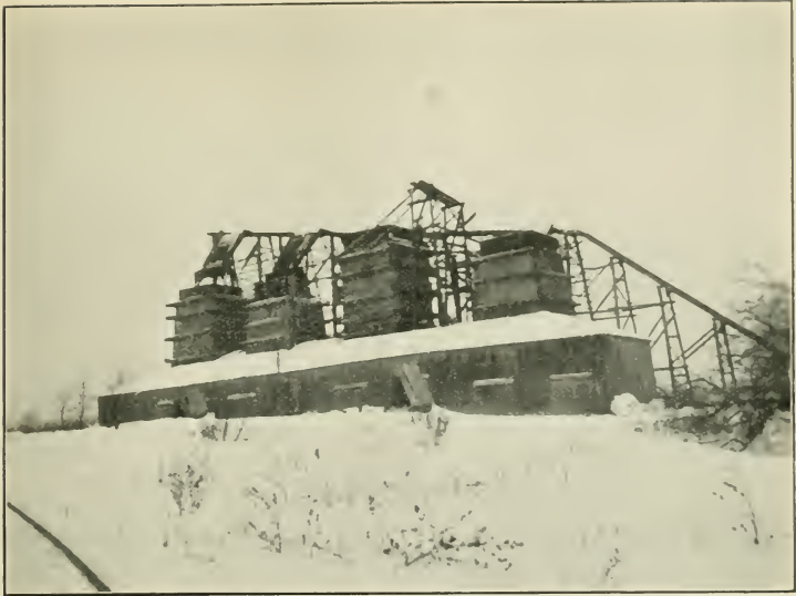
Lime kilns at Sherkston quarry, using natural gas as fuel. Welland County.
