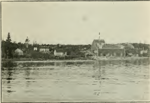
Flint Lake gold mine and mill, 1903.
