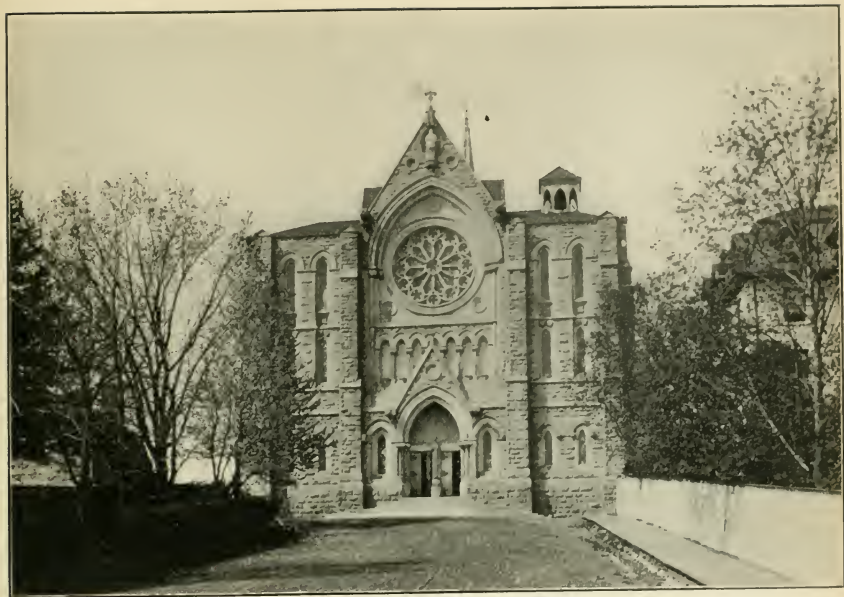
Roman Catholic Cathedral, Guelph; built of limestone from Guelph quarries (Guelph formation).
