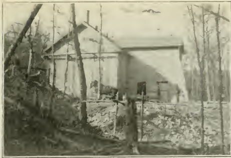
Shaft house, Ranson copper mine.
