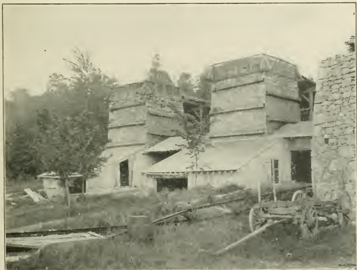
Lime kilns at Dolly Varden siding. Halton County.
