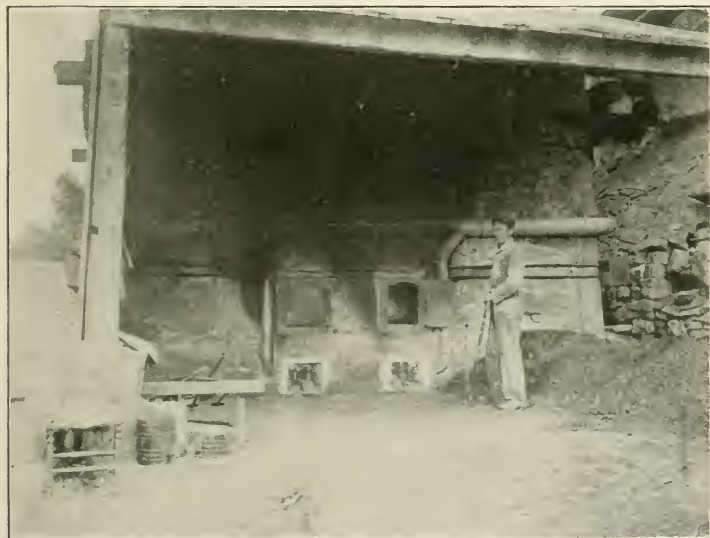
Lime kilns at Limehouse, showing double fire-door and forced-draught pipes. Halton County.
