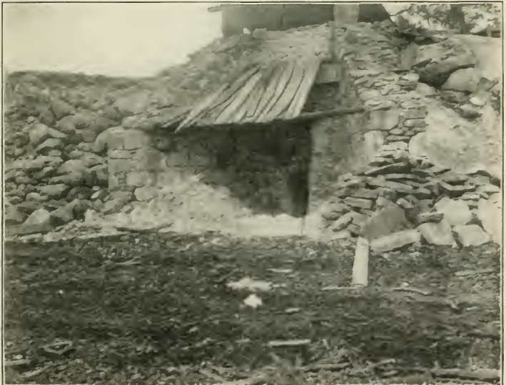
Lime kiln at Galt (Standard White Lime Co.) Old "set" kiln, one of a series of three. Waterloo County.
