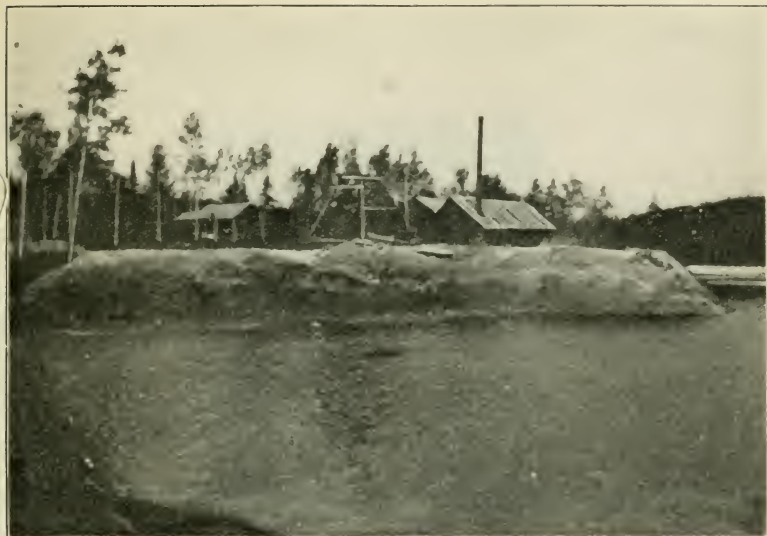
Gold Standard mine : shaft buildings and rock dump.
