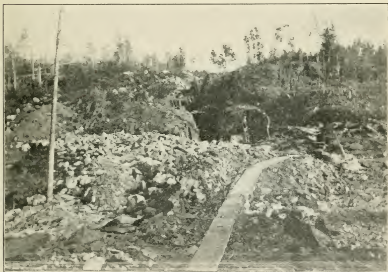
Flint lake gold mine, showing open cut.
