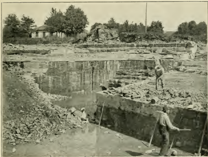
Elliott's limestone quarry, St. Mary's. Product used for building, and waste rock for road metal. Perth County.
