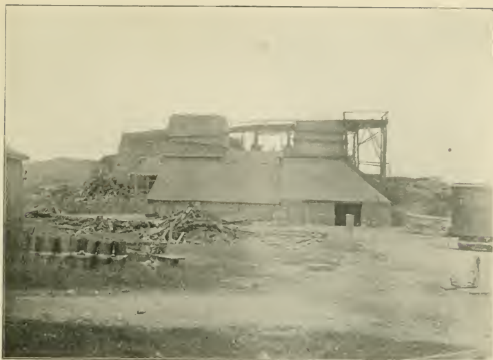
"Kennedy's" kilns, Guelph, (Standard White Lime Co.) Wellington County.
