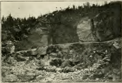
Combined gold mine, showing flat quartz vein overlain by trap.
