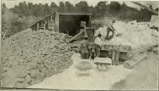
Cobbing ore, Olden zinc mine.
