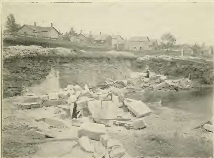
"Kennedy's" quarry, Guelph, (Standard White Lime Co.) Product used for building, and waste rock burned to lime. When taken out, stone is soft and easily worked, but hardens on exposure.
