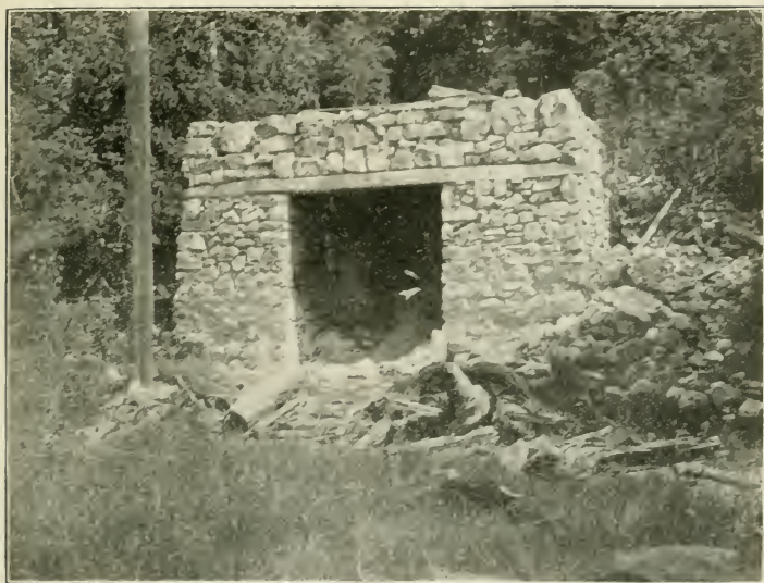
An ancient "set" kiln for burning field boulders; 10 feet high, inside measurement.
