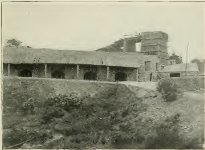
Limehouse: a series of old "set" kilns, with new "draw" kiln on right. Halton County.
