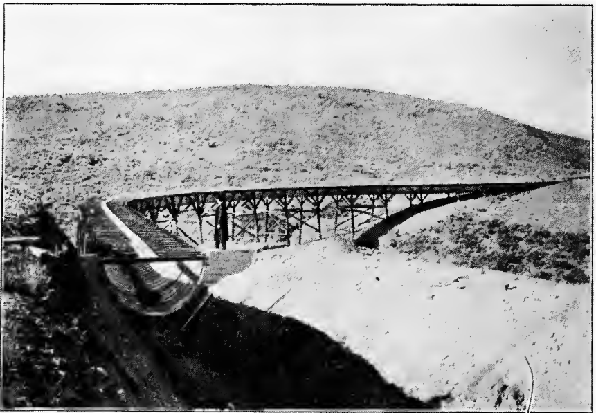
FIG. D.—Metal flume on timber trestle.
