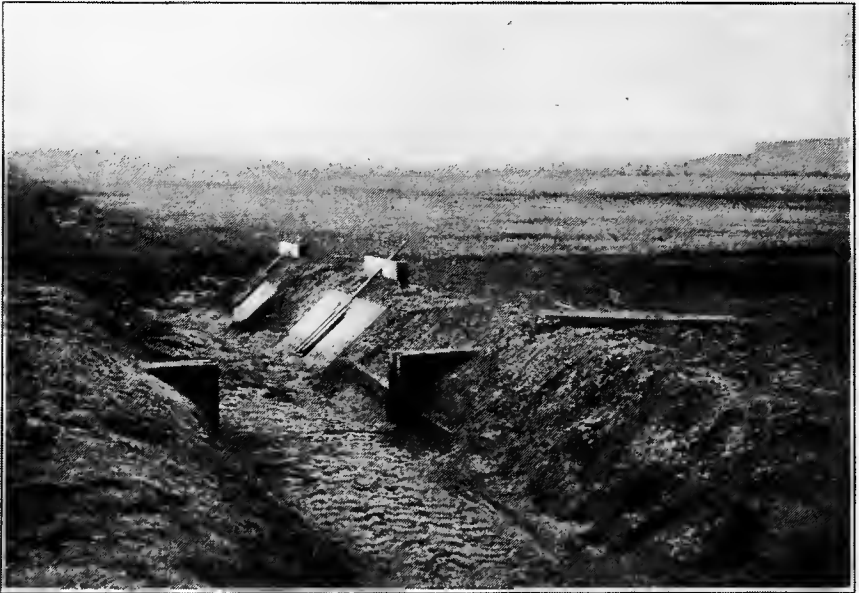
FIG. D.—Farmers' water gates on inclined concrete slabs. Sun River Project, Mont.
