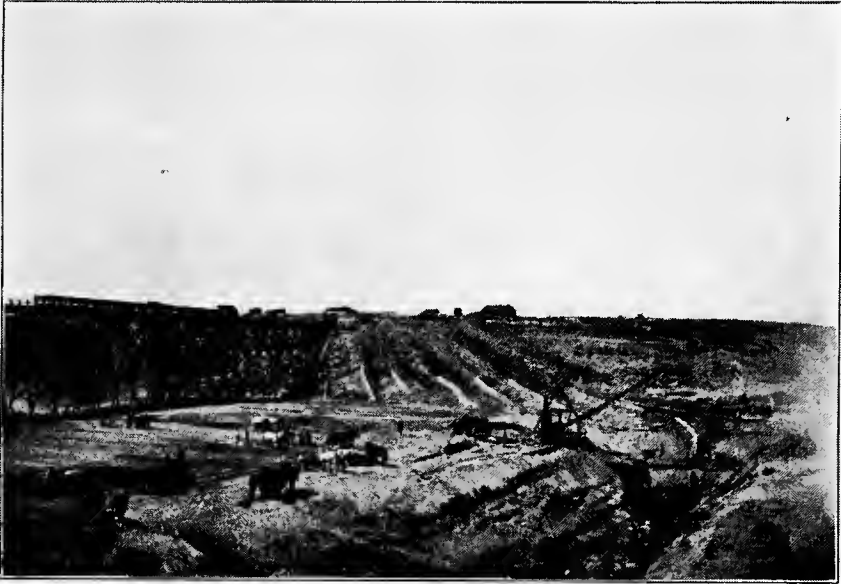
FIG. A.—Foundations for earth dam, showing excavation for puddled core and earth being brought to the site by railroad train, then distributed and rolled in thin layers. Umatilla Project, Ore.
