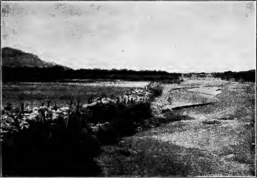
FIG. A.—Brush and stone dam, typical of pioneer conditions. Las Cruces canal, Rio Grande, N. Mex.
