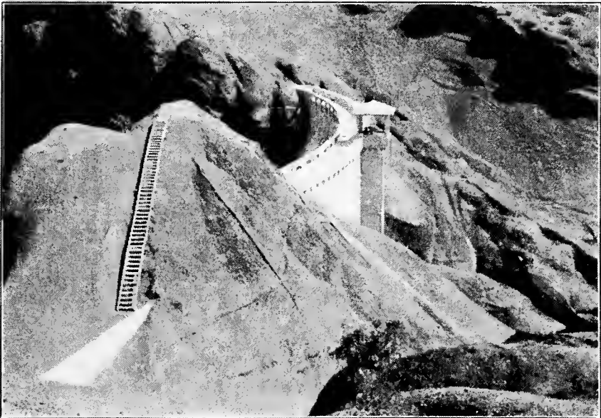
FIG. B.—Concrete structure for regulating floods. East Park dam, Orland Project, Cal.
