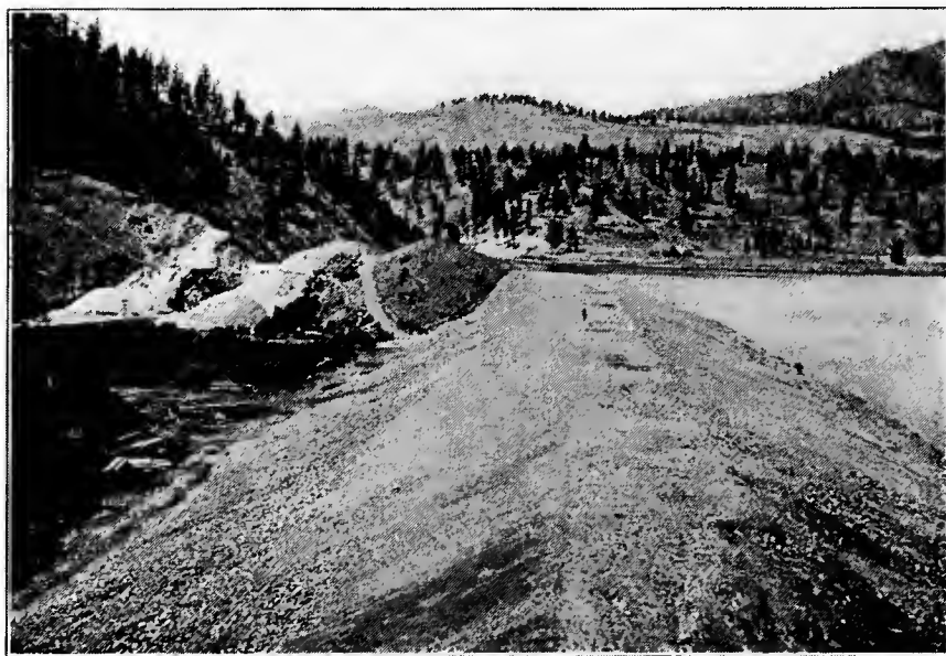
FIG. D.—Completed dam built by hydraulic process, shown above.
