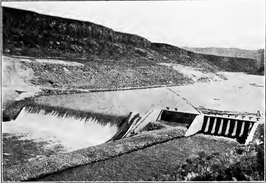
FIG. A.—Diverting dam in Boise River, Idaho, a typical structure for taking out river water by gravity.
