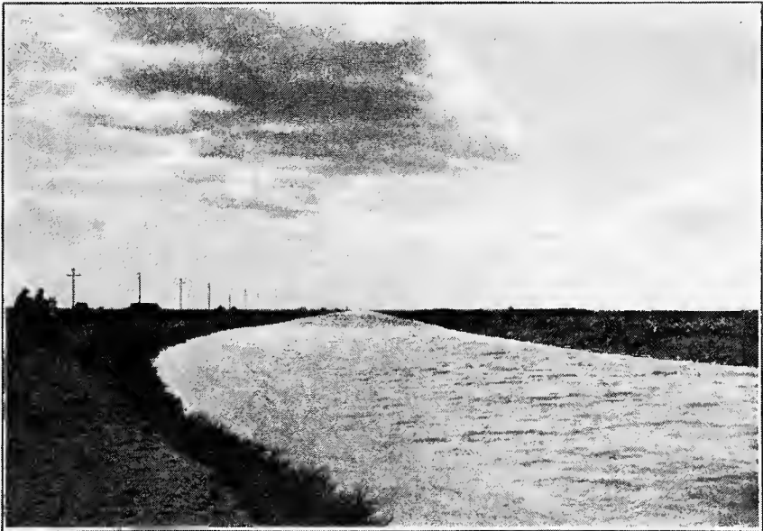
FIG. B.—Main northside canal of Minidoka Project, Idaho. Illustrative of the larger irrigation canals, with power transmission lines located on the bank.
