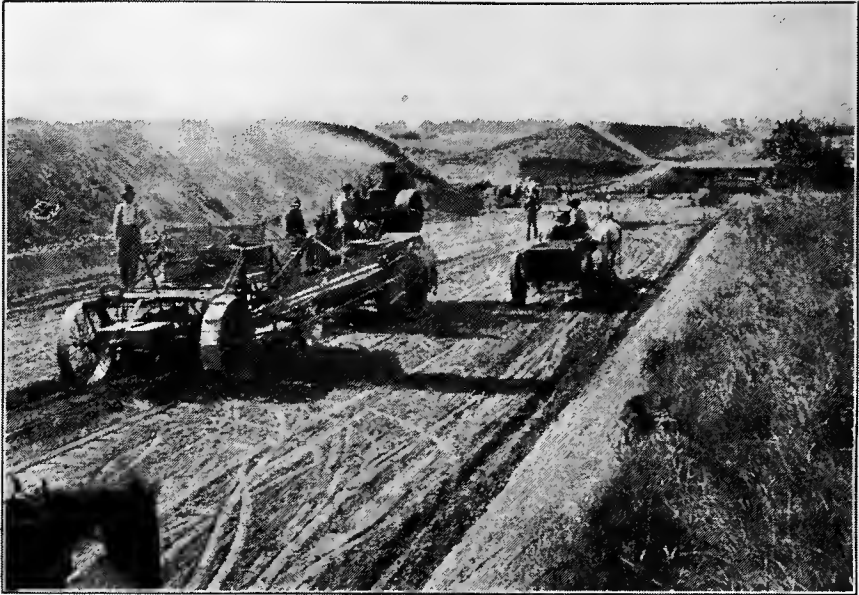
FIG. C.—Excavating canal by use of excavator with belt conveyor, drawn by traction engine. Belle Fourche Project, So. Dak.
