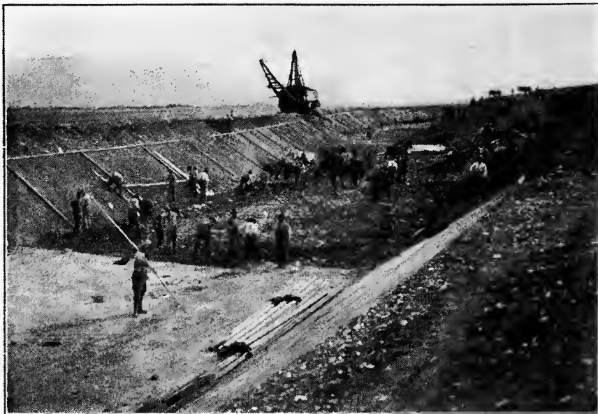
FIG. C.—Lining canal with concrete to increase the capacity, and reduce the seepage. Boise Project, Idaho.
