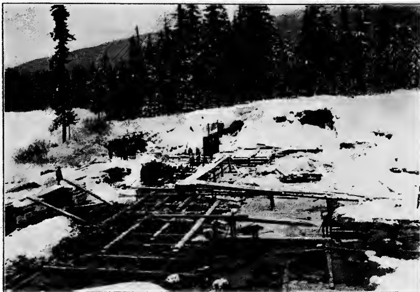
FIG. C.—Foundations for timber dam. Yakima Project, Wash.
