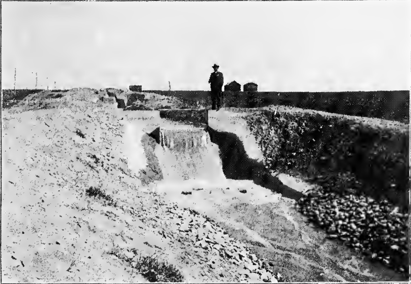
FIG. A.—Series of checks and drops with inclined chutes terminating in water cushion with concrete blocks to break the force of the water. North Platte Project, Nebr.
