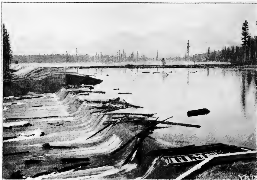
FIG. C.—Spillway of Bumping Lake dam. Yakima Project, Wash.
