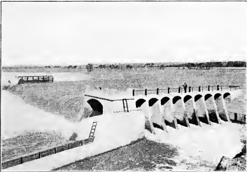
FIG. B.—Concrete headworks with steel gates. Interstate canal, North Platte Project, Nebr.
