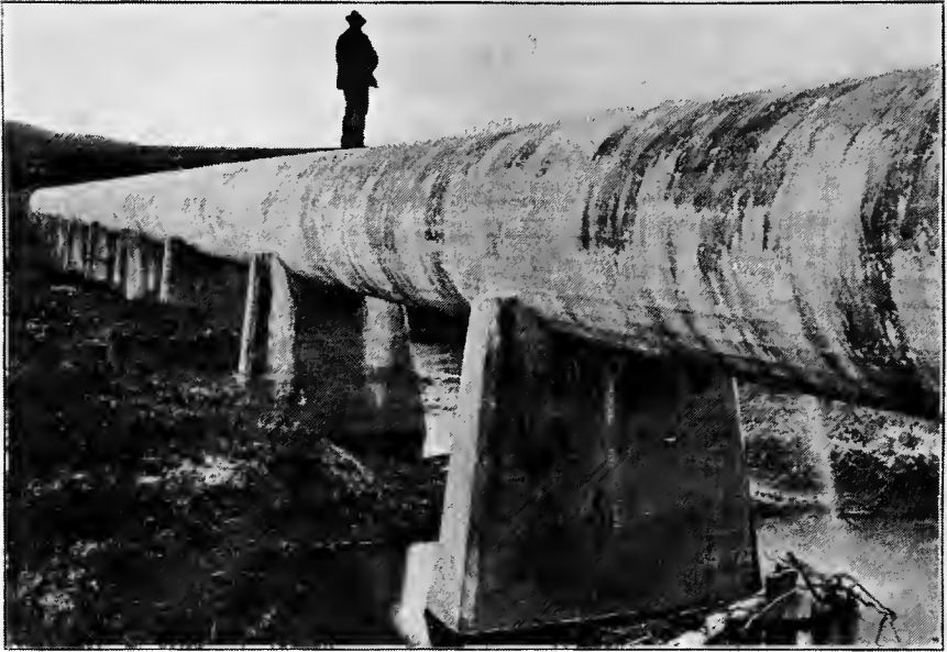
FIG. C.—Concrete pressure pipe used in place of flume. Sun River Project, Mont.
