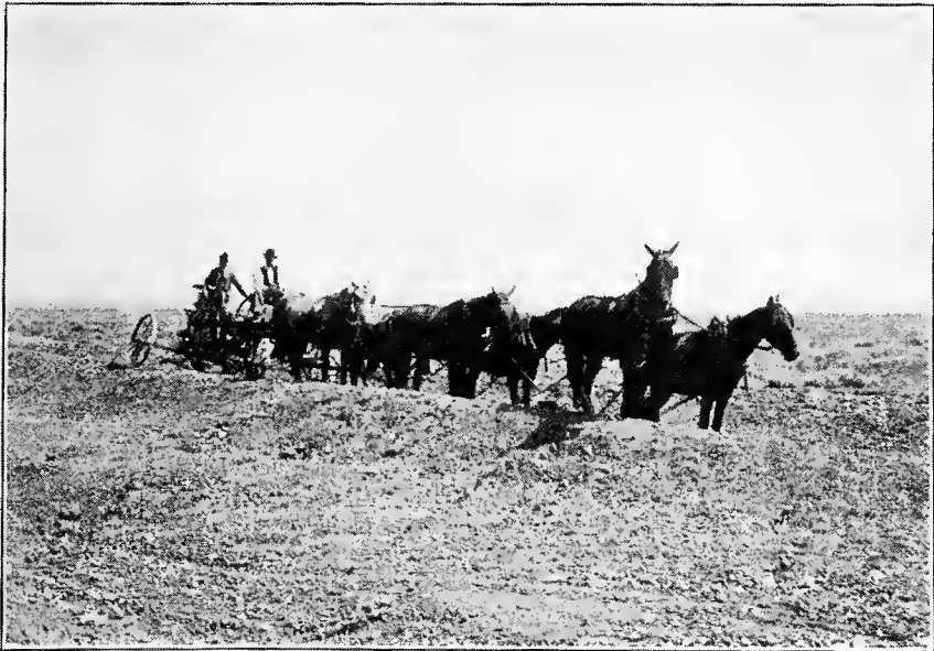
FIG. B.—Throwing up small laterals by means of four-horse road machine. Huntley Project, Mont.
