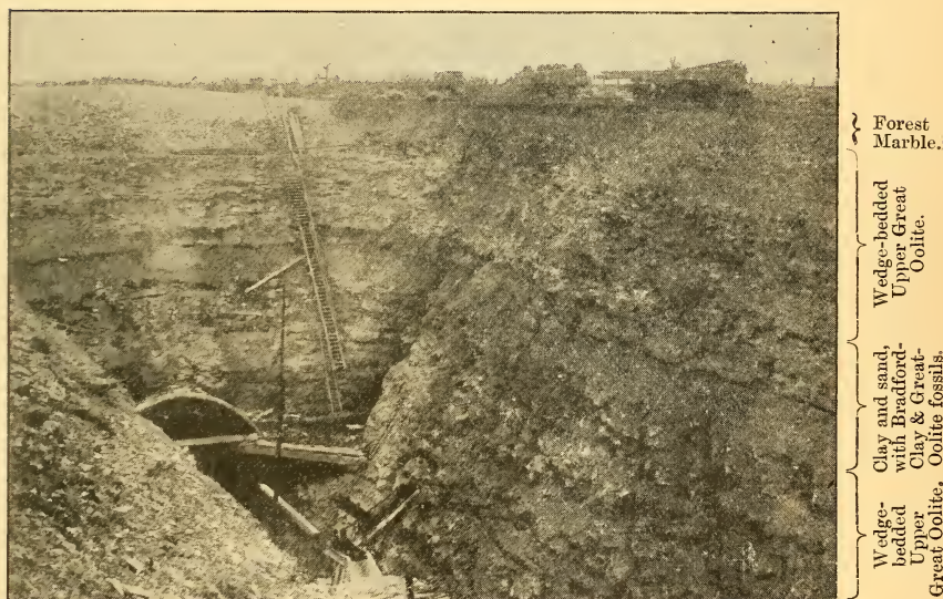
Fig. 4.—The eastern end of Sodbury Tunnel.
