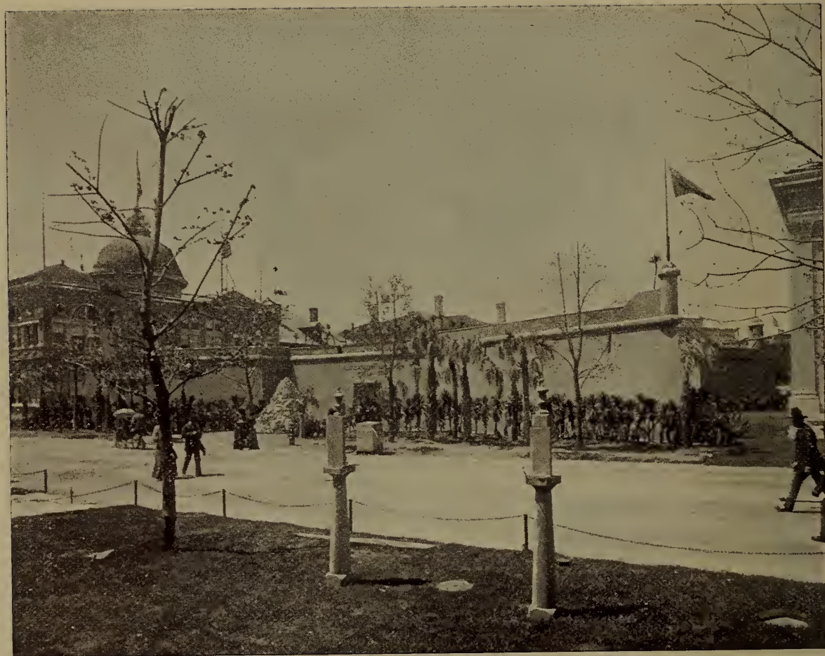
FLORIDA STATE BUILDING.
