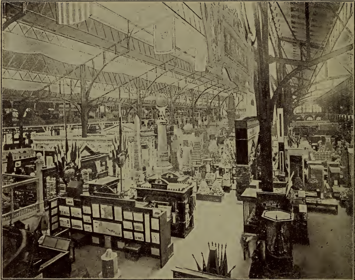
INTERIOR VIEW MINING BUILDING.
