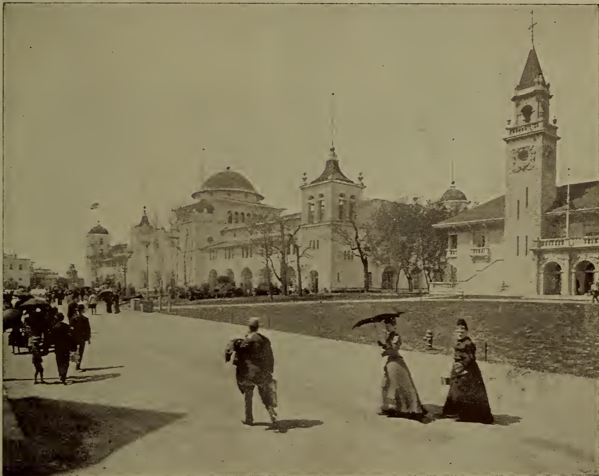
CALIFORNIA STATE BUILDING.
