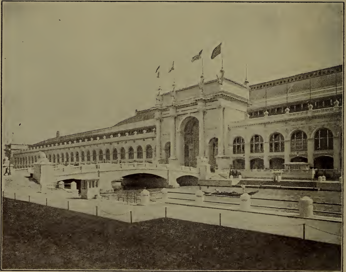
WEST DOORWAY OF MANUFACTURERS' BUILDING.
