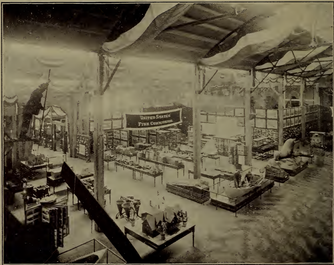
INTERIOR OF FISHERIES BUILDING.
