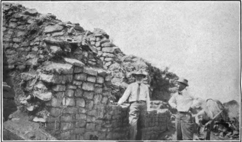
2. MASONRY OF NORTH WALL. PHOTOGRAPH BY MRS. F. W. CHINKSCALES.
