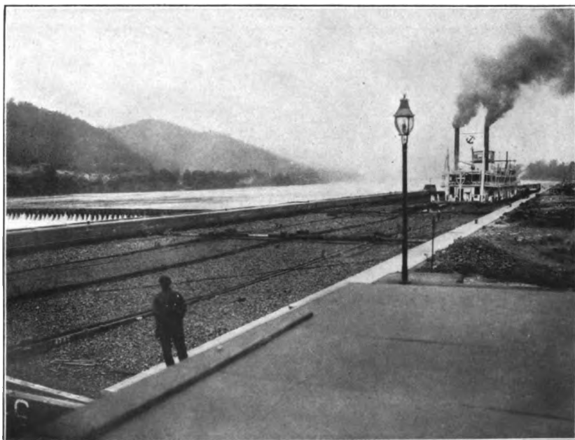
2. A FLEET OF COAL BARGES PASSING LOCK NO. 2, OHIO RIVER. THE MOVABLE DAM IS UP AND IS SHOWN ON THE LEFT.
