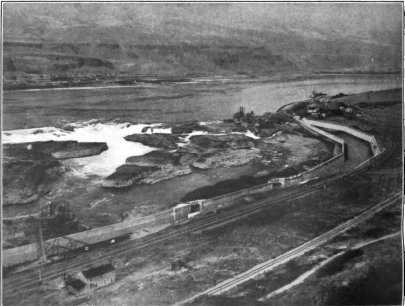
2. THE UPPER END OF THE DALLES-CELILO CANAL, COLUMBIA RIVER, OREG. SIDE WALLS OF CONCRETE CARRY THE CANAL TRUNK AROUND CELILO FALLS.
