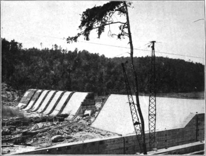
1. DAM NO. 17, BLACK WARRIOR RIVER, ALA., UNDER CONSTRUCTION. THIS DAM HAS A 63-FOOT LIFT, AND IS BEING BUILT BY PRIVATE ENTERPRISE FOR THE CREATION OF ELECTRIC POWER. LOOKING TOWARD THE ABUTMENT END FROM THE LOCK SIDE.
