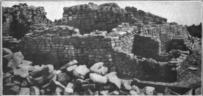
3. NORTHWEST ANGLE, COMPLETELY EXCAVATED. PHOTOGRAPH BY J. WIRSULA.
