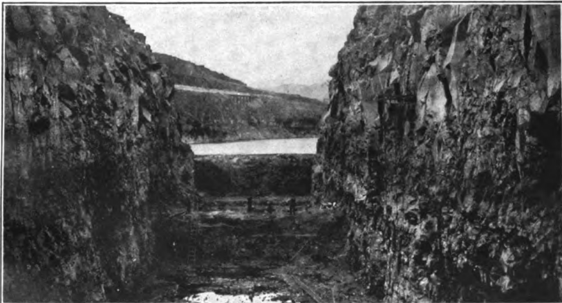
2. EXCAVATION FOR A LOCK IN THE BASALTIC ROCK FOR THE DALLES-CELILO CANAL, COLUMBIA RIVER, OREG.
