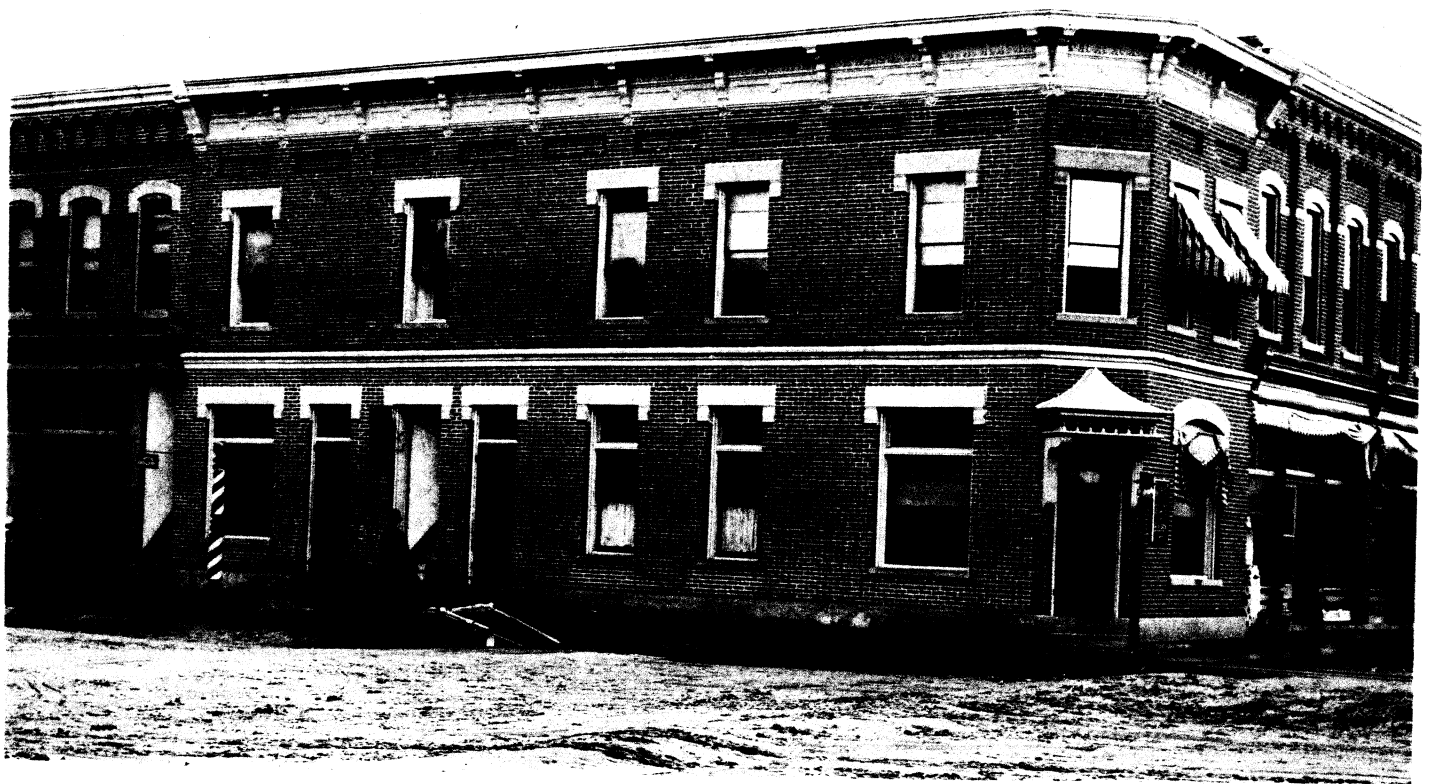
BLISSFIELD STATE BANK BLOCK.
