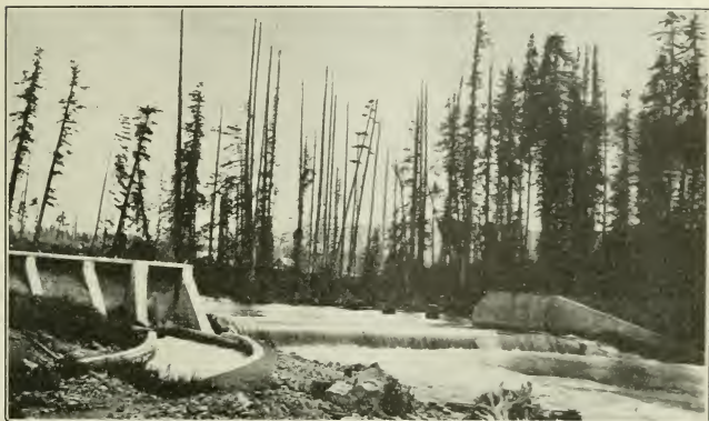
Diversion dam showing flume to intake, of Puntledge River Hydro-Electric Installation on Puntledge river about two miles below impounding dam.
