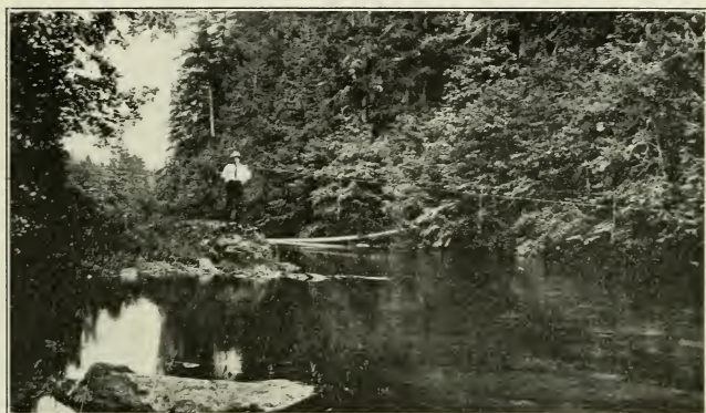
Metering Section on Sproat river near outlet from Sproat lake.
