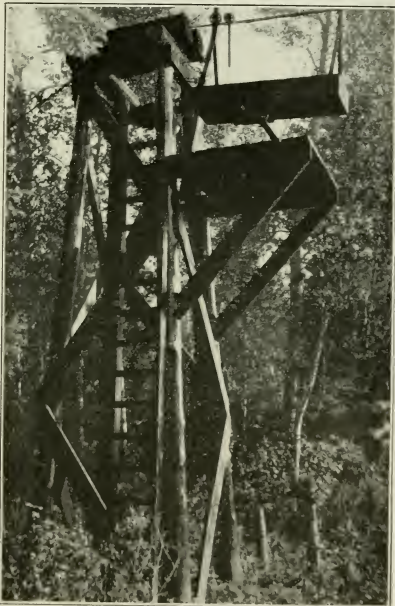
Cranbrook District (H)—Photograph showing support for cable way and platform attachment for cable car.
