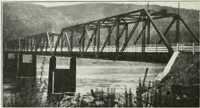
Nelson District (I)—Highway Bridge on Columbia river near Trail, showing metering section on upstream side of bridge.
