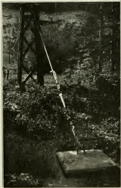
Cranbrook District (1)—Photograph showing Elk river cable station above Canyon.
