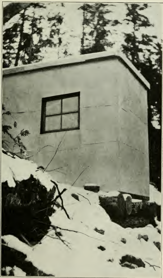
Adams River—Automatic Gauge House.
